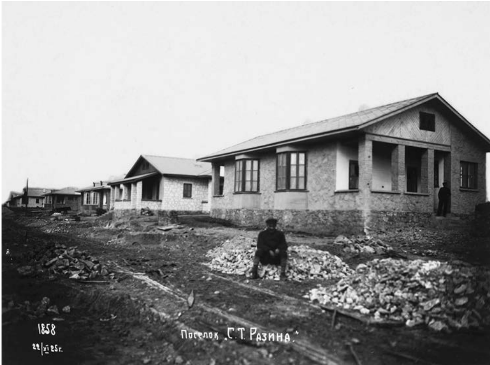
Figure 2.13. Type II (background) and Type III (foreground) houses, Azneft Stepan Razin settlement, Baku, Azerbaijan, November 22, 1925. Architects: Aleksandr Ivanitskii, Viktor Vesnin, Leonid Vesnin, et al. Canadian Centre for Architecture, PH1998:0011:015. Gift of Howard Schickler and David Lafaille.
