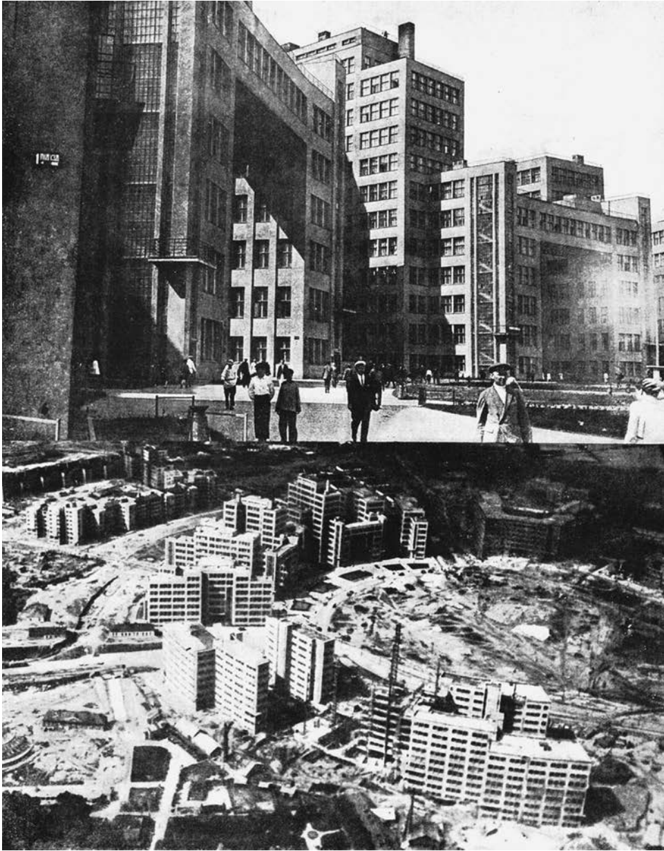
Figure 7.2. Derzhprom building, perspective (top) and aerial view (bottom). Kharkiv, Ukraine, c. 1929. Architects: S. Serafimov, S. Kravets, and M. Felger. El Lissitzky, SSSR stroit sotsializm (Moscow: IZO-GIZ, 1933), 267. © 2020 Artists Rights Society (ARS), New York.
