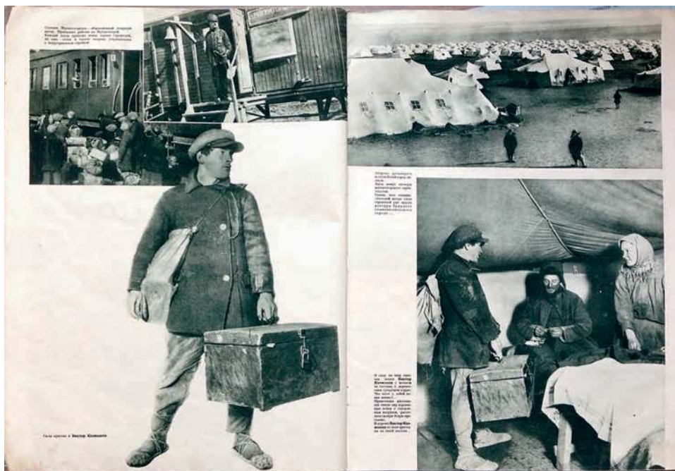
Plate 24. Magnitogorsk issue, with Viktor Kalmykov, “young rural fellow” ( molodoi derevenskii paren' ), arriving to work on the factory's construction. USSR in Construction , no. 1 (1932). Magnitogorskii kraevedcheskii muzei.
