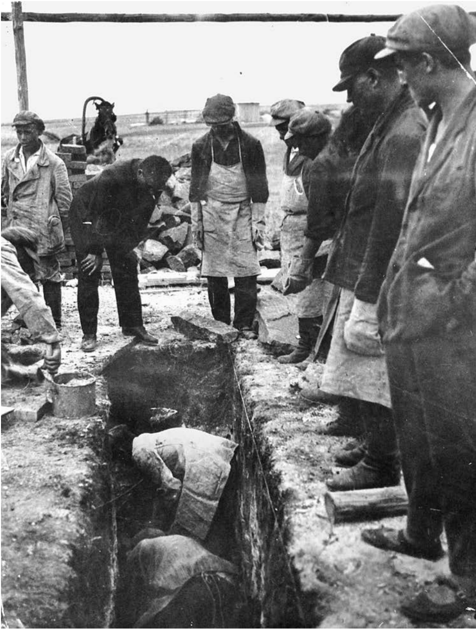
Figure 6.3. Laying the first housing foundation, Pionerskaia Street, Magnitogorsk, Russia, summer 1930. Magnitogorskii kraevedcheskii muzei.
