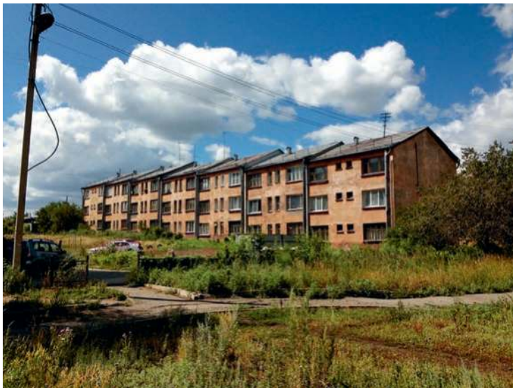
Plate 16. Kirov District “sectional housing,” Magnitogorsk, Russia, 1931–34. Architects: Standartgorproekt / Ernst May Brigade. Photo by the author, 2013.
