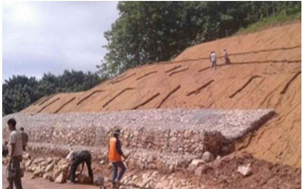
Fig. 7 Landslide mitigation, Lao PDR
