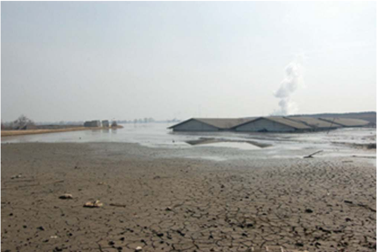
Fig. 12 Damage to houses in the muddy flood (BPLS 2007)
