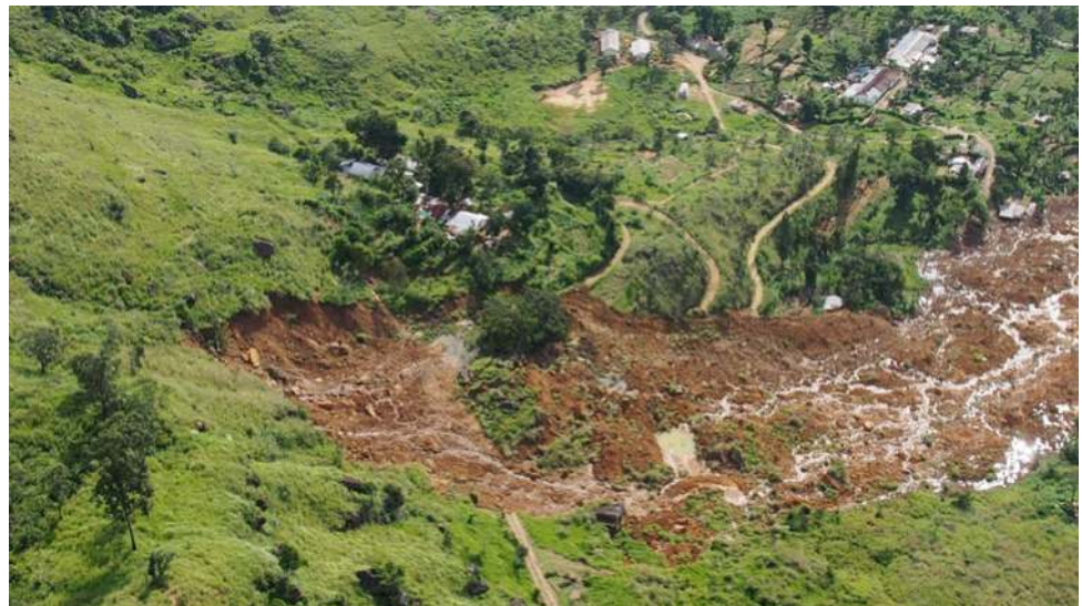
Fig. 1 Meeriyabedda landslide, Sri Lanka ( image source National Building Research Organization, Sri Lanka)
