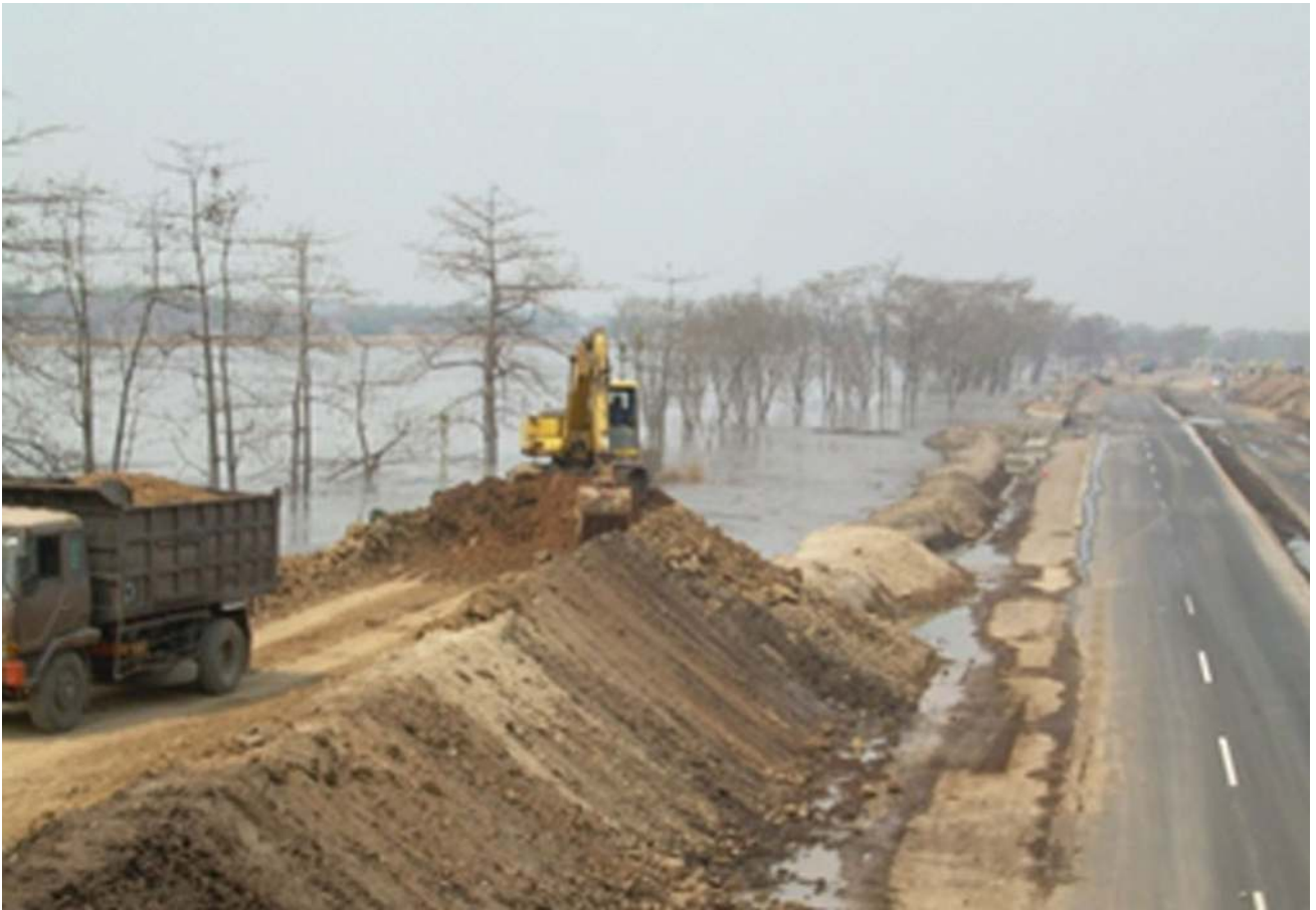
Fig. 21 Construction of permanent dykes (BPLS 2007)
