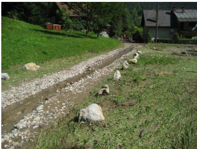
Fig. 7 The consequences of flooding it’s clearly visible; the torrent diverted from original channel and took the forest road as its riverbed (Kambič 2009)
