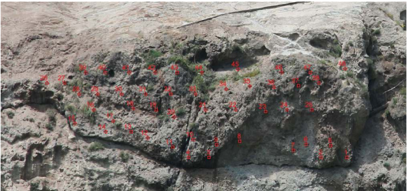
Fig. 31 Positioning of the the 48 installed dowels
