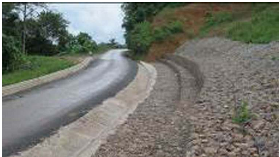
Fig. 5 Resilient landslide protection measures in Bountai District (Lao PDR) provided communities with safer access to public services
