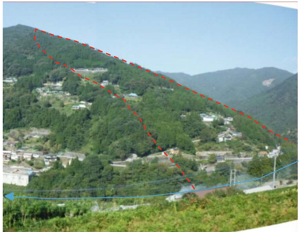
Fig. 8 Overall view of landslide No. 25
