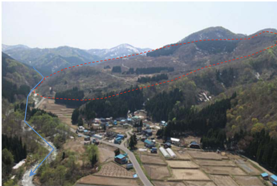
Fig. 5 Full view of the Tozawa landslide site
