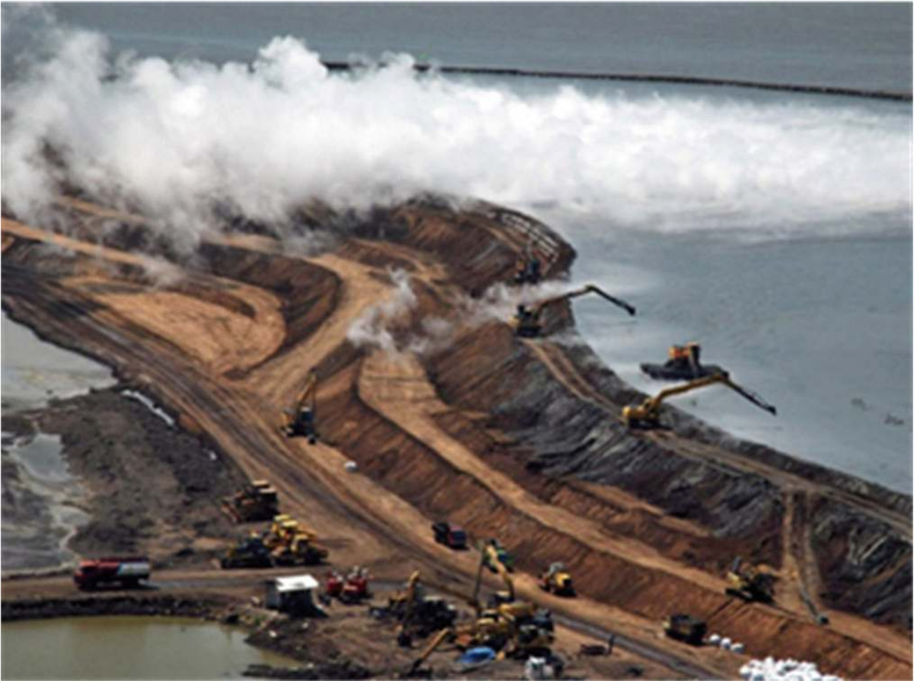
Fig. 23 Maintenance of dykes
