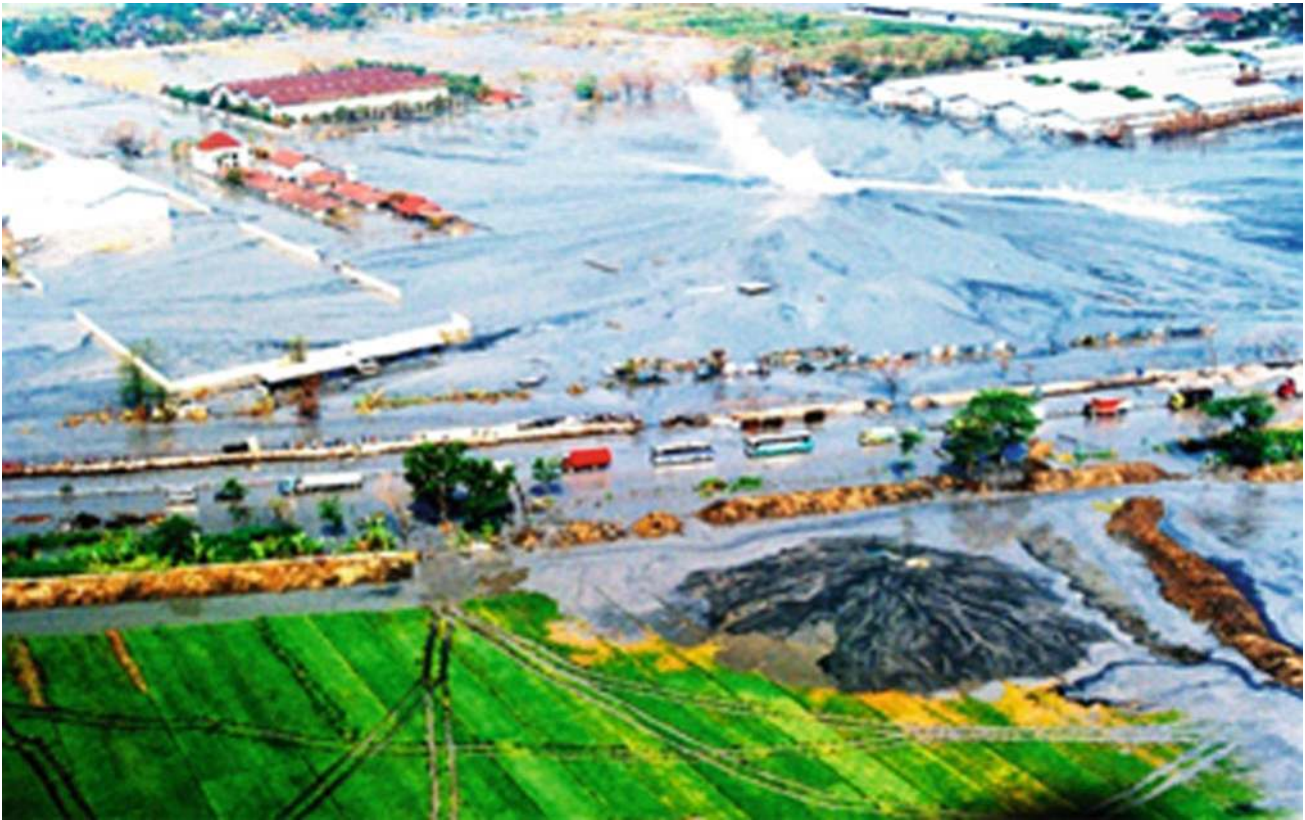
Fig. 11 Damage to area infrastructure (BPLS 2007)
