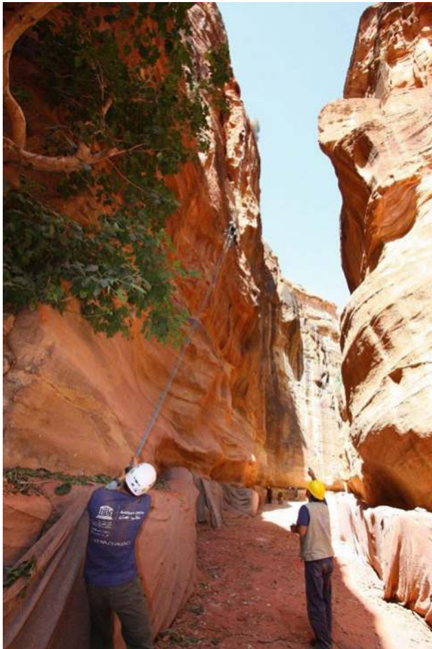
Fig. 2 Landslide risk mitigation works
