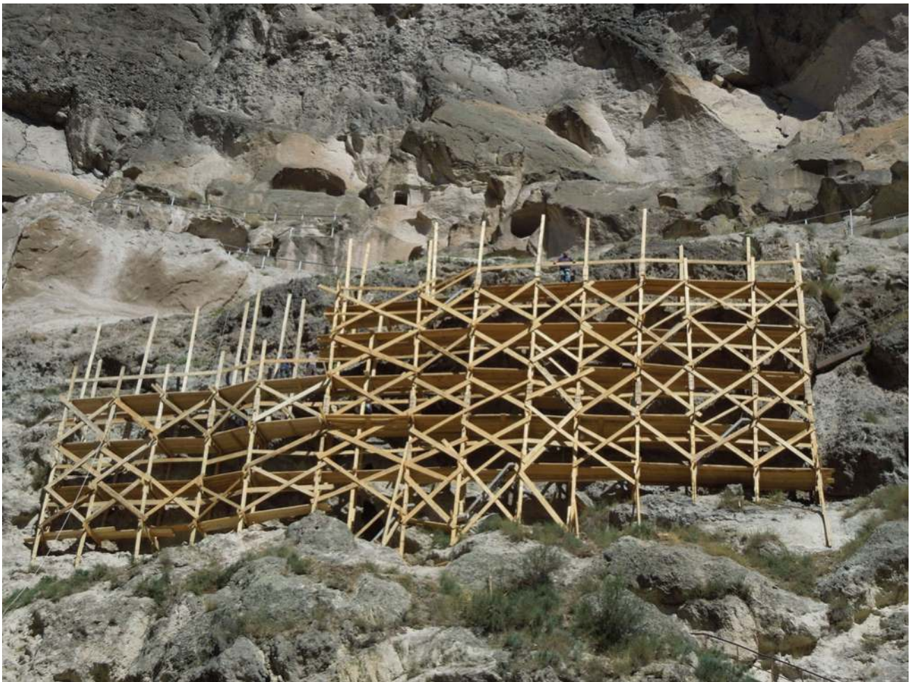
Fig. 30 The wood scaffolding realised in Vardzia
