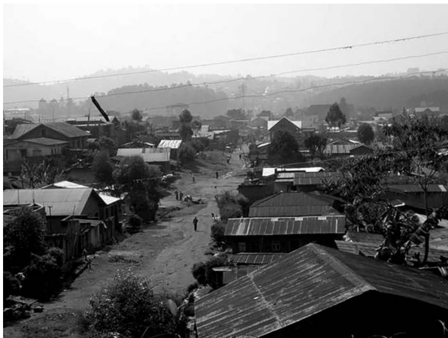
Figure 6.2 Street view with community-built electricity lines, Butembo, photographed 30 July 2010
