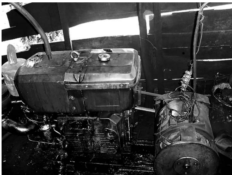
Figure 6.4 Commercial generator, photographed 2 August 2014, Keshero, Goma
