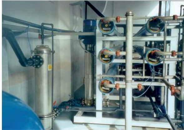
Figure 18 Reverse osmosis unit producing irrigation water for a green house in Gran Canaria, Spain
