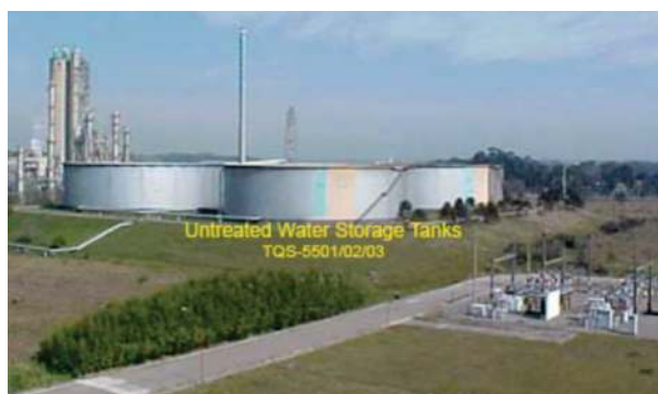
FIGURE 14 – UNTREATED WATER STORAGE TANKS OF REPAR REFINERY
