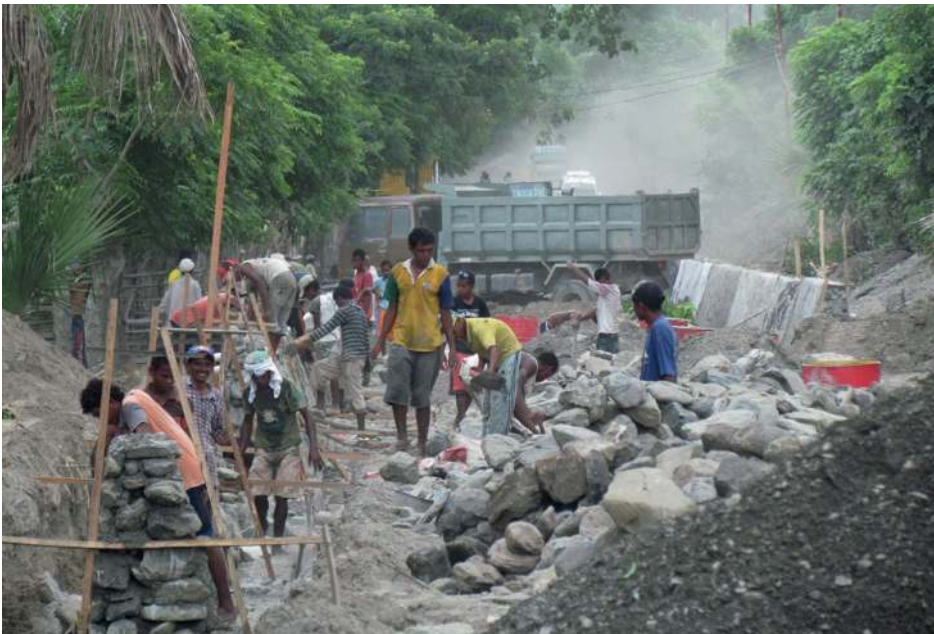
Figure 7.1 National road upgrading project.
