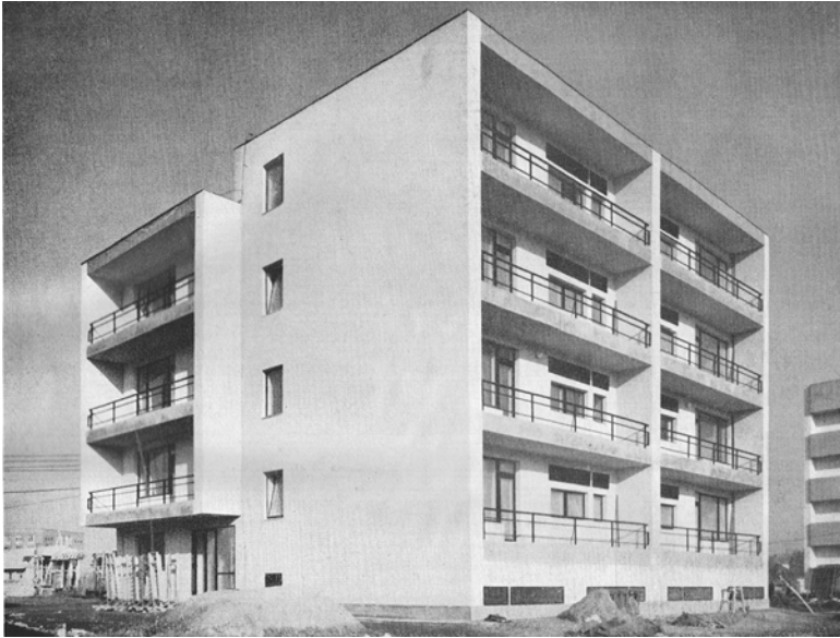
Figure 1: Apartment house, Budapest 1961. Architect: Olga Mináry (1929-2000). Mináry received the Ybl Prize for this building in 1964. Source: Magyar Építőművészet 1961, 1, 11.
