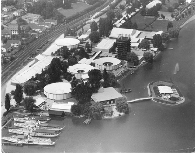
Figure 1: Aerial view, SAFFA 1958 on the Landiwiese along Lake Zürich, showing the pavilions, the SAFFA Tower and the SAFFA Island. Source: ETH-BIB-Zürich, Saffa-LBS_H1-021321.tif (Open access).
