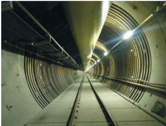
Figure 5. Stretch with steel ribs.
