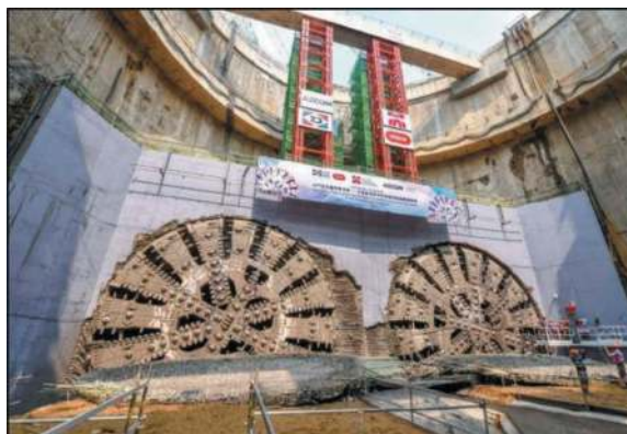
Figure 17. TM-CLKL – Twin TBMs (14m dia) break-out.
