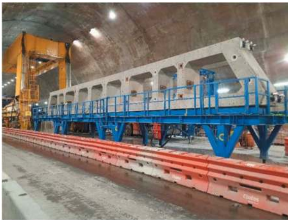
Figure 9. Loader for mezzanine beam installation.
