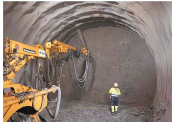
Figure 25. Sprayed concrete.
