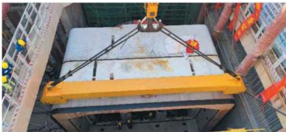
Figure 9. Pipe section lifting down well.
