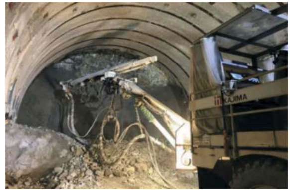
Figure 17. Face spraying by automated shotcrete.
