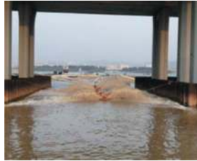
Figure 8. Backfilling of sand division unit.
