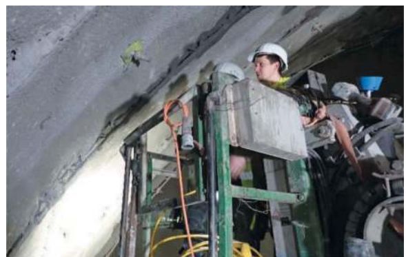
Figure 7. Geotechnical monitoring of rock bolts.
