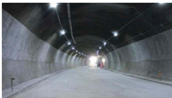
Figure 13. Relining by high strength shotcrete - Pilot application at “Manfreida” tunnel.
