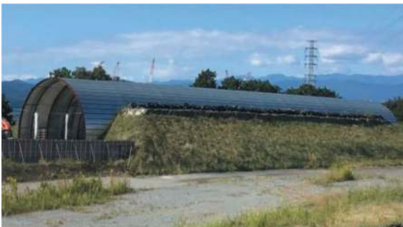
Picture 1. Mock-up tunnel.
