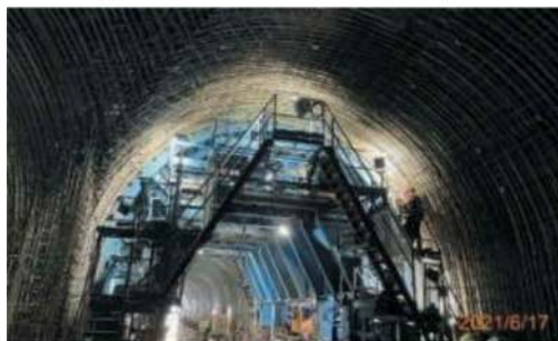
(2) Concrete lining for the desilting tunnel (2021.6)
