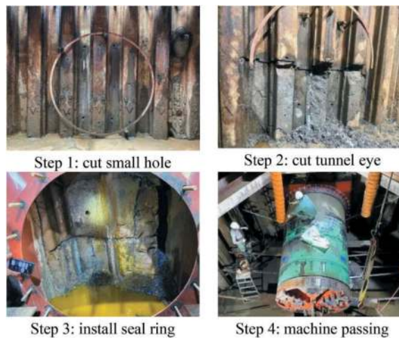
Figure 13. Check water leakage and cut tunnel eye.
