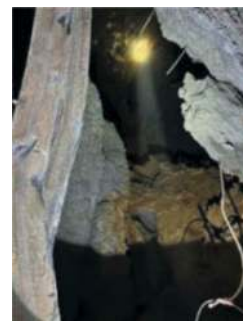
Figure 7. Karst cave revealed in tunnel.
