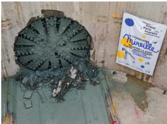
Figure 3. March 2022, TBM breakthrough at CMF.
