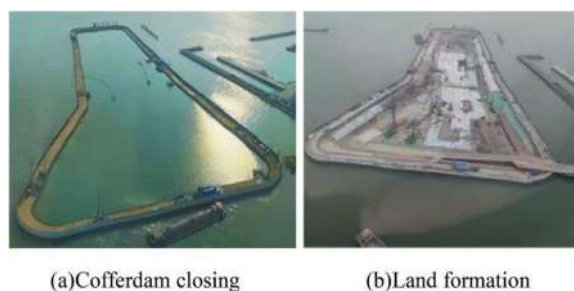
Figure 2. Bird's-eye view of cofferdam.
