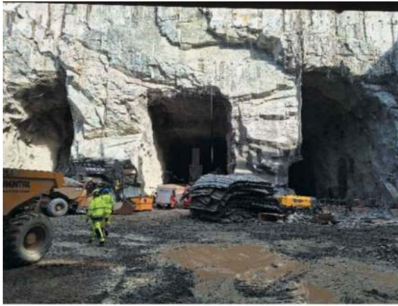
Figure 12. Pillars in the Center Pilot.
