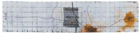
(a) The failure mode of the A-side
