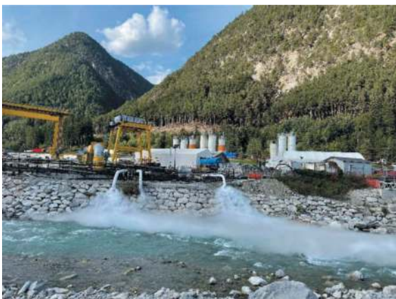
Figure 8. View of nitrogen vents.
