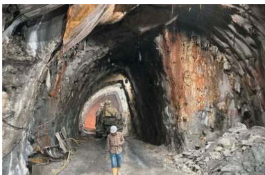
Figure 7. T01 P2 tunnel face.
