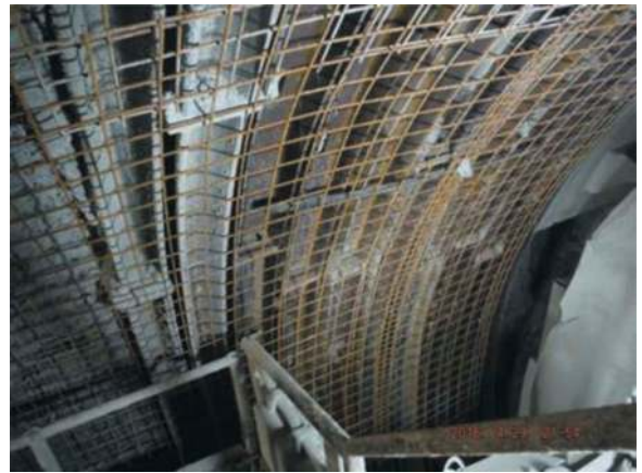
Figure 11. “Continuous steel profile” solution UNP 180 profiles set shoulder-to-shoulder.
