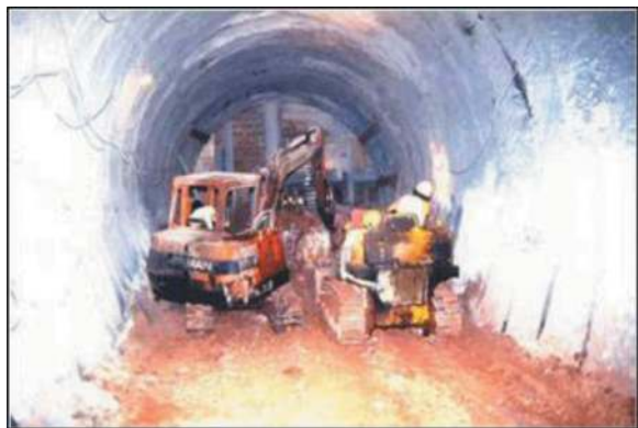
Figure 1. One of the first SCL tunnels for the North-East Line.
