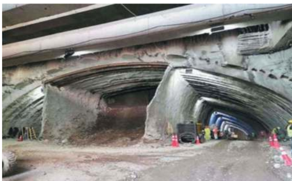
Figure 19. Hybrid tunnel portal at the ending of the cut & cover tunnel.
