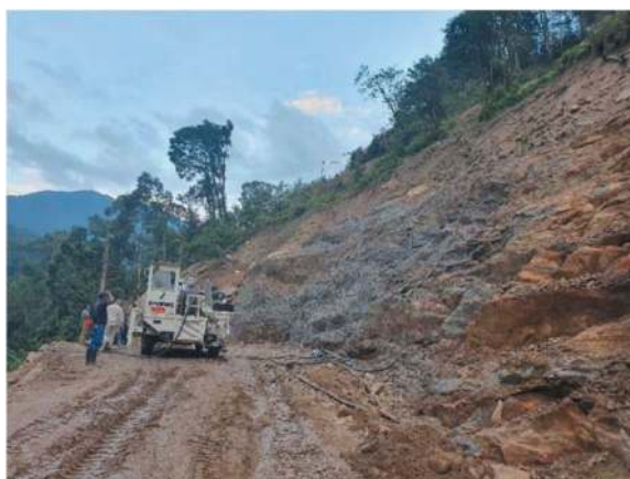
Figure 14. Adit construction at Kholongchhu.
