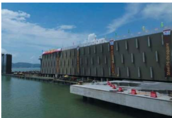
Figure 9. Successful landing of steel shell of immersed tunnel on Guishan Island.
