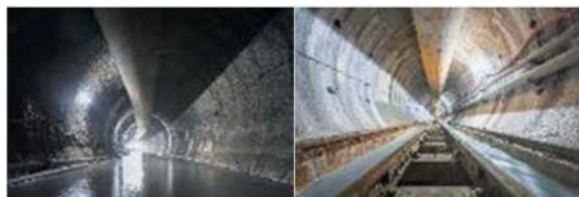
Figure 1. Support in headrace tunnel.
