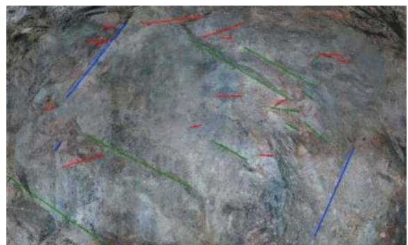
Figure 9. Result of geological sketching on tunnel face.
