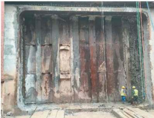
Figure 18. Actual picture of the steel box with wall at the end.
