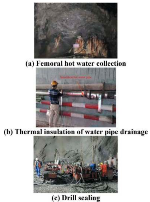
Figure 8. Heat source control.
