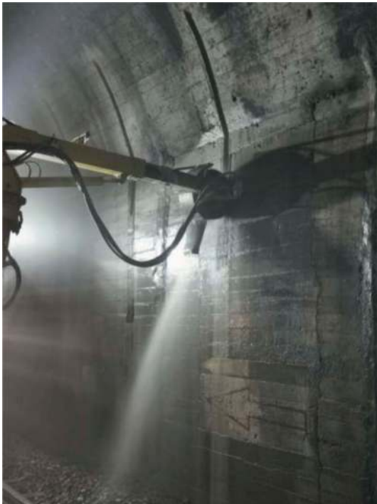
Figure 13. Slotting operation of the complete equipment for treating the defects of operating tunnels.
