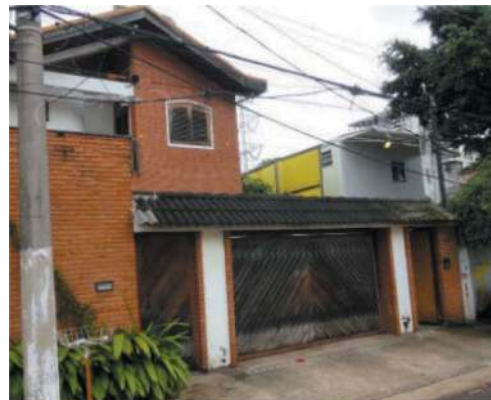
Figure 4. Photo of the house façade.
