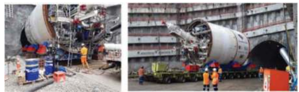
Figures 17 & 18. Shield transport down to the portal.
