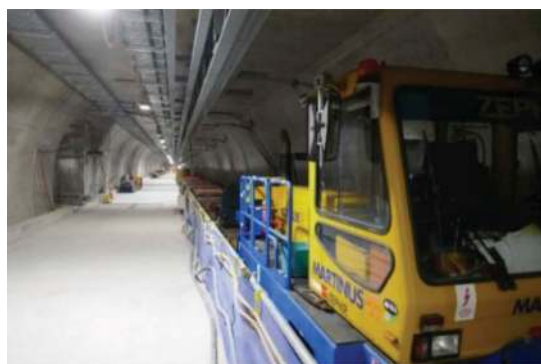
Figure 21. A zephir rail vehicle delivering tracks for installation at Karanga-a-Hape Station.
