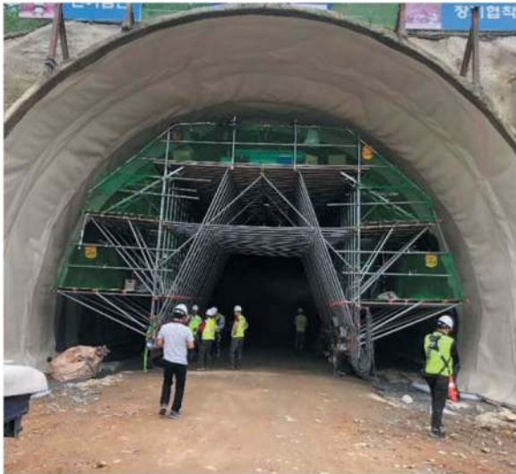
Figure 7. Tunnel in South Korea with SikaProof®-110.
