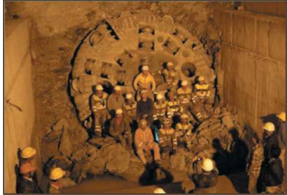
Figure 3. Breakthrough in inclined pressure shaft with TBM.
