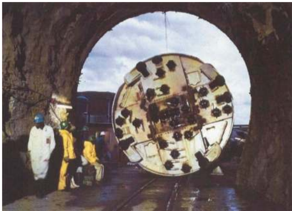
Figure 3. The MK15 open-type TBM at the tunnel portal.
