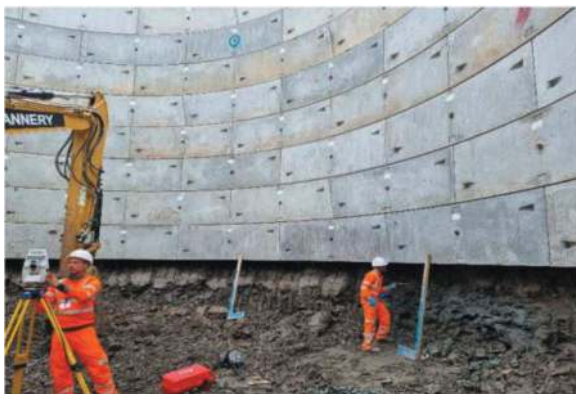
Figure 4. Bengeworth road shaft lining underpinning.
