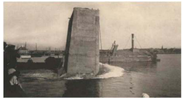
Figure 6. Aalborg Harbour (1906) launching caissons.
