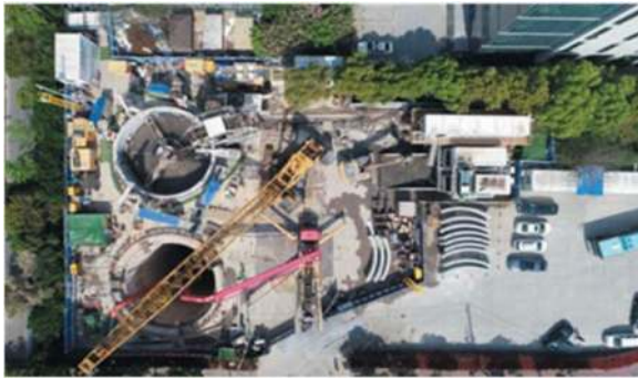
Figure 10. VSM Jobsite arrangement in Nanjing.
