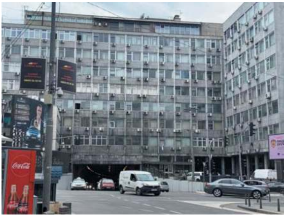
Figure 1. A rectangular motorway tunnel under a wide residential building at Belgrade, Serbia.
