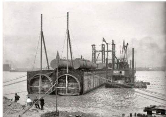
Figure 4. Tunnel element prepared for immersion.
