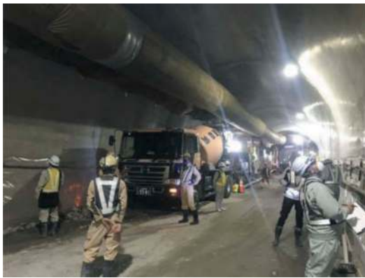
Figure 14. Practice test (construction site).
