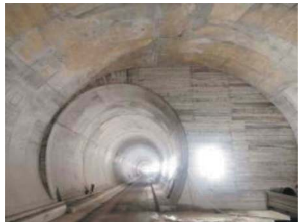
Figure 3. Final lining, change from single track to double track.
