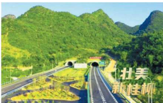
Figure 18. Photos of siding extra long tunnel.
