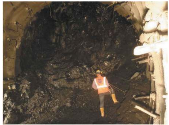
Figure 6. Excavation front in the fault zone of the Periadriatic Seam.
