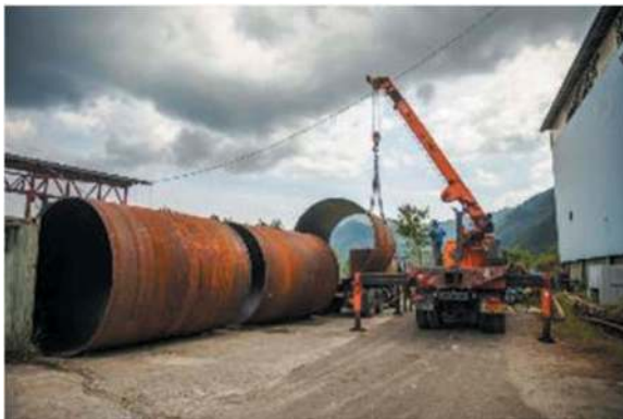
Figure 6. Assembled steel lining.
