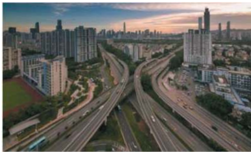
Figure 2. Situation of the base before construction.
