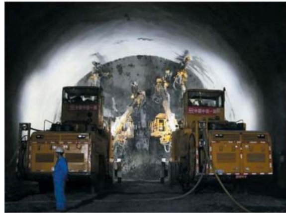
Figure 1. Automatic acquisition for the drilling parameters.
