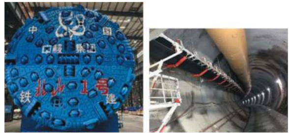
Figure 13. Physical cutterhead and tunnel formation.
