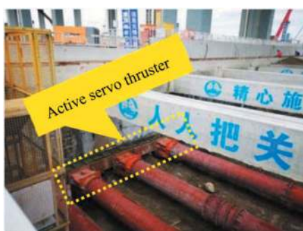
Figure 8. Steel support active servo system.
