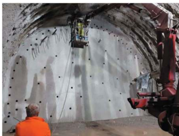
Figure 8. Consolidation of the tunnel face.
