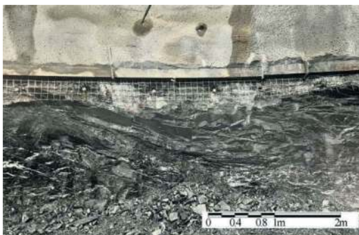
Figure 11. Typical Slate encountered at the South shaft-wall.
