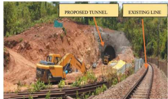
Figure 10. Pre-Cavity Photograph of Proposed & Existing Tunnel -1.
