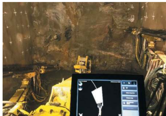
Figure 15. Drilling a grout curtain.
