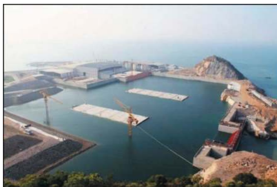
Figure 4. Tunnel element prefabrication and floating at casting yard (HZMB Link).
