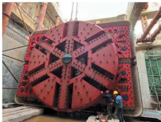
Figure 5. Actual picture of the cutter head of pipe jacking machine.
