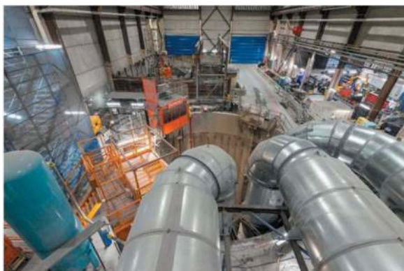
Figure 4. Lot 2 – access shaft to Albert Street cavern and acoustic shed.
