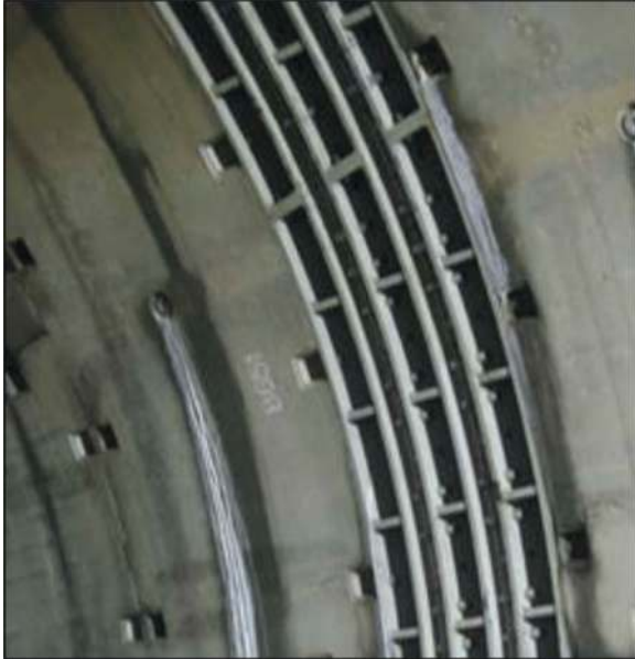
Figure 8. Seismic joint application on a TBM tunnel.
