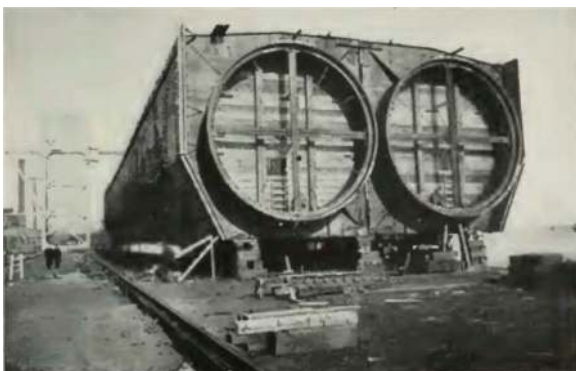
Figure 2. Completed tube at shipyard.
