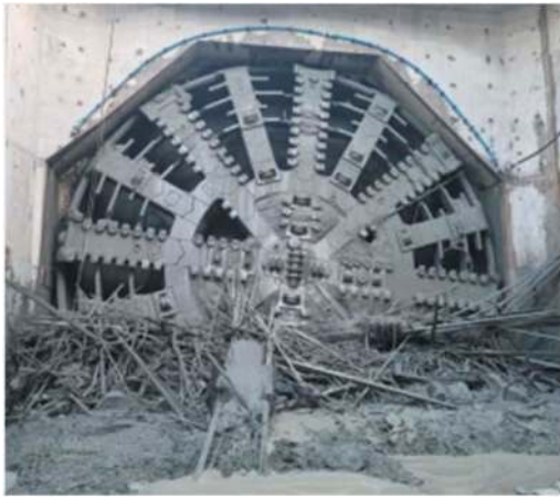
Figure 1. Silvertown break through southbound.
