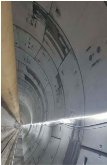
Figure 1. General view of the utility gallery during construction.
