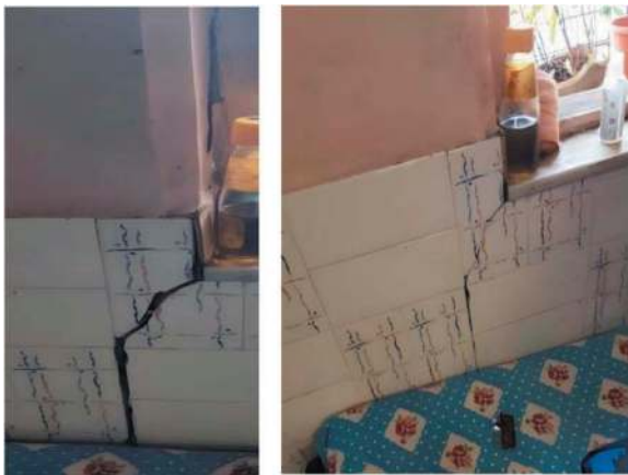
Picture 3a & 3b. Crack-2 prior to and after grouting measures.
