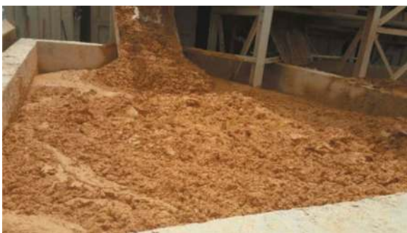
Figure 11. Muck Pit for sand.
