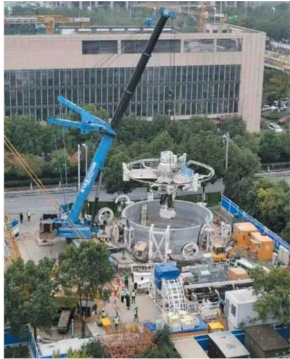
Figure 11. VSM lowered into start section of the first shaft.
