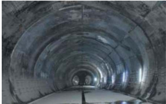
Figure 17. Final NATM cavern.
