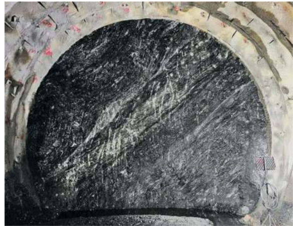
Figure 2. Typical carbonate Slate; overburden 380m (approx.).
