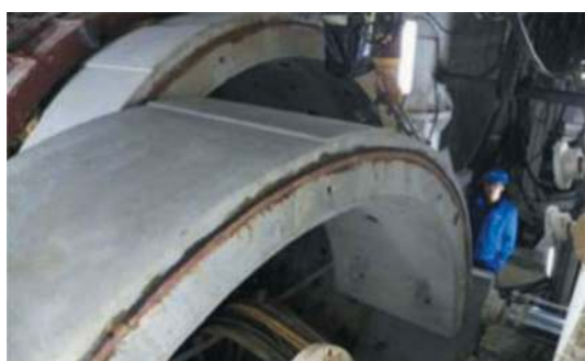
Figure 16. Installation of upper pipe.
