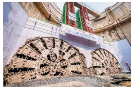
Figure 16. First double TBM breakthrough in hong kong.
