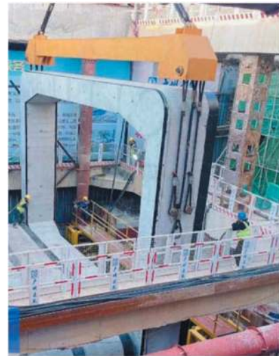
Figure 12. Down-hole after changing lifting point.
