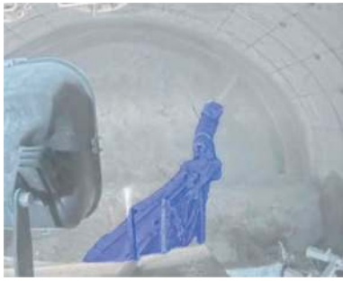
Figure 6. Identification of shotcreting machine booms by AI.
