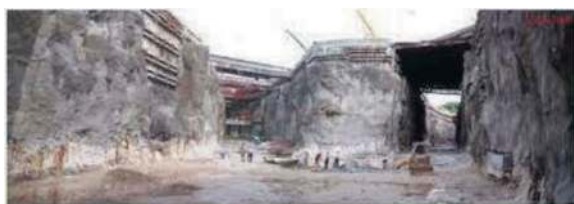
Figure 12. Excavation into limestone at north junction box.
