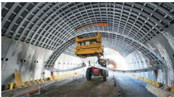
Figure 15. Relining by liner plates - Pilot application at “Castello” tunnel.
