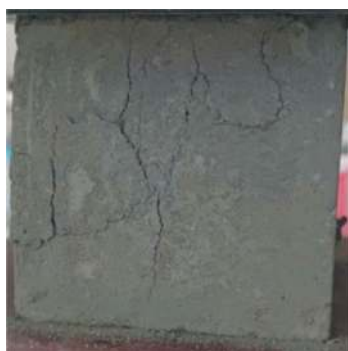
Figure 10. Crack propagation of fiber foamed concrete.
