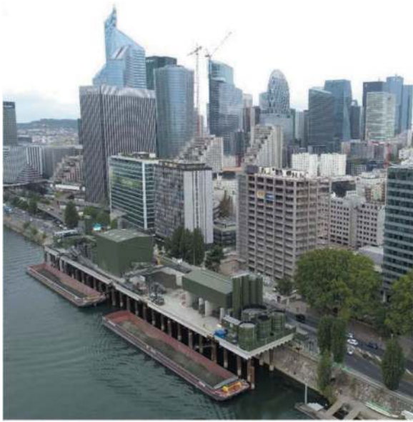
Figure 6. EOLE separation plant, Slurry TBM D11,4m – 6km.
