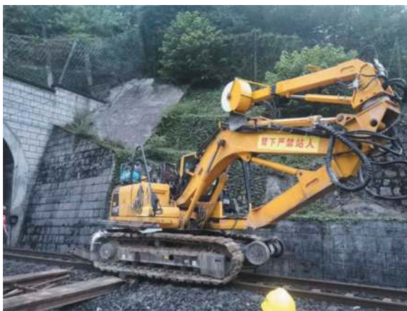
Figure 16. Photos of the equipment operating on the construction site.
