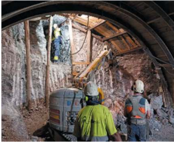
Figure 13. Heading front with a combination of manual means and small machinery.
