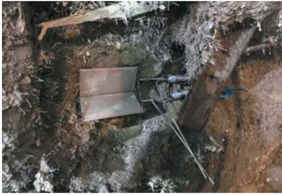
Figure 3. Installation of NATM pressure cells.
