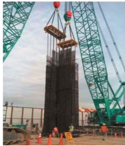
Figure 5c. Dwall cage tandem lifting.
