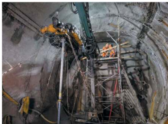
Figure 8. Injection work in the Hochstegen fault zone.
