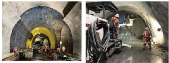
Figures 24 & 25. Karanga-a-Hape tunnel lining construction (left) & tunnel excavation (right).
