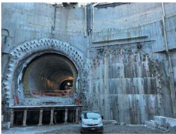
Figure 13. Consolidation section of the Isarco underpass.
