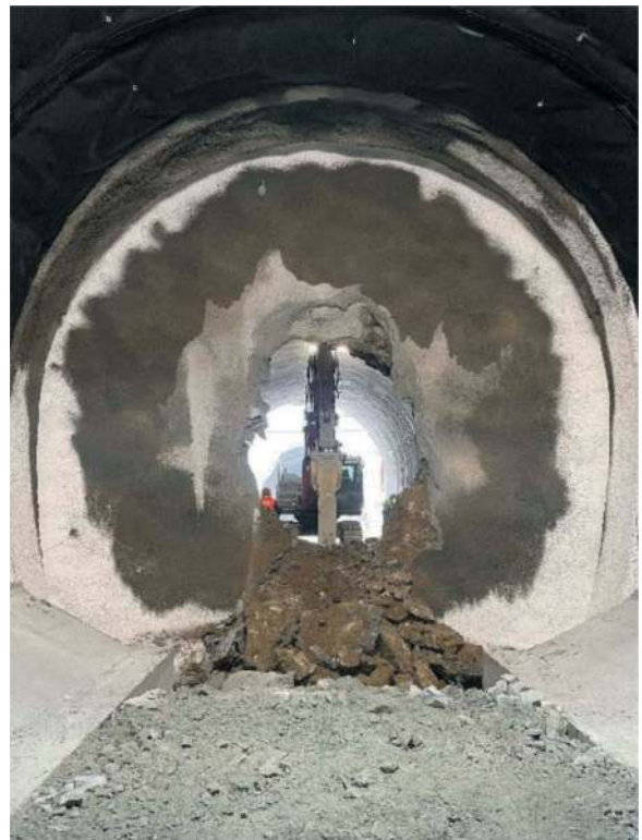
Figure 18. Final breakthrough under the Isarco river: GNBDI tunnel on 07/04/2022.
