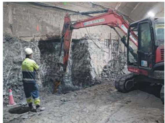
Figure 17. Excavation of a wall trench.
