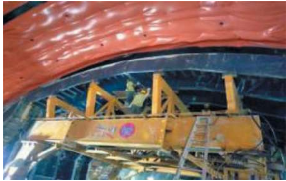
Figure 16. Gantry fixing for final lining.
