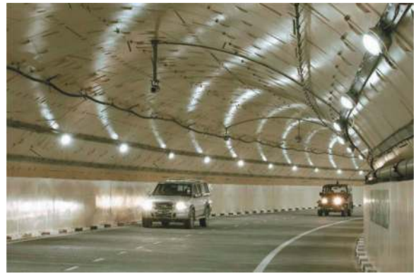
Figure 7. The motorway open to traffic (Mode 1 and 2).
