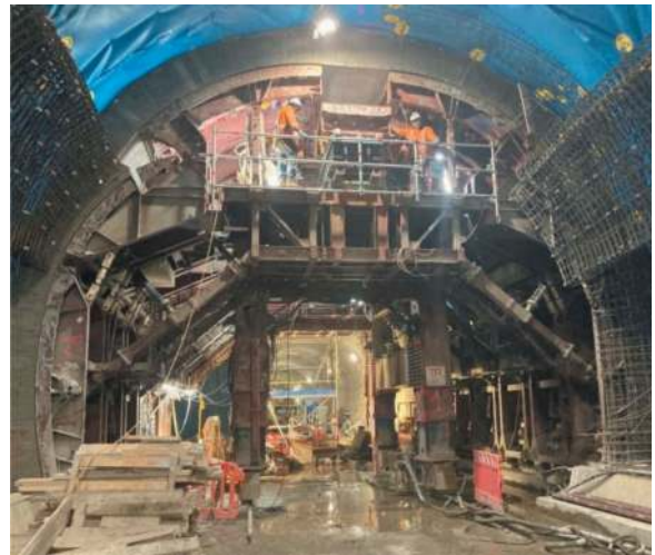
Figure 7. PT form during transition (central section about to be inserted).
