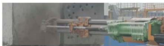
d Drilling test process-drilling for 3m
