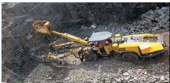
Figure 13. Rocket Boomer in operation at the main Tunnel.
