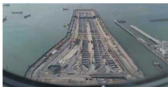
Figure 3. Bird's-eye view of excavation in cofferdam.
