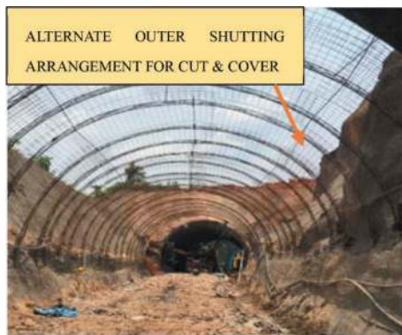
Figure 15. LG, Wire mesh & GI sheets for outer shuttering of Gantry.
