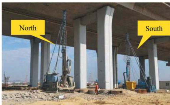
Figure 5. Symmetrical reinforcement grouting construction on both sides of bridge piers.
