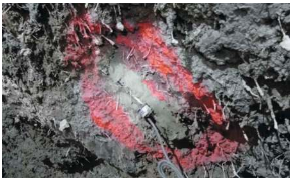
Figure 4. Installation of strain gauges.
