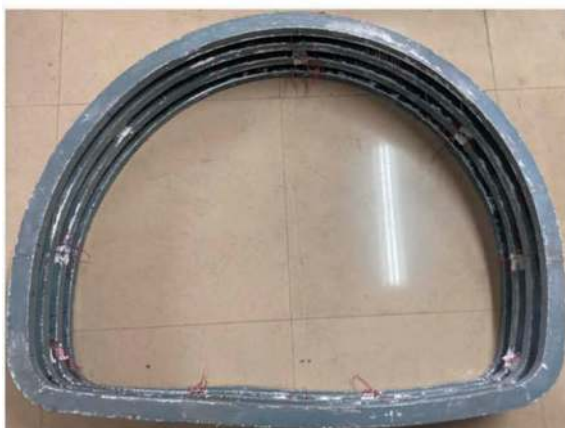
Figure 4. Overall failure of arch frame.
