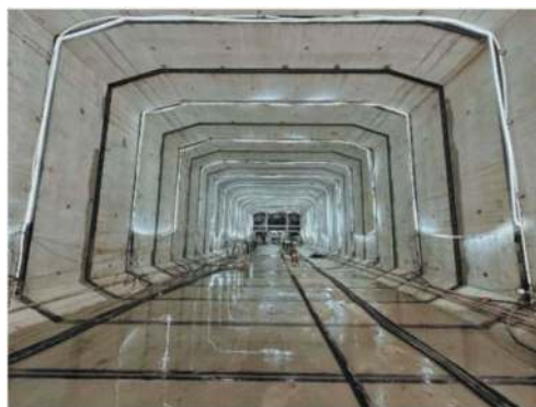
Figure 27. Actual picture of pipe jacking tunnel.
