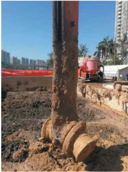
Figure 3. Solidification equipment used on site by Shenzhen Metro.
