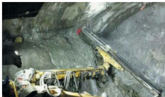
Figure 2. Drilling process for MPBX extensometers.
