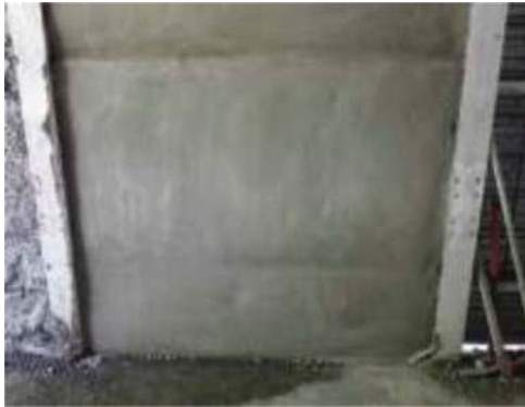
Figure 10. Surface finish after spraying (Lower level).
