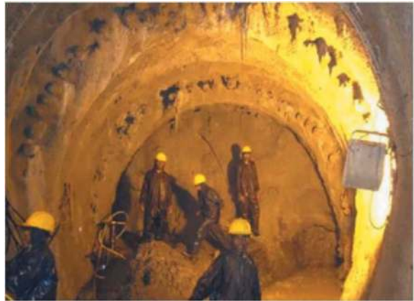
Figure 7. Pipe umbrella support in Dagachhu HRT.
