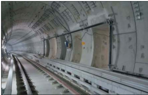
Figure 22. The five completed ventilation passages.
