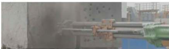
c Borehole test process-drilling for 2m
