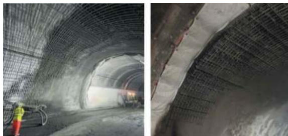
Figure 12. “Manfreida” tunnel construction site – relining by high strength shotcrete.
