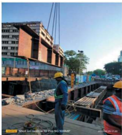
Figure 9. Steel decking dismantling.
