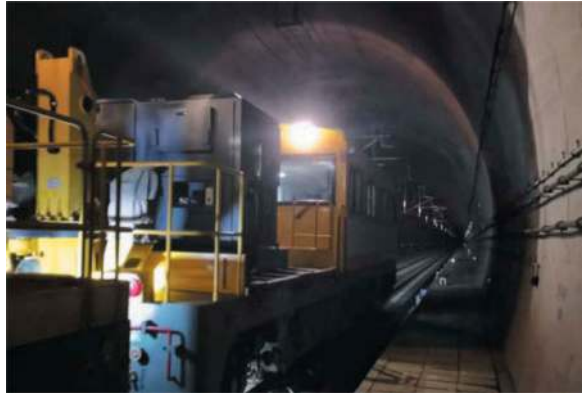
Figure 4. Inspection process in a single hole double track railway tunnel.
