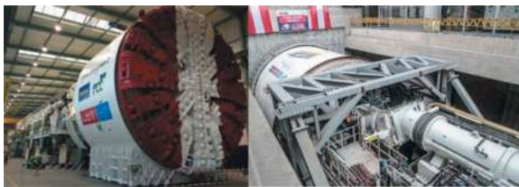
Figure 9. TBM VD at the factory and at site before launching.
