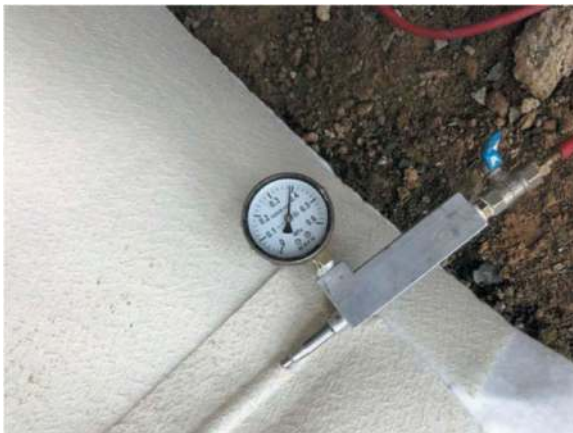
Figure 16. Test of welding seams.
