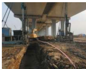
Figure 15. Soil reinforcement in passive area.
