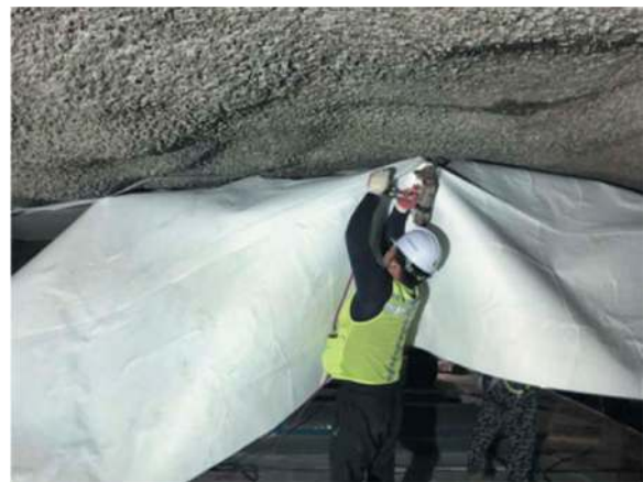
Figure 14. Fixation of the membrane using the geotextile.
