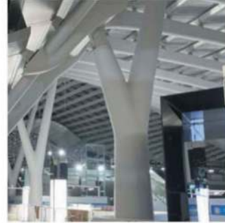
(A) centripetal joint bearing support
