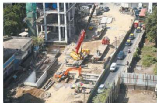
Figure 10. Breaking of RCC decking.
