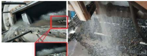
Figure 15. Water and gravel extracted by the screw conveyor.
