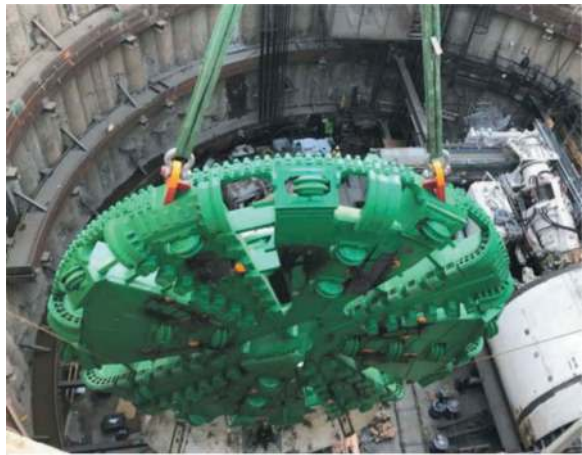
Figure 11. BL TBM “Aura” cutterhead being lowered into the launch shaft.
