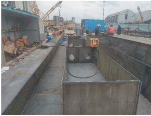
Figure 17. Connecting wall steel box processing.
