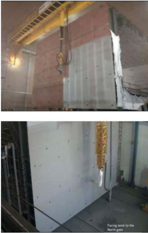
Figure 13. Application of intelligent painting.
