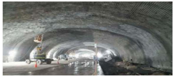
Figure 20. Bifurcation cavern of Los Militares N entrance branch.
