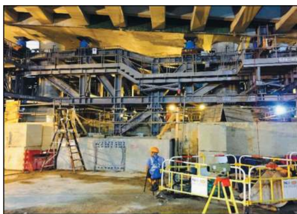
Figure 8. Underpinning of Canal Road Flyover to facilitate pile obstruction removal.
