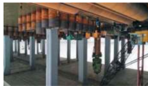
Figure 10. No-resonance drilling process.
