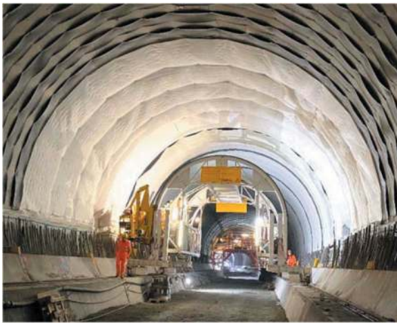
Figure 12. Scaffolding for membrane installation.
