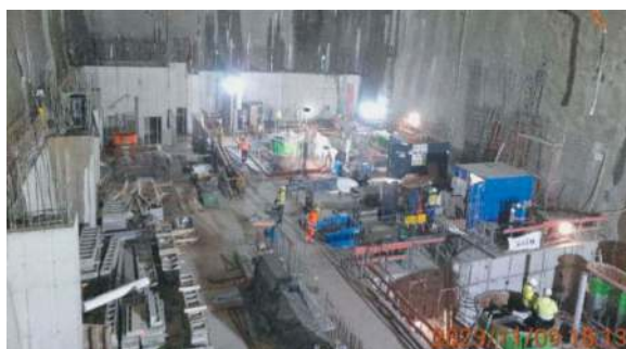
Figure 13. Installing of mechanical part and inner lining.
