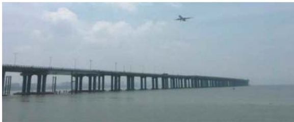
Figure 2. Existing Guangzhou-Shenzhen coastal expressway.
