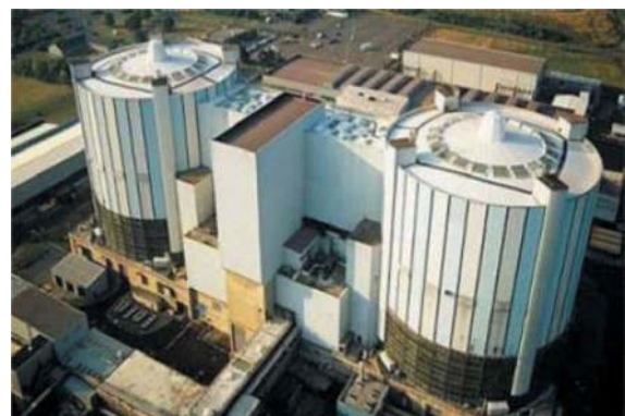
Figure 5. Oldbury reactor buildings.
