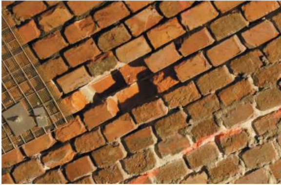
Figure 3. Detail of the masonry vault and of the first aid intervention.
