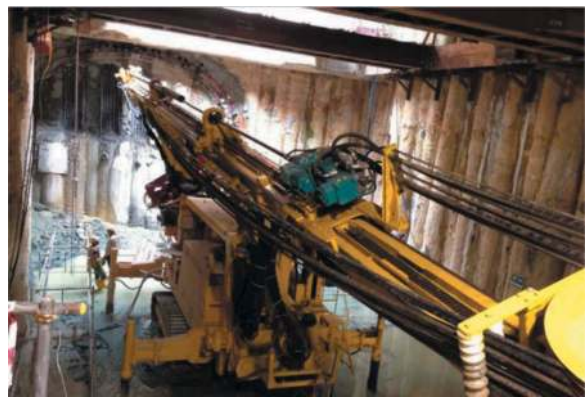
Figure 26. Pipe roofing by horizontal drilling rig.
