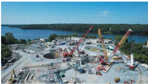
Figure 11. Main site aerial picture during TBM assembly.
