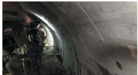
Figure 6. Tunnel segment support.
