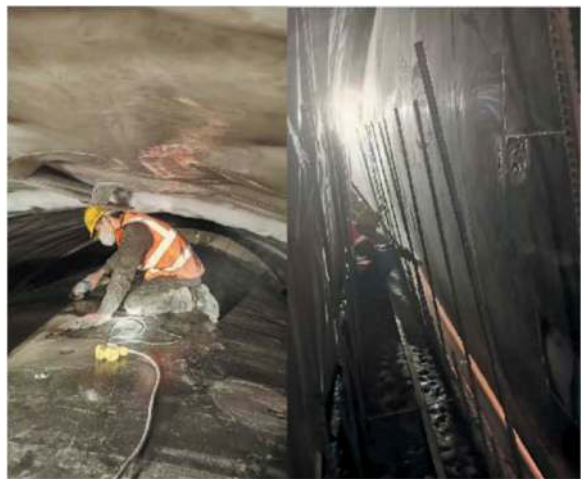
Figure 1. Manual grinding of secondary lining trolley in tunnel.
