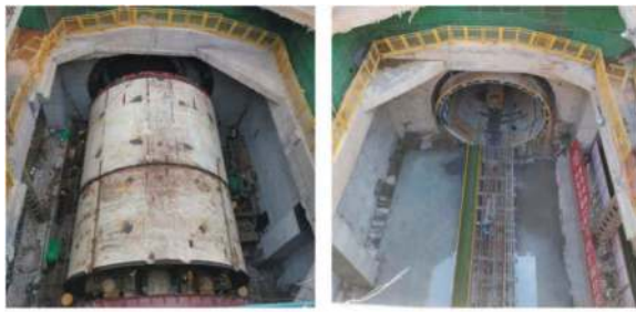
(a) Before the large shield (b) After the large shield
