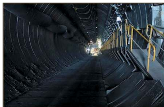
Figure 2. Long access tunnel is at 16.7% incline.
