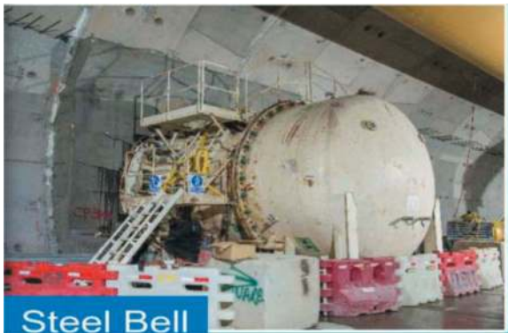
Figure 13. Steel pressurized chamber for receiving mini-TBM.
