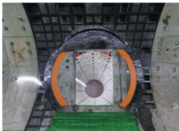
Figure 11. CP opening structure.
