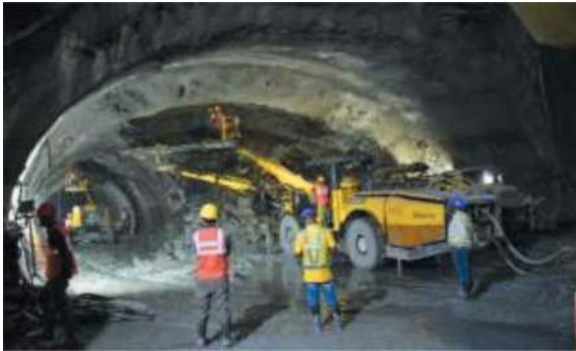
Figure 13. Crossover end wall shotcrete.
