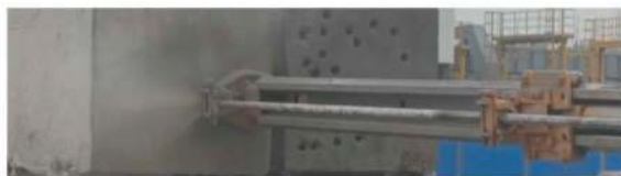
b. Borehole test process-drilling for 1m
