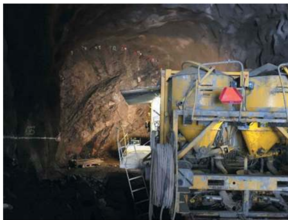
Figure 16. Grouting unit during the injection of a grout curtain.
