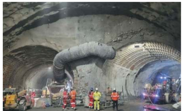
Figure 13. Excavation works inside the tunnel adit La Praz.
