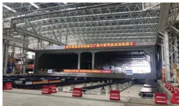
Figure 27. First steel sandwich element casting construction (Picture by Ying Li in 2019).
