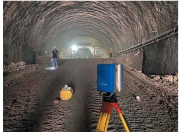
Figure 4. The on-site operation of the Z+F5016 three-dimensional laser scanner.
