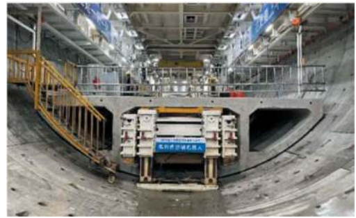
Figure 11. Arc-shaped components assembly robot on-site operation.
