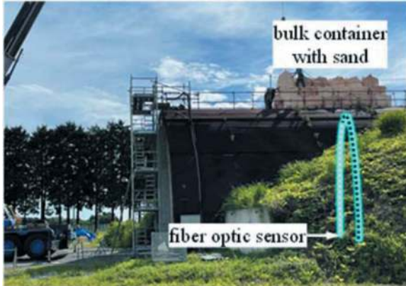
Figure 5. Loading test with bulk container.
