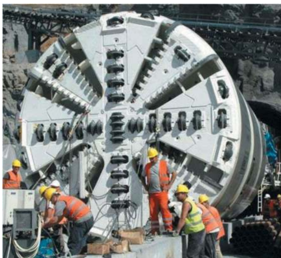
Figure 2. TBM used in Kartal Kaynarca tunnel.
