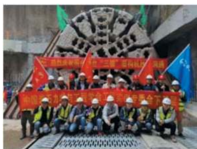
Figure 13. A three-mode TBM completes the first tunnel boring.
