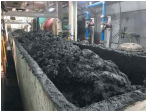
Figure 13. Muck skip for soil disposal (EPB TBM).
