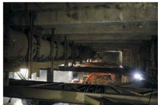
Figure 8. Supporting of 1450 mm water pipeline below rcc decking at sitaladevi station.
