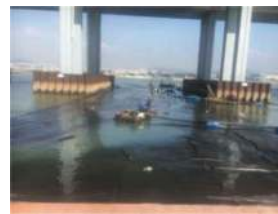
Figure 5. Sand backfill process.
