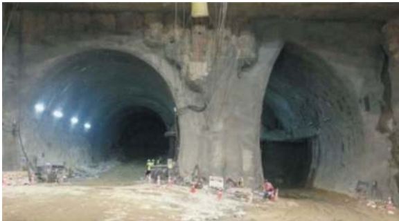
Figure 28. A partial stage of the 2-Arches tunnel excavation.
