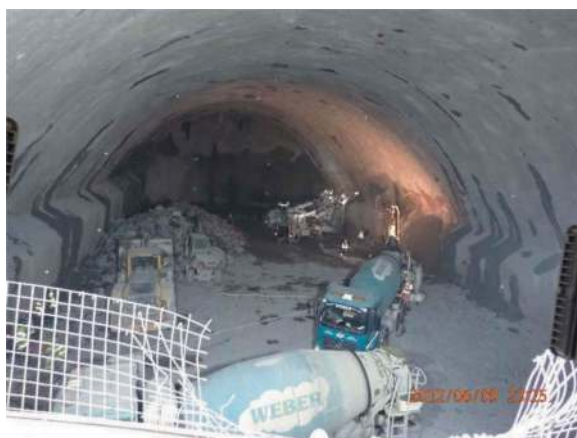
Figure 12. Excavation works in the cavern in June 2022.
