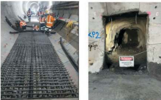
Figure 19. Reinforcement for first stage concrete and cross passage opening without lintel.
