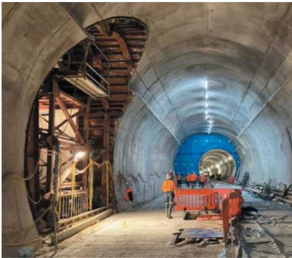
Figure 9. Junction formwork.
