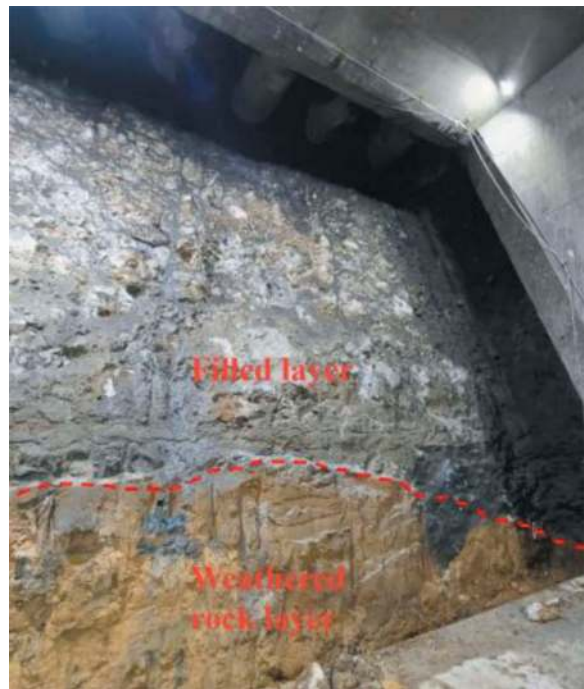
Figure 4. Excavation surface of the grouting area.
