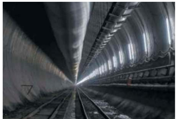
Figure 5. Tunnel lining with universal tubing rings.
