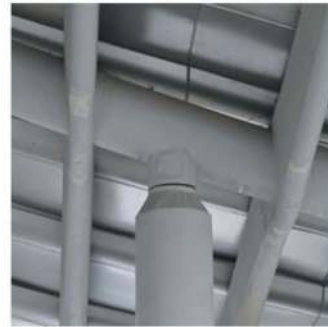
(A) centripetal joint bearing support
