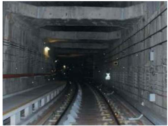
Figure 16. Extensive monitoring of the live CCL tunnels.
