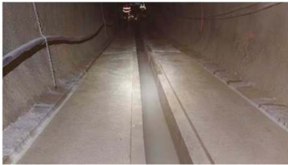
Figure 10. Completed drainage niche.
