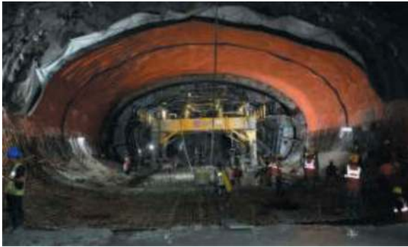
Figure 14. Waterproofing & rebar work in progress.
