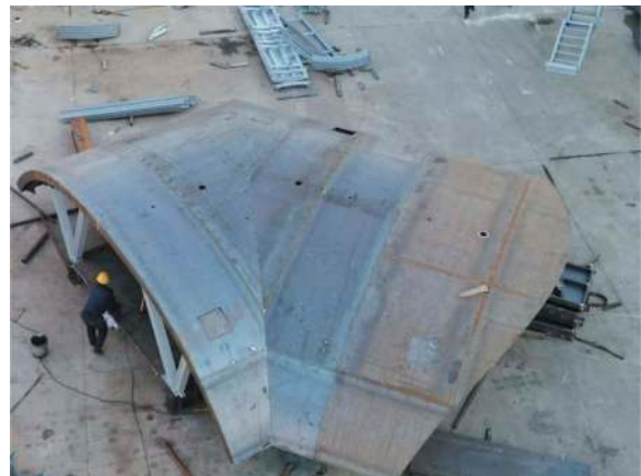
Figure 17. Adit A4 Crown formwork skin during manufacture with corner and junction piece.
