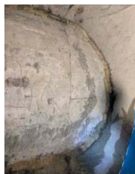
Figure 18. Primary grouting materials filled up TBM TAIL VOID.
