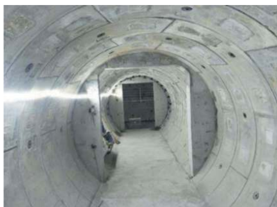
Figure 10. CP after segment erecting.
