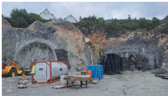
Figure 12. Kolltveit tunnel, West portals: the construction site in July 2023.
