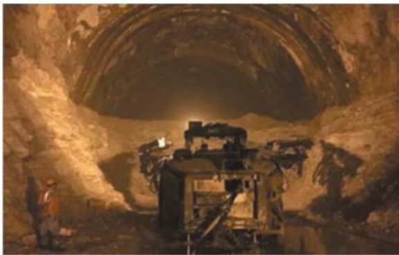
Figure 9. Top heading and Benching in Punatsangchuu 2.
