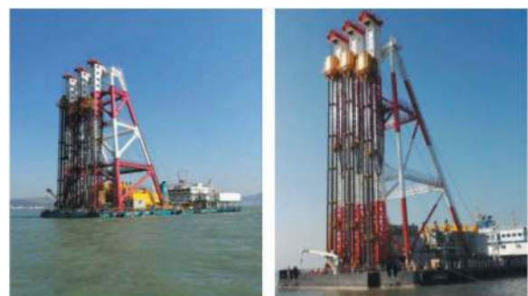
(a) DCM construction ship (b) On-site construction photos
