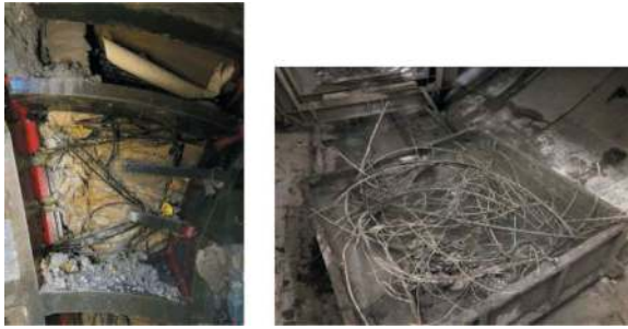
Figure 23. Ground anchors from excavation spoil.
