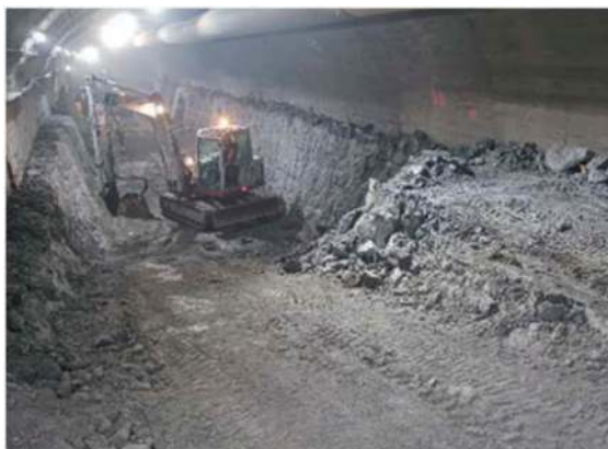
Figure 15. Bench excavation and transition ramp to the heading front.
