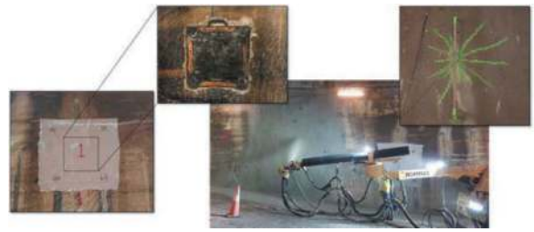
Figure 4. Photos of the large-scale field testing on shotcrete lining.
