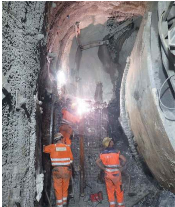
Figure 13. Excavation of one lateral side tunnel to free the cutter head.
