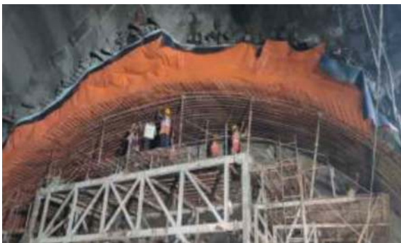
Figure 15. Overt rebar fixing work in progress.
