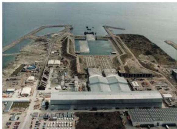
Figure 13. Øresund tunnel element fabrication.
