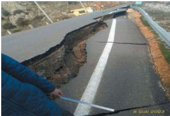
Figure 15. Cracks and openings on the crest of the dam body.
