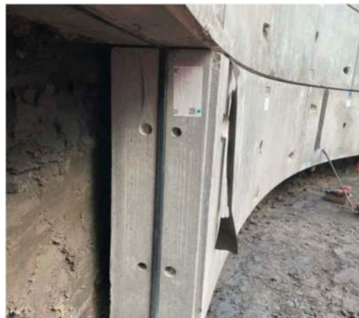
Figure 5. Bengeworth road shaft lining underpinning.
