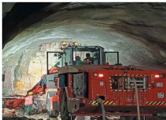
Figure 14. Tam rock boomer in operation at escape tunnel.
