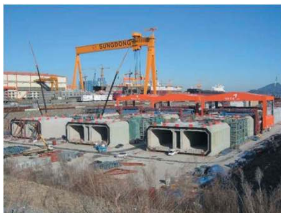
Figure 11. Busan-Geoje immersed tunnel, casting yard.
