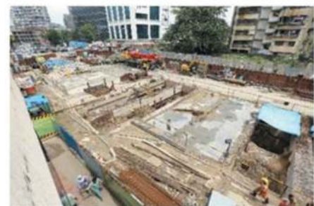
Figure 6. Construction of RCC decking.
