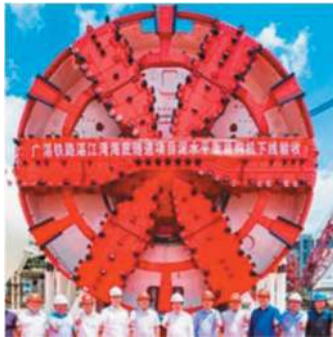
Figure 10. Zhanjiang Bay Tunnel of Guangzhou-Zhan High Speed Rail.
