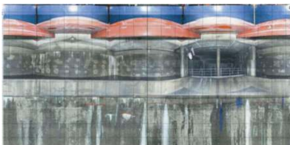
Figure 5. 360° panoramic image of the shaft surface.
