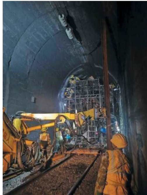
Figure 14. Slotting operation of the complete equipment for treating the defects of operating tunnels.
