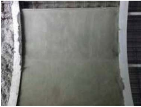
Figure 9. Surface finish after spraying (Upper level).
