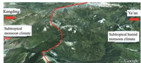
Figure 6. Climate difference between two ends of the Erlangshan tunnel.
