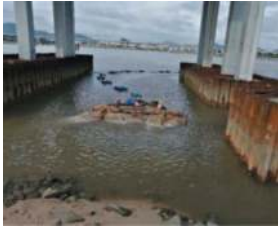
Figure 7. Backfilling of sand division unit.
