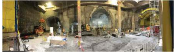
Figure 23. MC20, Adits 4 & 5 connections to Beresford Square shaft.
