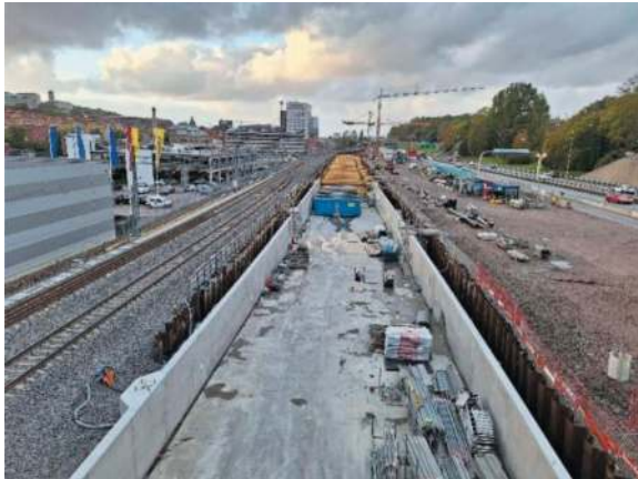
Figure 4. Almedal trough and tunnel section.
