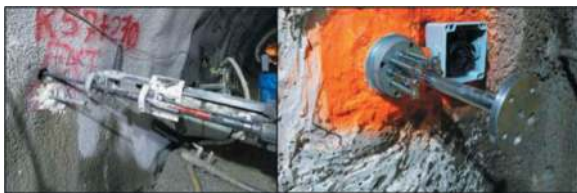
Figure 15. Installation process for MPBX extensometers in tunnels.
