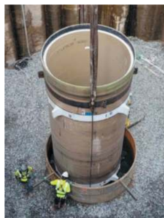
Figure 6. Drop pipe installation.
