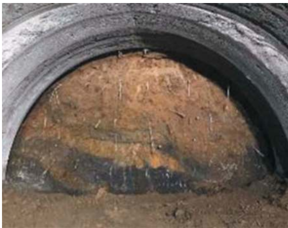
Figure 5. Face conditions of landslide deposits.
