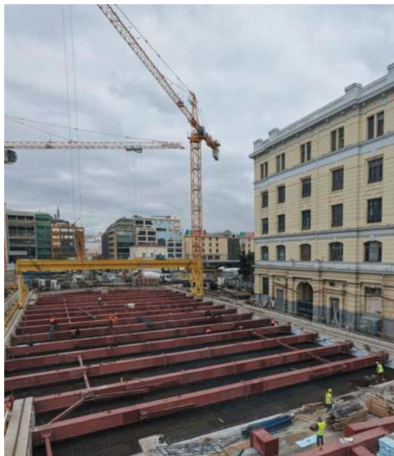
Figure 3. Retaining structure with emphasis in the struts during the construction phase.
