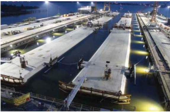
Figure 5. 2 nd Midtown Tunnel dry dock, Virginia USA.
