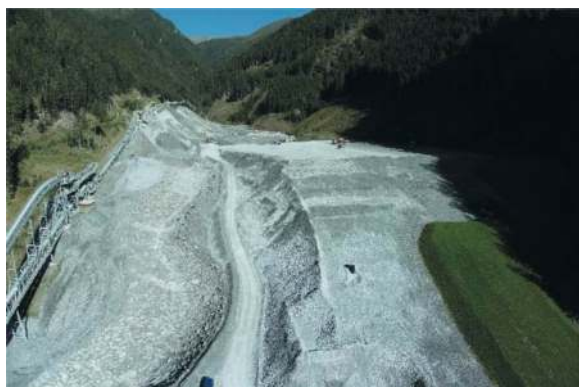
Figure 8. View of the Padaster valley spoil disposal site during the construction.
