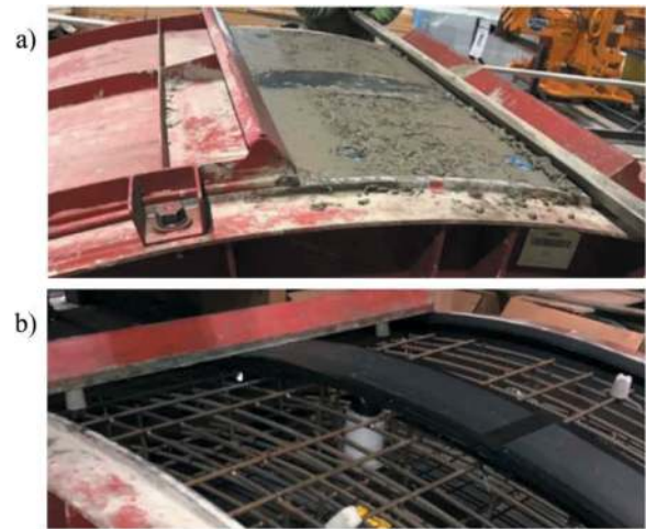
Figure 2. Insertion of O-ring box inside formworks and reinforcement cage (source: Optimas).
