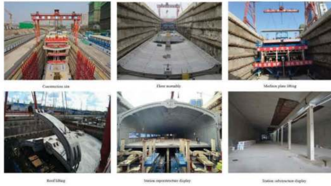
(b) On-site assembly of prefabricated station structure
