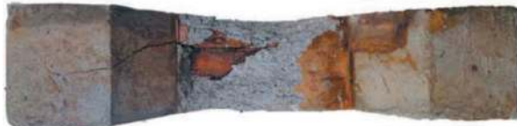
(c) The failure mode of the C-side
