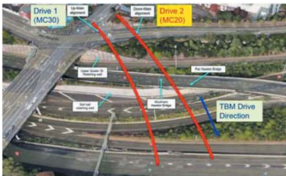
Figure 19. CRL Tunnels at CMJ (facing South).
