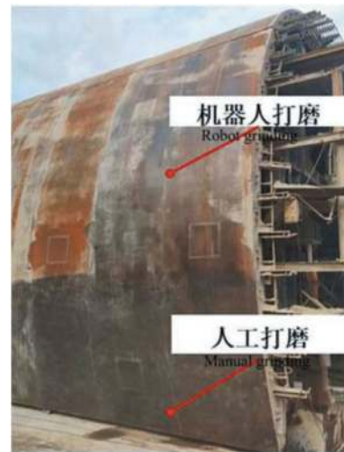
Figure 14. Comparison between manual operation and robot operation.
