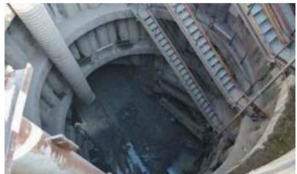
Figure 11. Access shaft for crossover.
