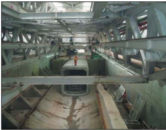
Figure 19. Chong Ming south tunnel during construction.
