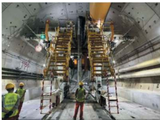
Figure 16. Rotation and forward of partition walls.
