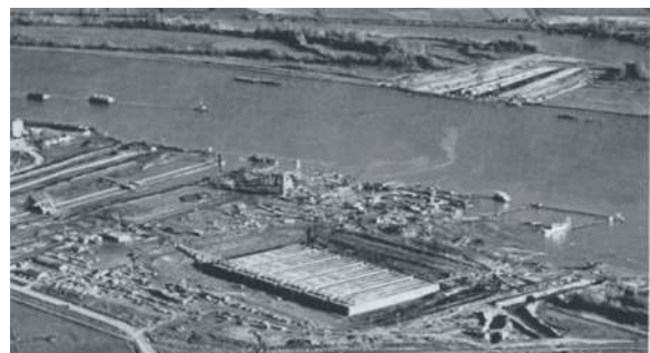
Figure 9. Deas Island Tunnel (1958).
