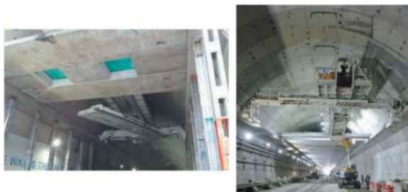
Figure 17. Launching gantry – overhead ventilation duct slab installation.
