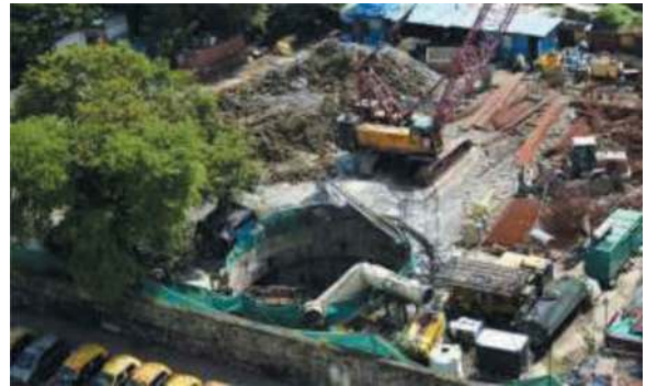
Figure 10. Aerial view of shaft during construction.
