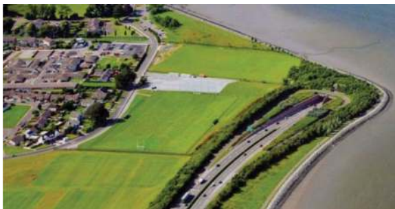
Figure 3. Reclaimed southern approach at Jack Lynch Tunnel.
