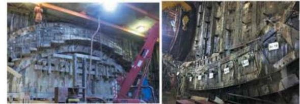
Figure 29. Completion of upper and lower halves propulsion.
