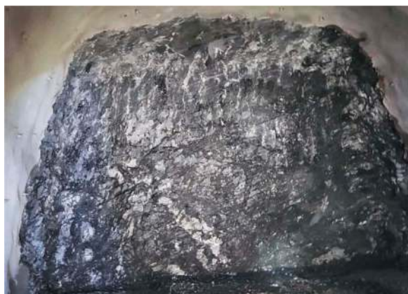
Figure 14. CHT excavation face.
