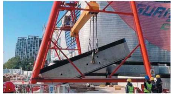
Figure 11. The pitch is erected by the eccentric vertical roll hole before it is lowered into the well.
