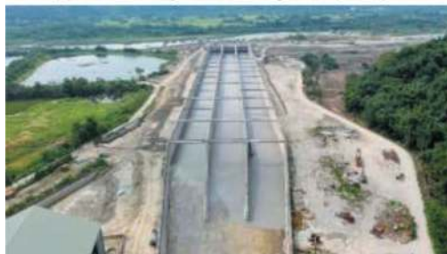
(3) Outlet and deposition pool structure
