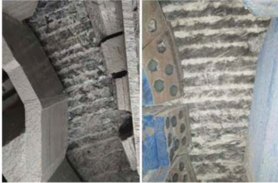
Figure 12. The tunnel face of high-strength and highly abrasive hard rock formations.
