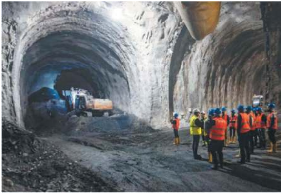
Figure 3. Photo central tunnel Emergency stop and cross passages.
