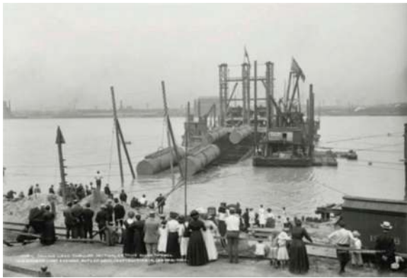
Figure 5. Immersion in progress.
