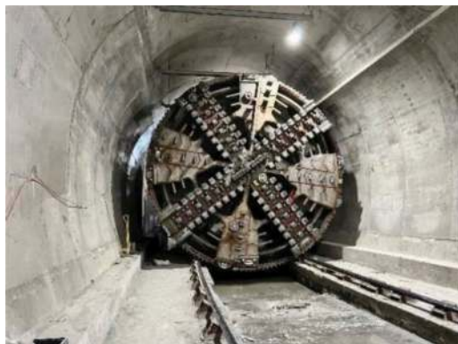
Figure 20. TBM transition in KHP MC20 mined tunnel with permanent lining.
