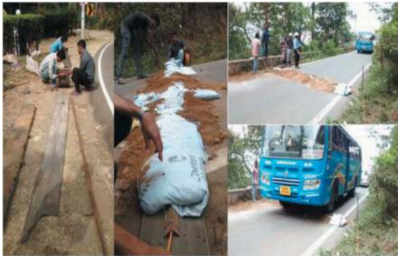
Figure 4. Imaging cable crossing the highway.
