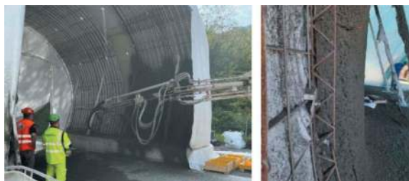
Figure 11. “San Fermo” tunnel - Field test of shotcrete application.
