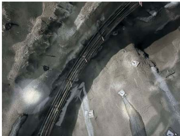
Figure 8. Rebars of RRSII prior to application of sprayed concrete.
