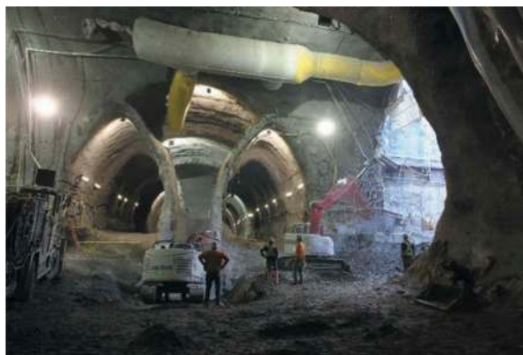
Figure 1. Underground station Cavern (Eglinton LRT project, Toronto).
