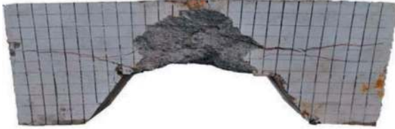
(b) The failure mode of the B-side
