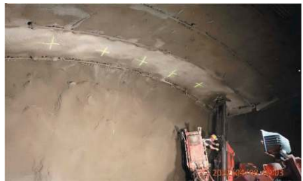
Figure 6. Installing GEWI 32 Anchor bolts 9 m.
