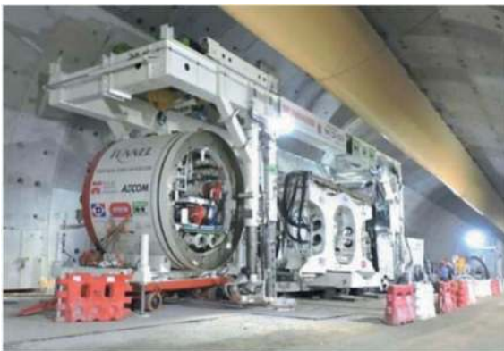
Figure 14. Cross passages with MTBM.
