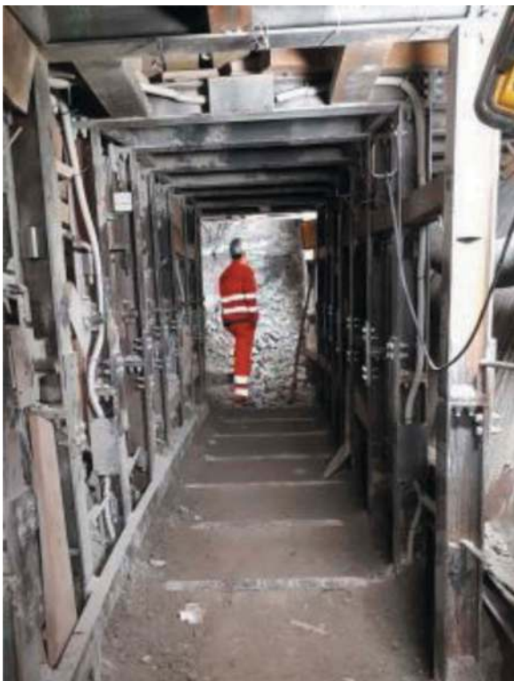
Figure 8. Lateral tunnel parallel to the TBM shield.
