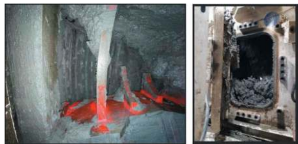
Figure 10. Tunnel face inspection during maintenance.
