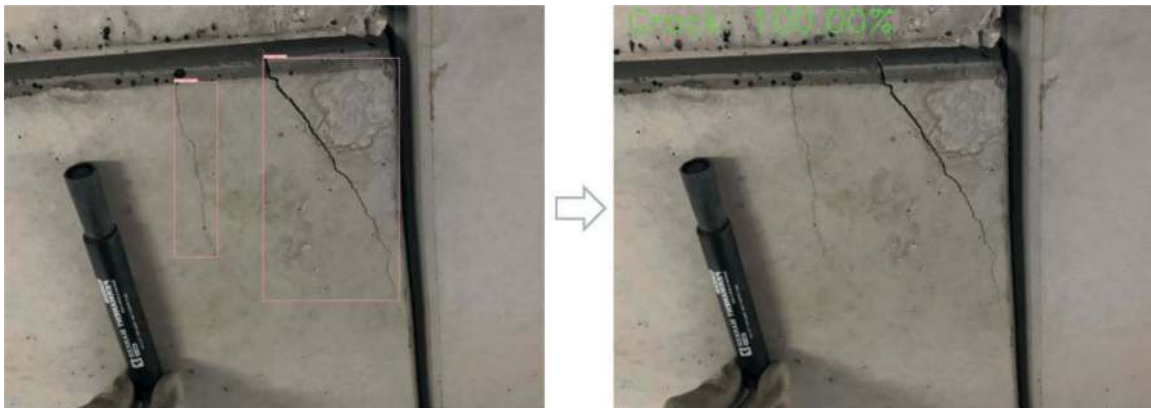
Figure 9. Examples of crack detection utilizing YOLOv8, a cutting-edge computer vision model developed by Ultralytics.
