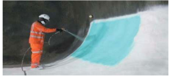
Figure 1. Liquid membrane application on the tunnel surface (Bridgepreservation, 2013).
