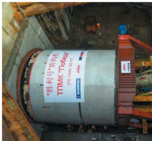
Figure 8. General view of the head part of the pobeda TBM.
