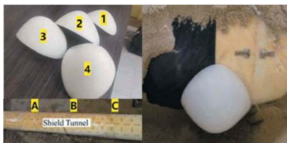
Figure 5. Degree and location of damage.
