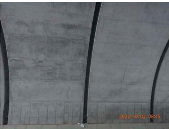
Figure 9. Slots between the arch elements.
