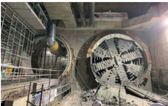
Figure 13. TBM MC20 drive breakthrough at Aotea station.
