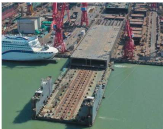
Figure 8. Successful transfer of steel shell of immersed tunnel transportation.
