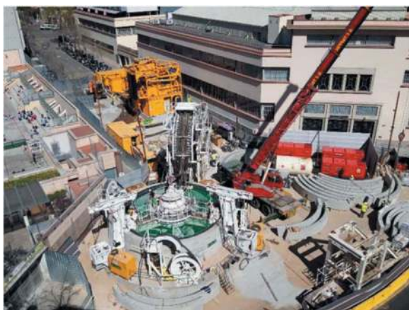
Figure 5. VSM Jobsite arrangement in Barcelona.
