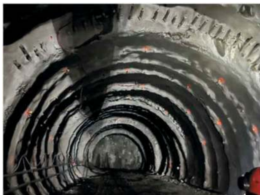
Figure 5. Pipe roofing prior to the installation of double RRS.
