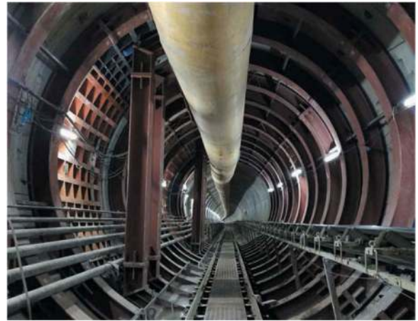
Figure 9. Temporary steel support.
