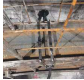
Figure 8. Installing load adjuster.
