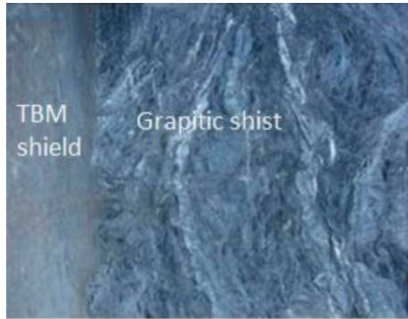
Figure 9. TBM shield and squeezing characteristic graphitic schist.
