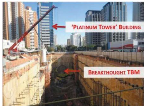
Figure 14. General view of the location with the building and TBM.
