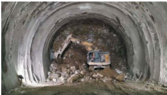
Figure 16. Full face excavation with steel ribs and shot-concrete placed.
