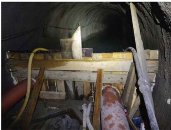
Figure 3. Damming and groundwater pumping. Preparation for reconstruction.
