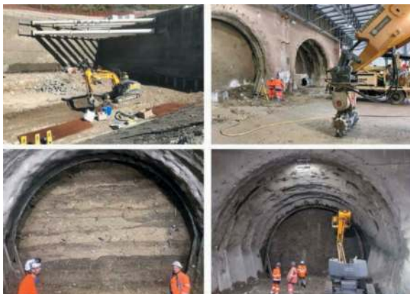
Figure 11. Excavation works in CO8 lot.
