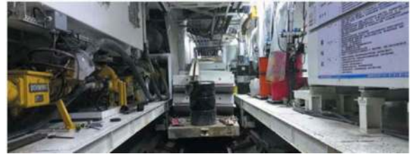
Figure 5. Environment of TBM construction.
