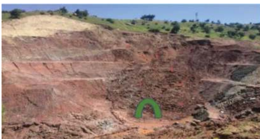
Figure 3. Diversion outlet, in-situ situation on 01.05.2020.
