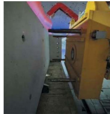
Figure 18. Effect of recognition of the center hole of the Mid-partition by the vision camera.
