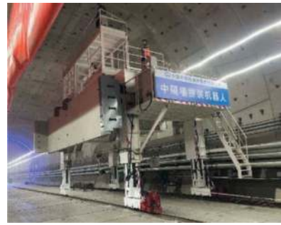
Figure 21. Field application of intelligent assembly robot for Mid-partitions.
