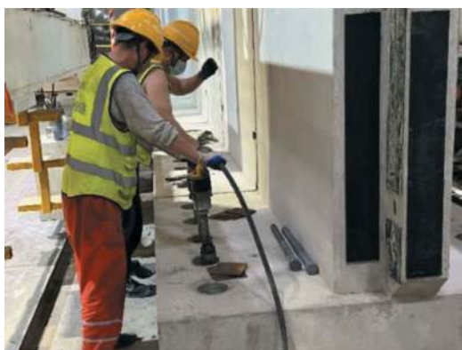
Figure 17. Tightening bolts in the bottom of partition walls.
