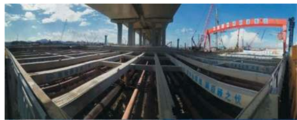
Figure 4. Excavation passing through Guangzhou-Shenzhen Coastal Expressway.
