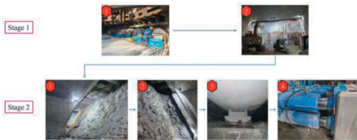
Figure 9. The procedure of the box jacking construction.
