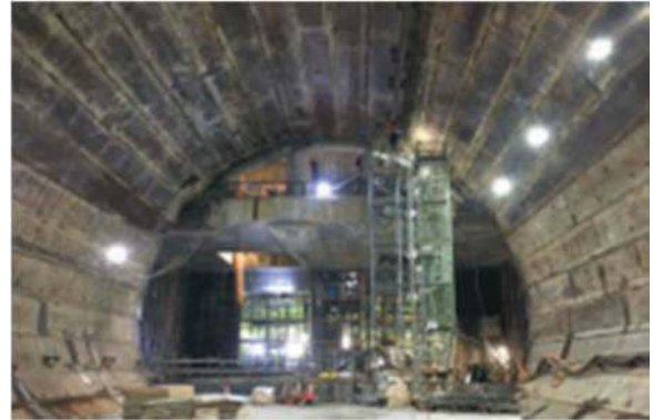
Figure 30. Completion of the internal excavation.
