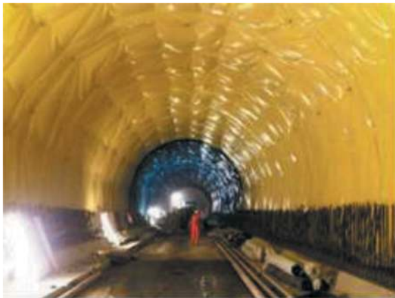
Figure 4. Waterproofing of the dome area for conventional excavation sections.
