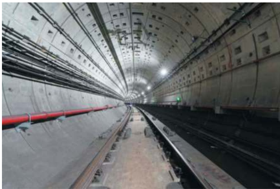
Figure 7. Interior lining of the metro.
