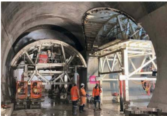
Figure 15. Junction between adits A3 and A4.
