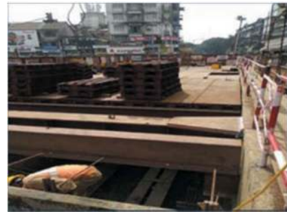
Figure 5. Steel decking installation in progress.
