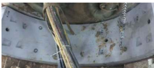
Figure 15. Installation of lower pipe.
