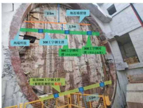
Figure 2. Layout diagram of I-beam support.
