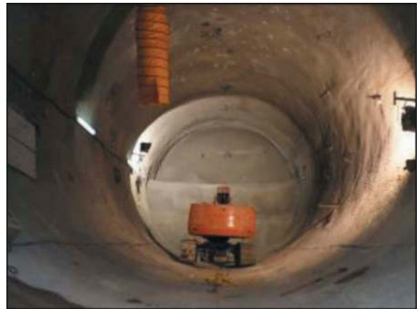
Figure 17. Tunnel excavation on hold prior to F1 race in 2009.
