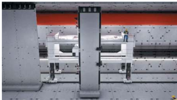
Figure 11. Mid-partition rotating 90° to reach vertical state.
