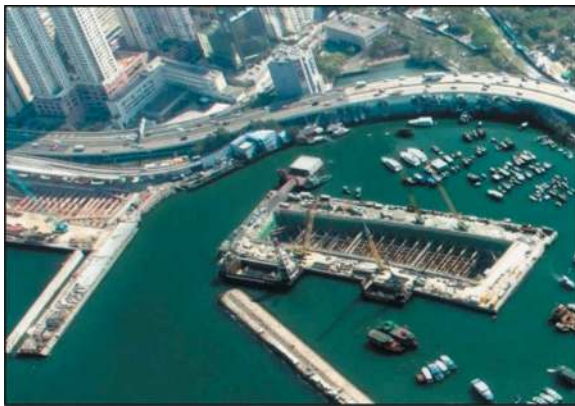
Figure 5. Central - Wan Chai Bypass, Hong Kong, SAR of China.
