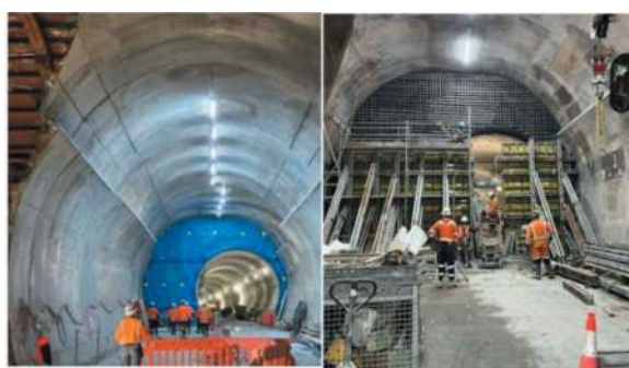
Figure 3. Headwall stitched to secondary lining.
