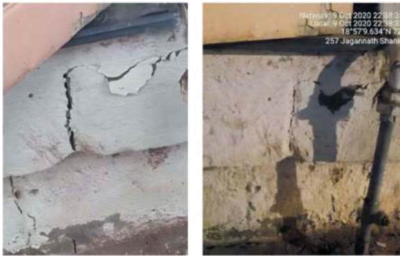
Picture 2a & 2b. Crack-1 prior to and after grouting measures.
