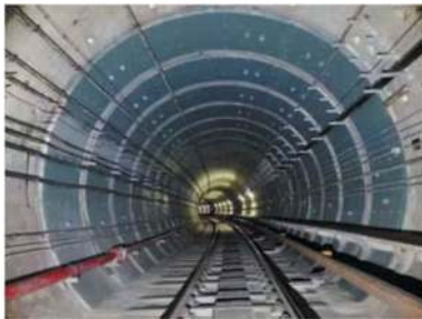
Figure 3. Steel plate bonded with lining inside tunnel.
