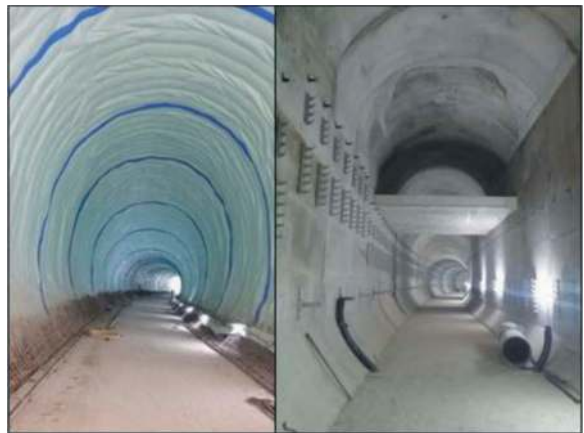
Figure 21. Waterproofing and completed tunnel lining.
