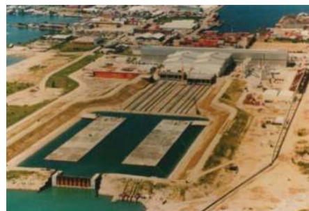
Figure 16. The first industrial tunnel element production facility with 2 production lines.
