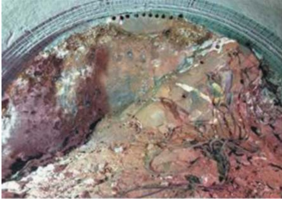
Figure 18. Tunnel face in Fort Canning Boulders Bed.
