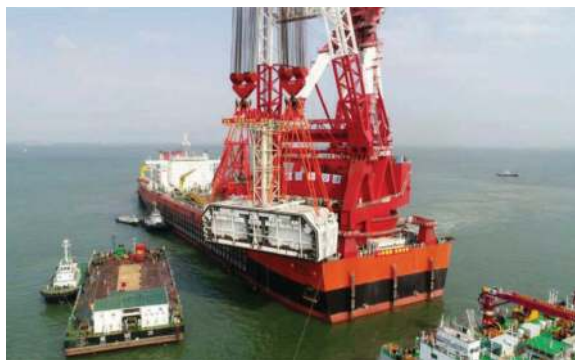
Figure 24. Closure joint installation of HZMB (Su Quanke, et al., 2022).
