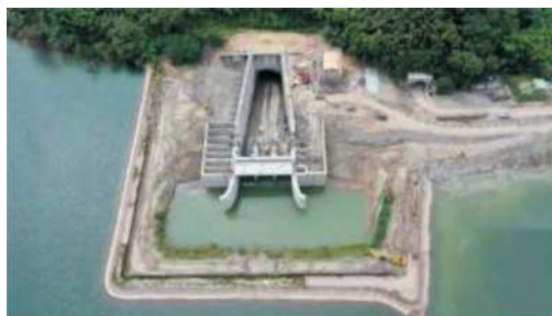
(1) Intake structure and cofferdam (2022.6)
