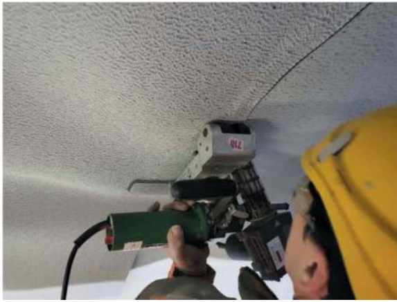
Figure 15. Hot air welding of the membrane.
