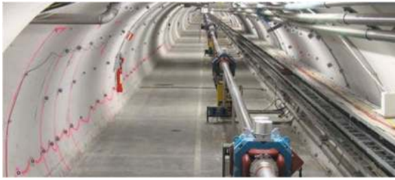
Figure 9. View of TT10 tunnel (Di Murro, 2019).
