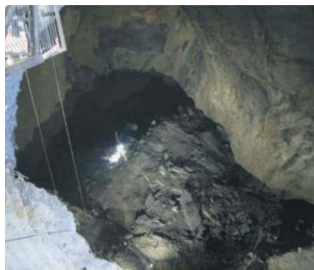
Figure 2. Cave roof wedge.
