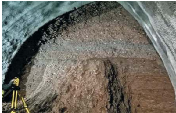
Figure 5. Contact between the 2nd deposit and the 1st deposit units of the Mapocho River alluvial gravels.
