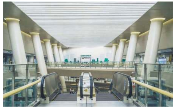
Figure 13. Real view of V-pillar of Huangmugang Hub.
