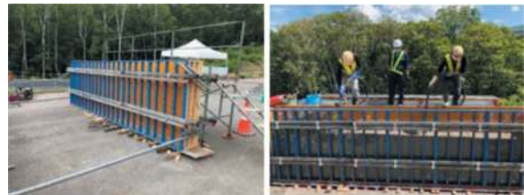
Figure 13. Flowability test (Field).
