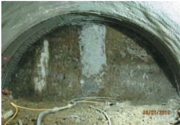
Figure 15. Demolition of CCL tunnel DWall during tunnelling.
