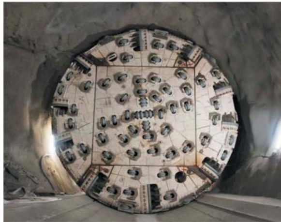
Figure 4. TBM cutter head, construction lot Mules 2-3.
