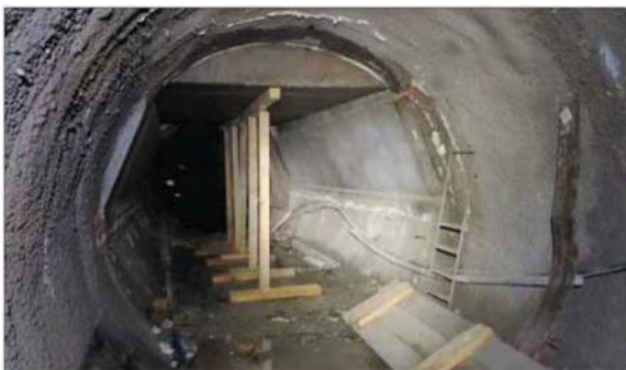
Figure 14. Intersection with cross passage No. 27 – construction phase.
