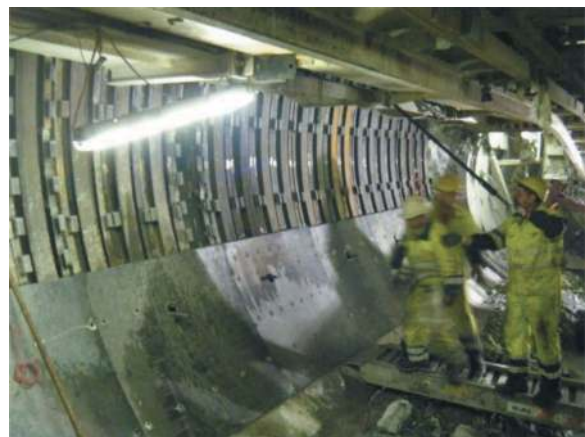
Figure 4. Repaired stretch with steel panels.
