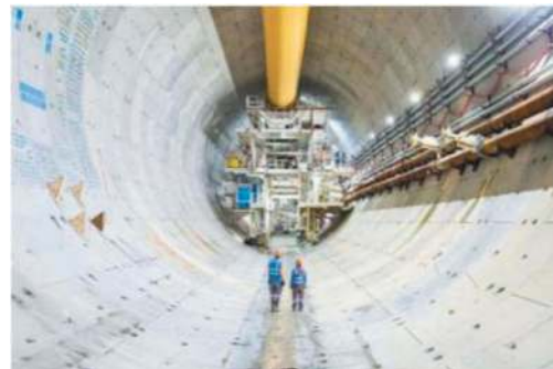
Figure 15. World's largest TBM tunnel.
