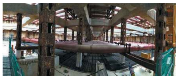
Figure 4. Excavation and support arrangement in cofferdam.
