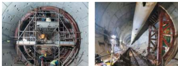
Figure 2. Temporary steel support for tunnel opening (left: Hamster cage Right: Half-moon).
