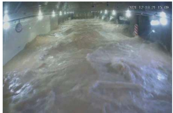
Figure 8. CCTV images of the SMART tunnel after activation (The Star, 22 February 2022).
