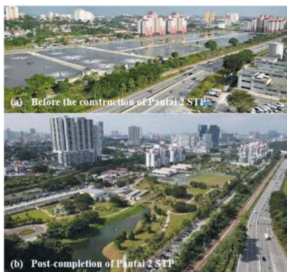
Figure 9. (a) Before the construction of Pantai 2 STP, (b) Post-completion of Pantai 2 STP.
