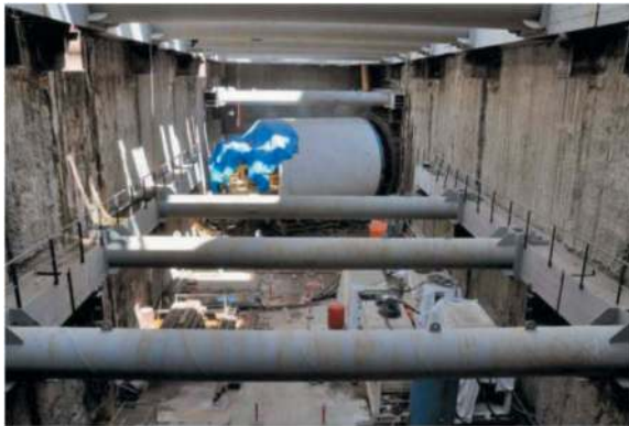
Figure 12. The portal of the tunnel.
