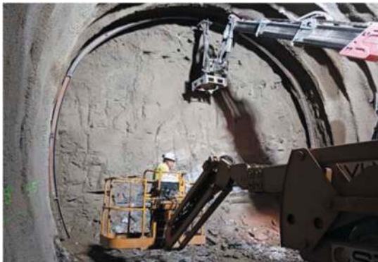
Figure 24. Colocation of HEB 140 profile.
