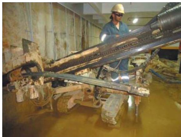
Figure 16. Removal of tie rods' strands.
