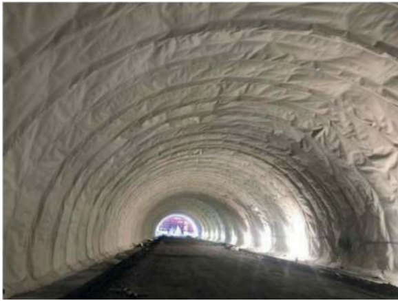
Figure 2. Fully bonded membrane ready for concrete application.
