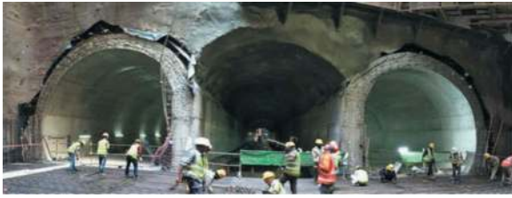
Figure 27. The 3-Arches tunnel in rock during permanent lining.
