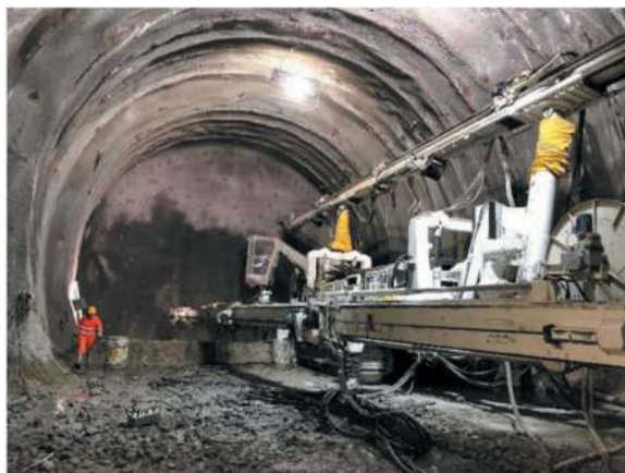
Figure 10. Excavation with QSJG® method.
