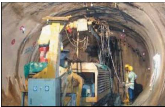
Figure 7. Pipe roof canopy installation.
