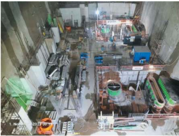
Figure 8. Inner lining works in the machine cavern November 2023.
