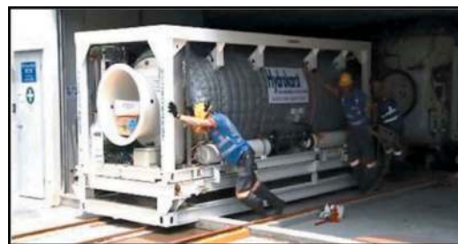
Figure 11. Pressurized shuttle transferred daily to tbm.
