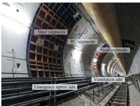
Figure 8. Steel segments for opening.
