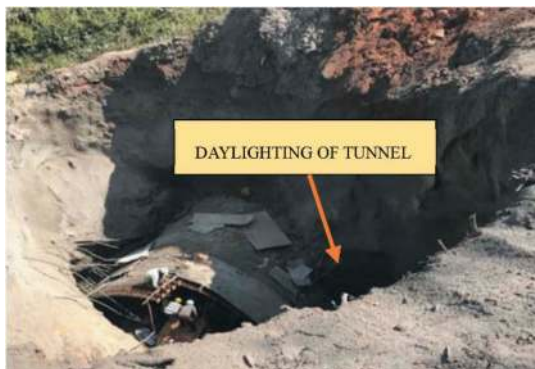
Figure 13. Complete Daylighting of Tunnel b/w Ch:1700 - Ch:1722.
