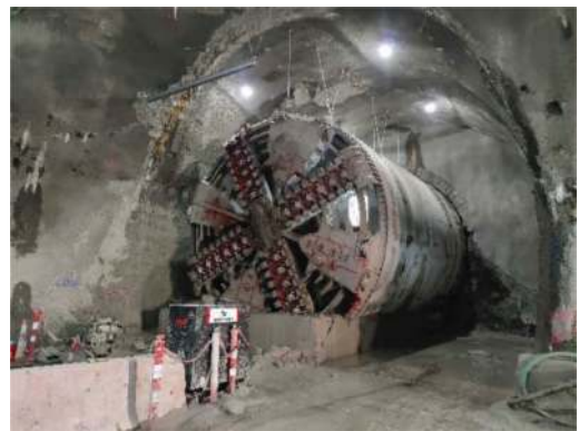
Figure 18. TBM breakthrough at KHP station MC30 cavern.
