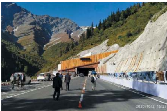
Figure 9. The South Portal of the Atal tunnel, one day prior official opening.
