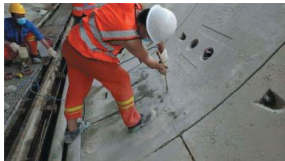
Figure 21. A cracked segment is repaired by injections.
