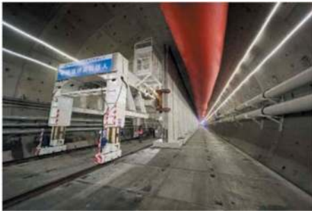
Figure 13. Partition wall assembly robot on-site operation.
