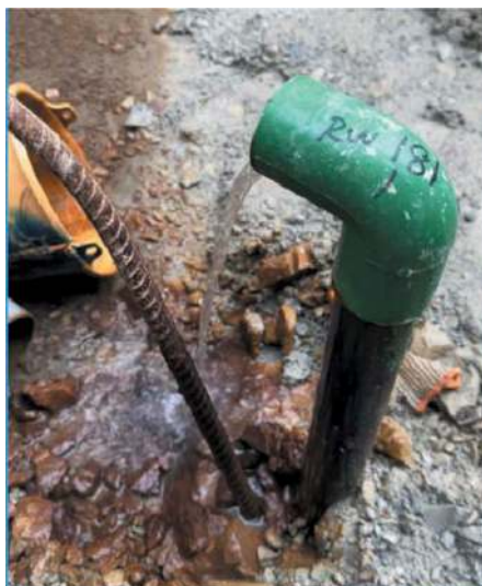
Figure 13. Outflow from relief well.
