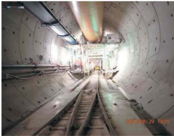
Figure 5. Tubbing ring lining in construction lot H41.
