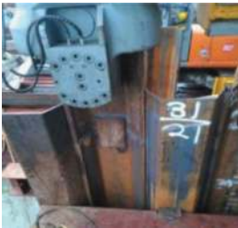
Figure 9. Hydrostatic pressing pile planting.
