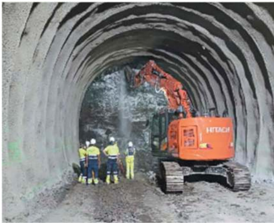
Figure 22. Excavation the complete section.
