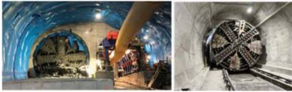
Figures 20 & 21. TBM breakthrough in MC20/MC30 cavern (left) & TBM crossing Karanga-a-Hape (right).
