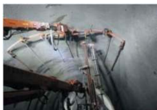
Figure 7. Mechanized Construction of Anchor Mesh Support.
