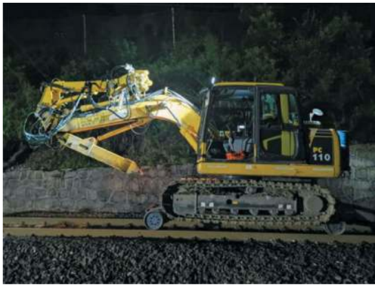
Figure 9. Road-rail transport platform.
