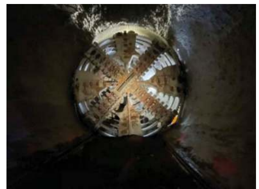
Figure 19. TBM in the KHP MC30 mined stub tunnel.
