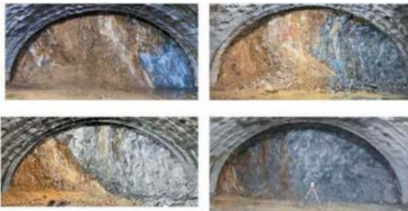
Figure 6. Mixed faces with different aspects, in the same tunnel and same week. Source: Authors.
