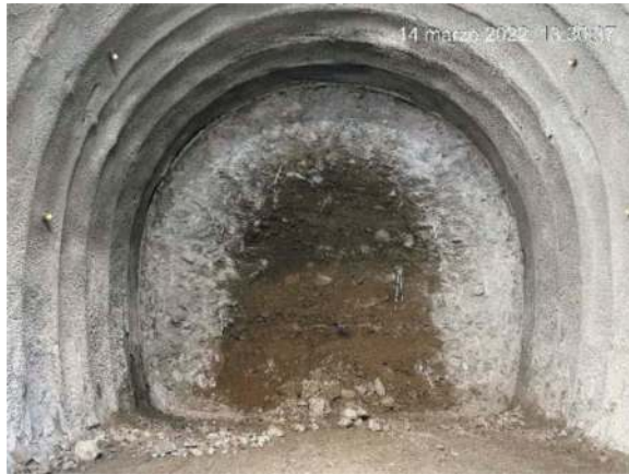
Figure 15. Band of frozen soil within the excavation profile.
