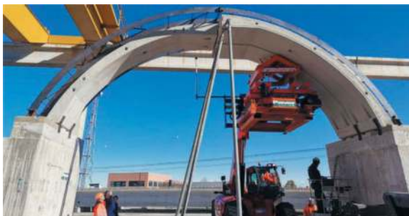
Figure 16. “Poderuzzo” tunnel - Field test of pre-cast concrete shell implementation.
