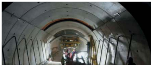
Figure 10. “Colle Marino” tunnel construction site – relining by high strength shotcrete.
