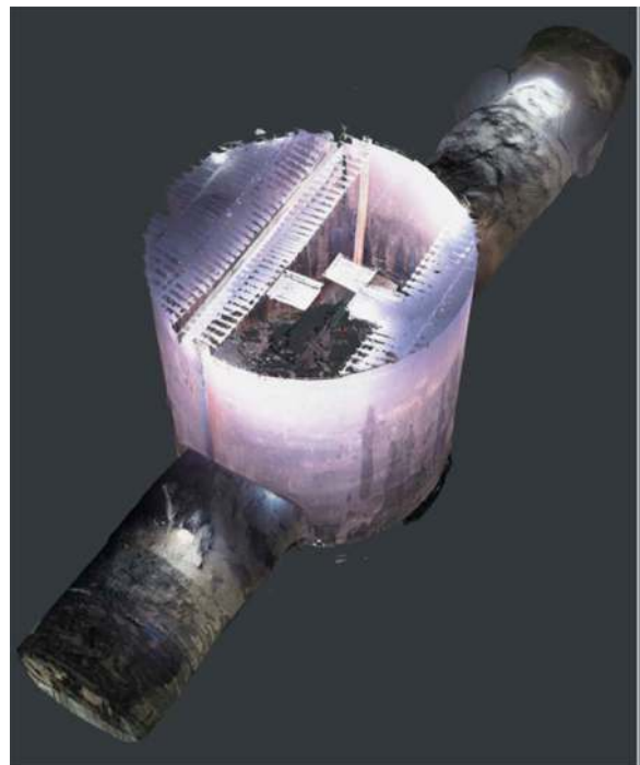
Figure 3. João Paulo I station points cloud.
