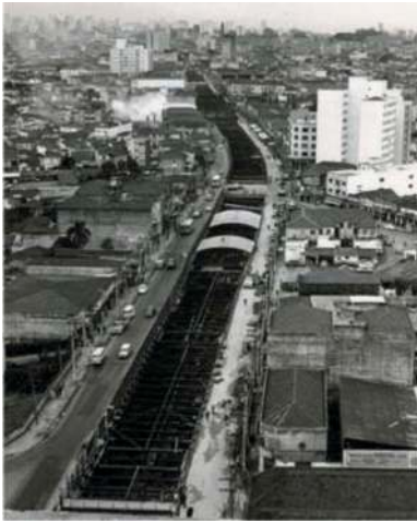
Figure 1. Cut & Cover in the south of the city - Line 1 - 1970s.(Metrô-SP).
