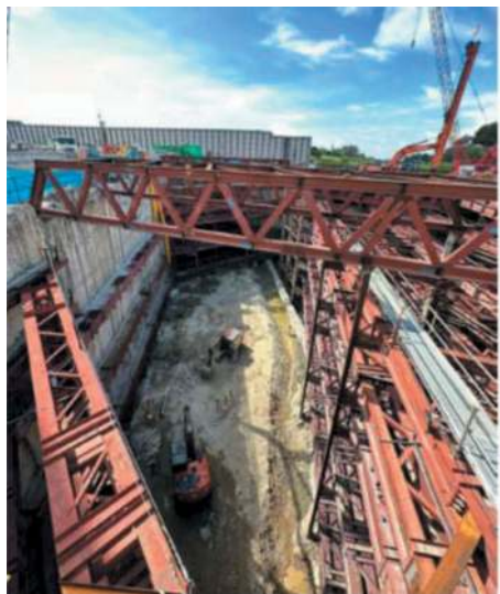
Figure 7. Strus and truss.
