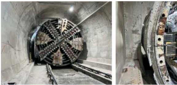
Figure 12. TBM Transition in KHP MC20 mined tunnel.
