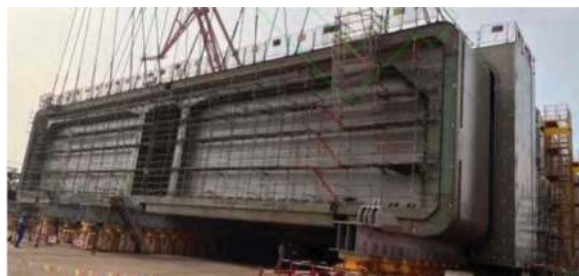
Figure 26. Closure joint of Shen-Zhong Link (DENG Bin, et al, 2023).
