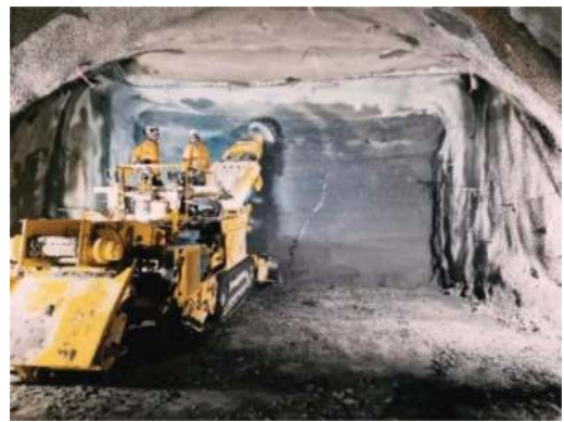
Figure 17. Excavation at KHP Adit A1.
