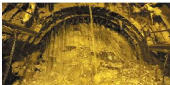
Figure 13. Very Large groundwater inflows.
