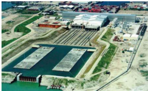
Figure 7. Øresund Tunnel casting factory.
