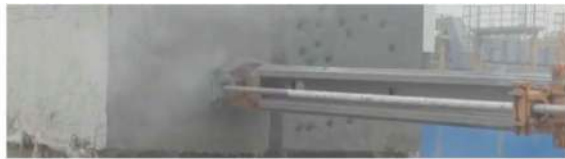
a Borehole test process-drilling for 0.1m
