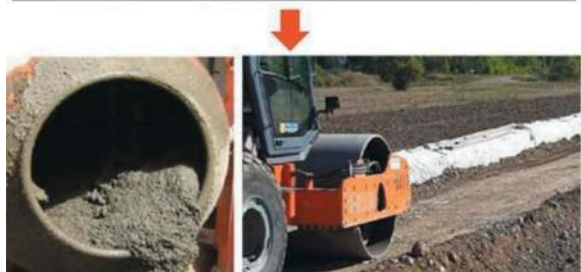
Figure 4. Reuse of excavated soil and rock.
