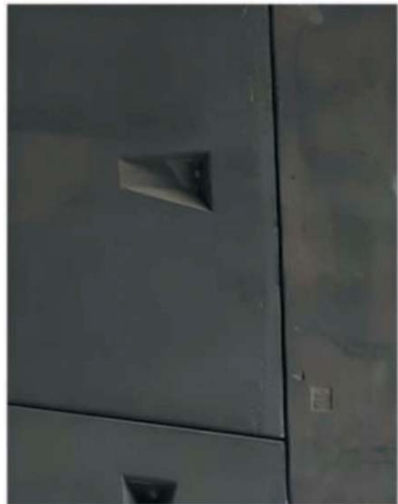
Figure 7. Radial and longitudinal joints for segment edges.
