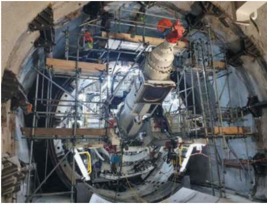
Figure 11. Temporary launching frame in MC30 drive.
