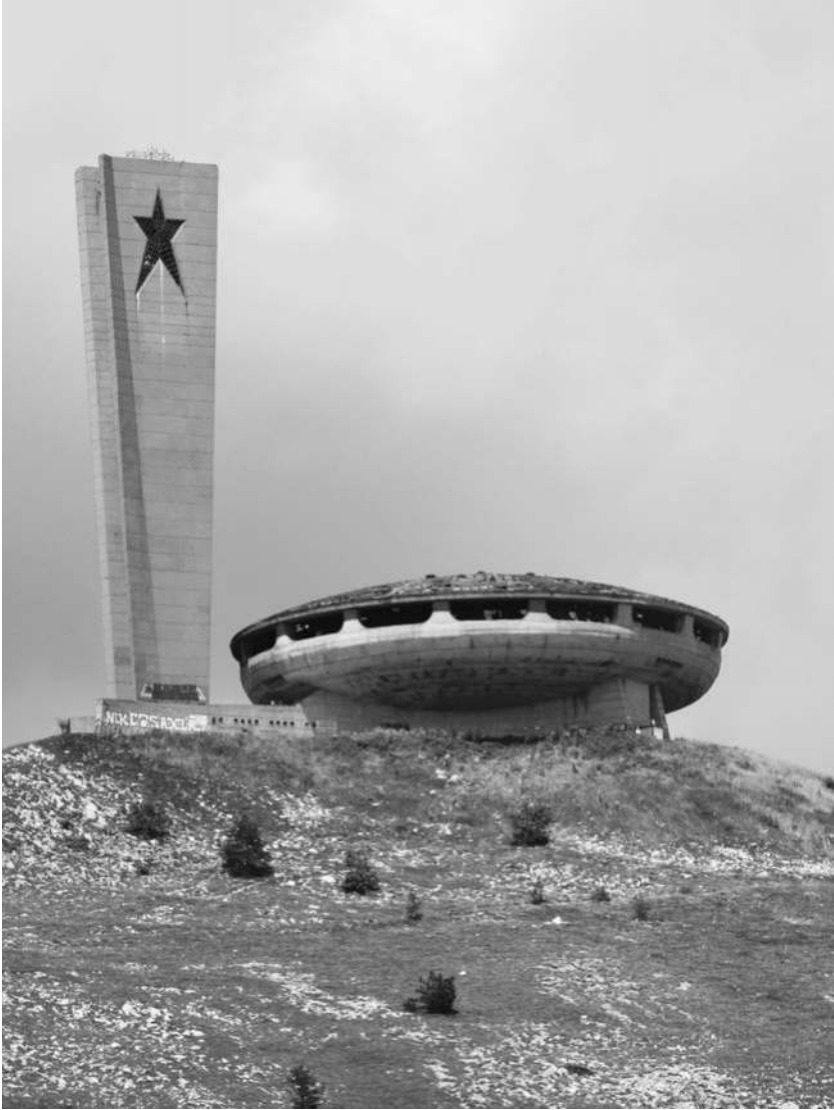
FIGURE 40. The Home Monument of the Party on Buzludzha in summer 2019. The graffiti, damaged ceiling, and missing red star are visible even from a distance. Photo by author.
