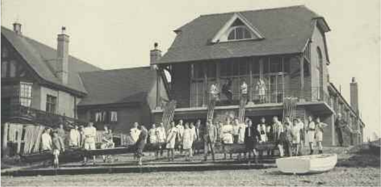
Fig. 87 The Polytechnic Boathouse was to suffer significant bomb damage during the Second World War and the boats were destroyed by fire.
