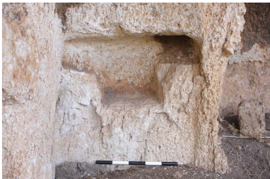
Figure 5.4: ‘T’ shaped beam socket JNN-U1 with slot carved at the upper end of the niche. Scale 0.5 m.
