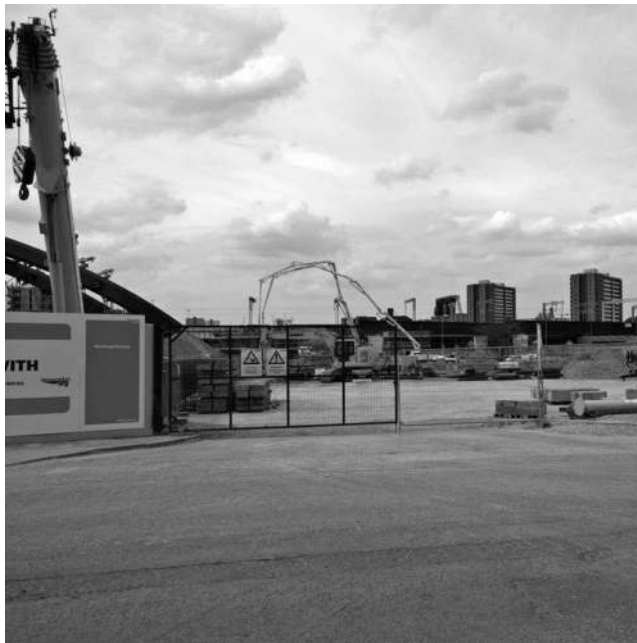
Figure 29.1 Factory, OMA – building site in Manchester (Authors' Own)
