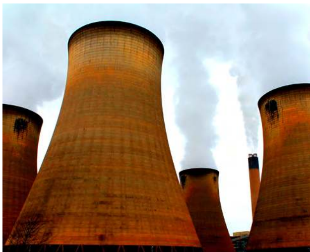
Figure 12.24 Cooling towers at the Drax power station in North Yorkshire, United Kingdom (credit: Les Haines, Flickr)
