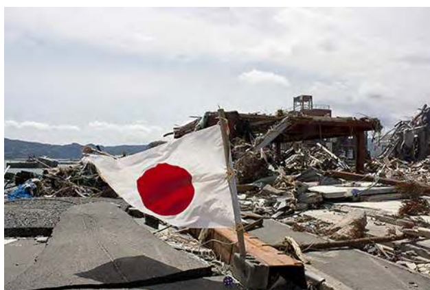
Figure 6.21 Devastation of March 11, 2011 earthquake in Honshu, Japan. (credit: Daniel Pierce)
