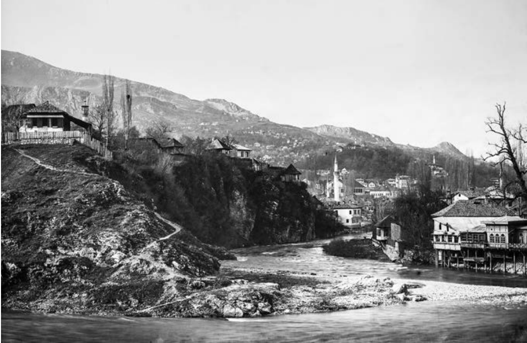
Figure 1.13. Sarajevo seen from the bend of the Miljačka River, 1910.
