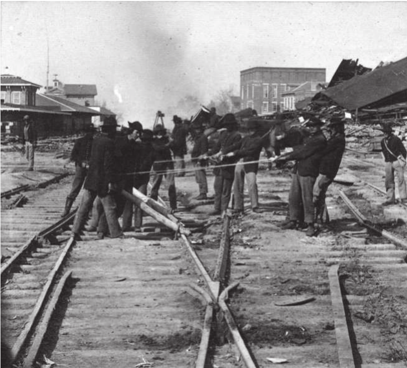
FIG. 3. Regiment of Michigan engineers and mechanics destroying railroad tracks in Atlanta, from a stereograph by George N. Barnard. ( Library of Congress Prints and Photographs Division )
