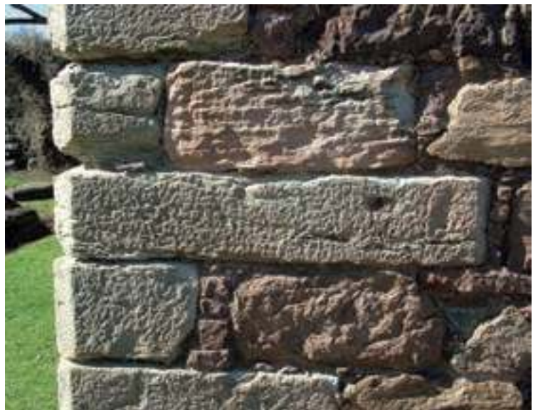
Fig. 4.38: Detail of reused pier sections showing tooling
