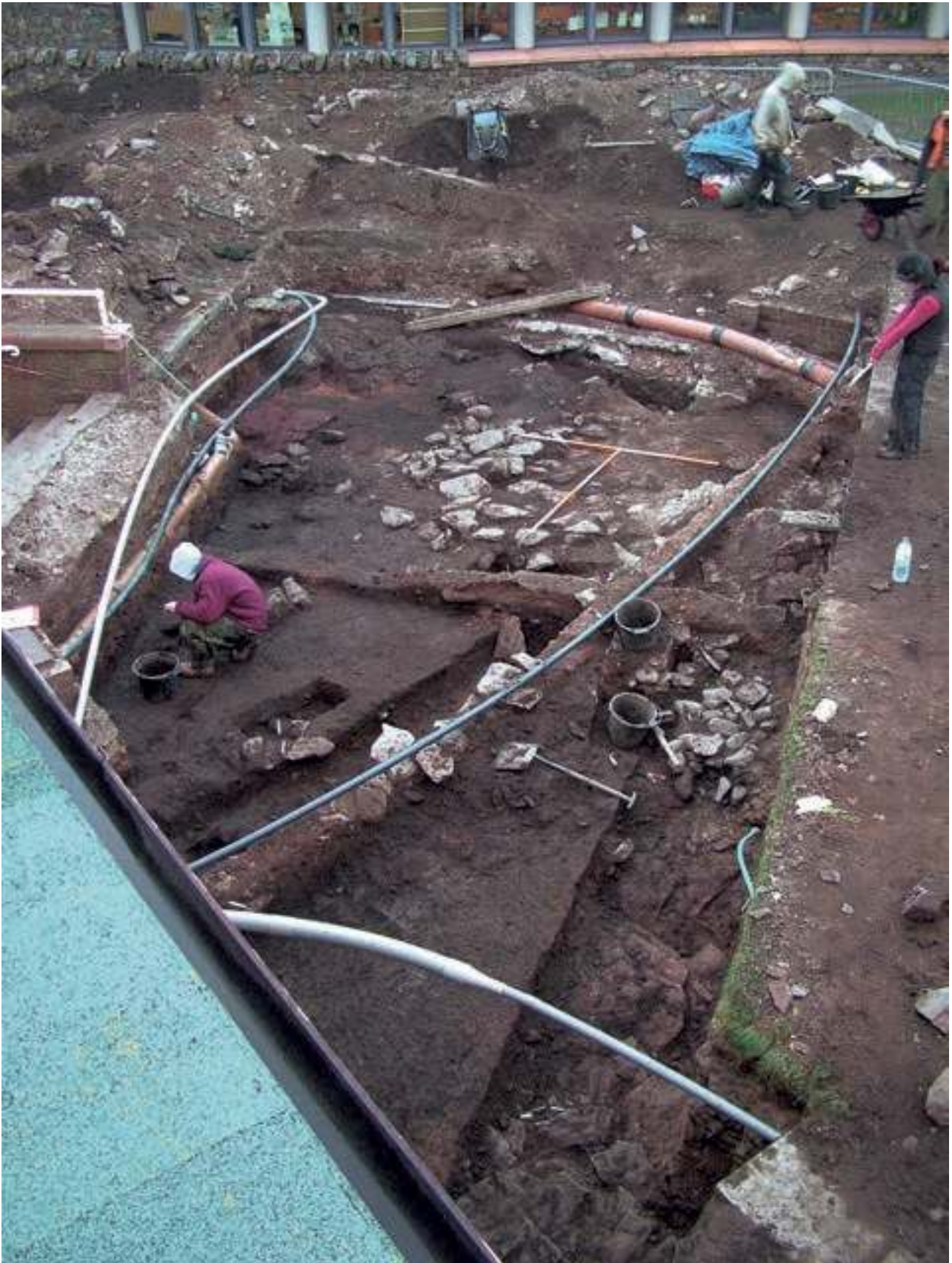
Fig. 1.13: General view of the tunnel area excavation in progress: working shot, looking E
