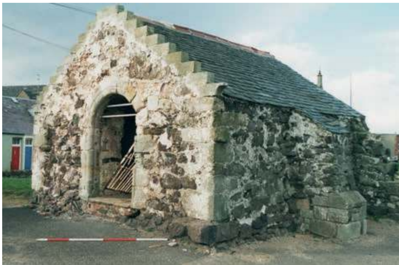
Fig. 4.32: View of the south porch from the SE taken in 2000, before commencement of repair works
