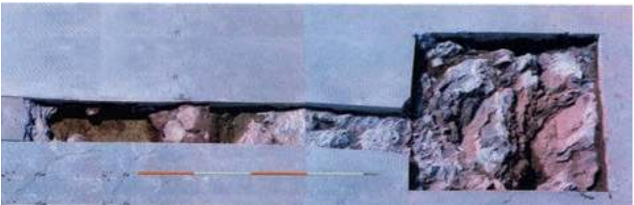
Fig. 1.7: Northern part of the services trench to the NW of the Scottish Seabird Centre site, bedrock revealed, looking SW
