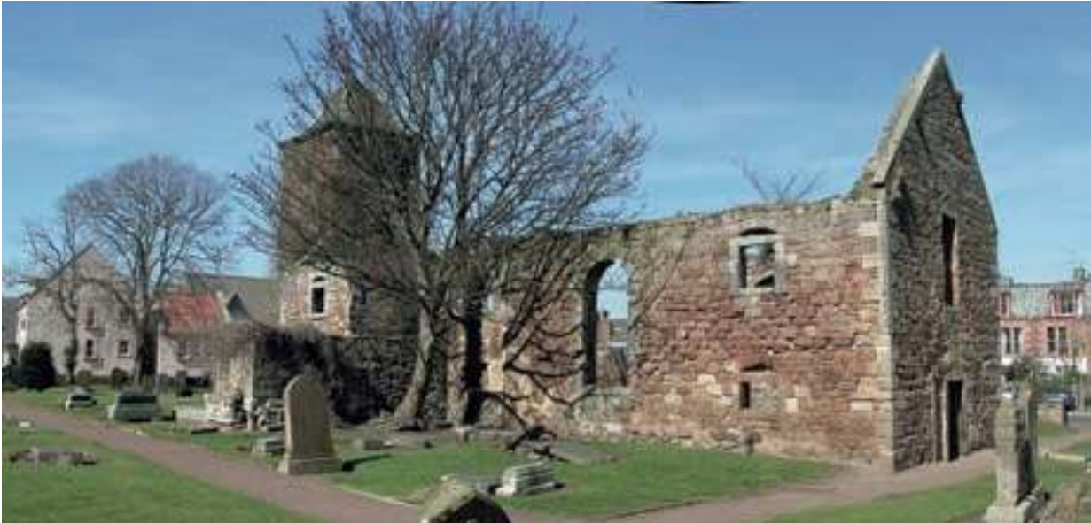
Fig. 4.36: The church of St Andrew, Kirk Ports, erected c.1658–64; view from the SE
