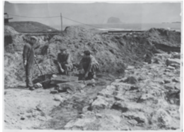
Fig. 4.18: General view of the 1951 excavation in progress, with Dr J. S. Richardson crouched, centre following the discovery of the red sandstone table tomb close to the junction of the west tower and nave, looking ENE (Courtesy of East Lothian Council Archives & Local History Service)
