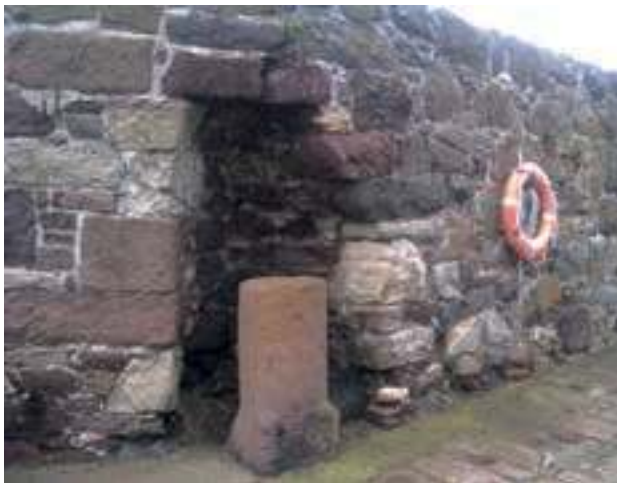
Fig. 4.41: Part of the northwest-facing harbour breakwater; interior face, showing an assortment of reused stones likely recovered from the medieval church site
