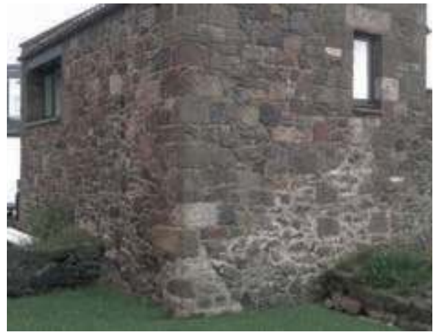
Fig. 4.42: The south and east walls of Church Cottage contain reused stonework from the church
