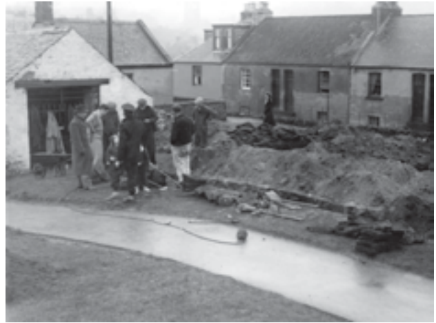
Fig. 4.16: The test trenching operation nearing completion, looking SW (courtesy of Mrs Lorna Burton)
