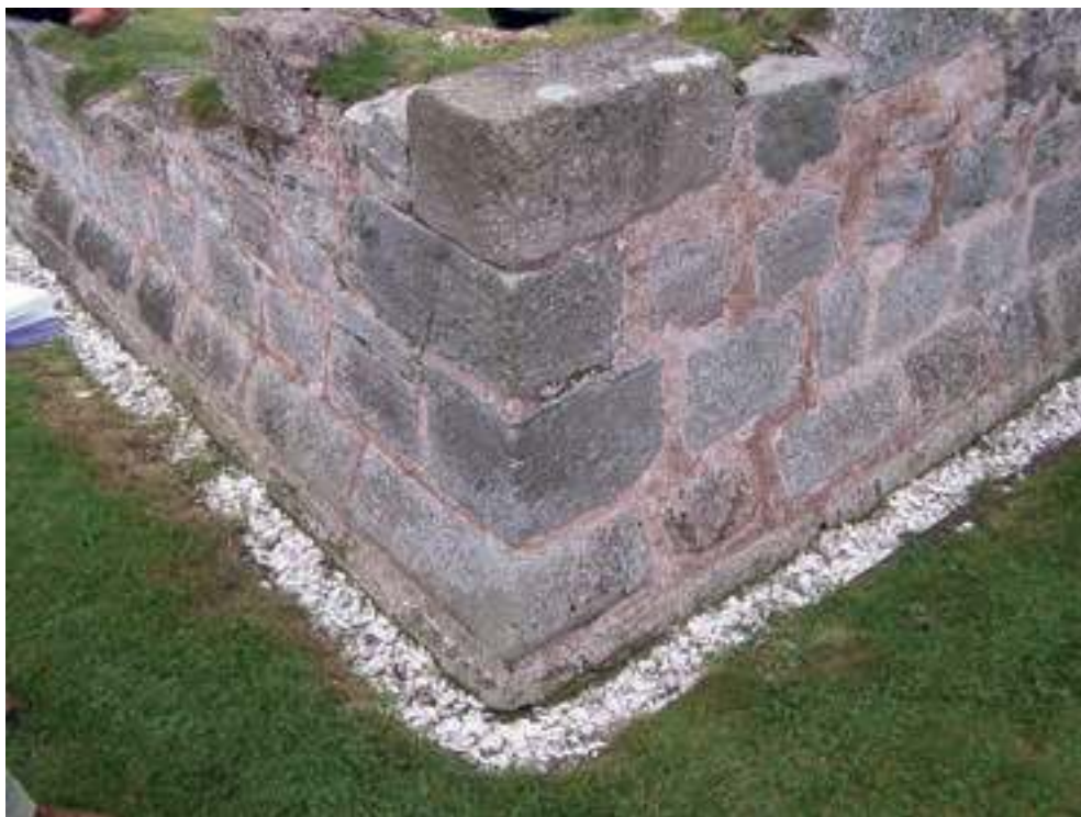
Fig. 4.23: The upstanding NW corner of the north transept, looking SE
