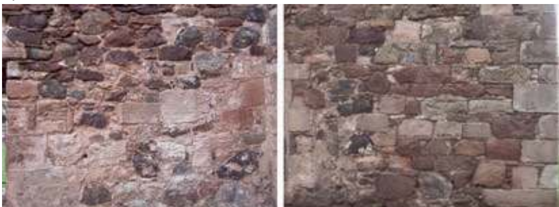
Fig. 4.39: Much of the general lower walling of the 17th century church, contains reused stonework, this demonstrably from the Old Kirk
