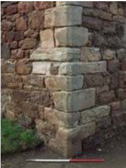
Fig. 4.37: Pier sections from the old church employed as quoins in the church of 1659–64
