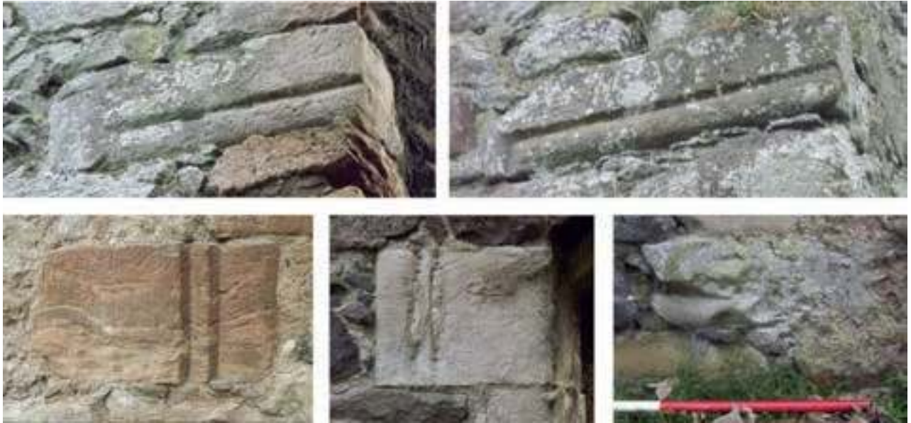
Fig. 4.40: Individual stones displaying moulded detail: lintels with quirked rolls (above), and jamb stones with twice-quirked angle rolls, and part of a pier base, inverted (lower right)
