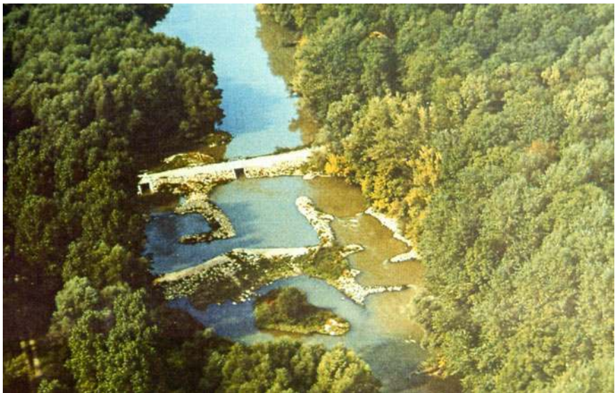
Fig. 24.4 Lateral connection of Korneuburger Au with the main channel of the Danube via a fish bypass system (courtesy of Verbund AG)
