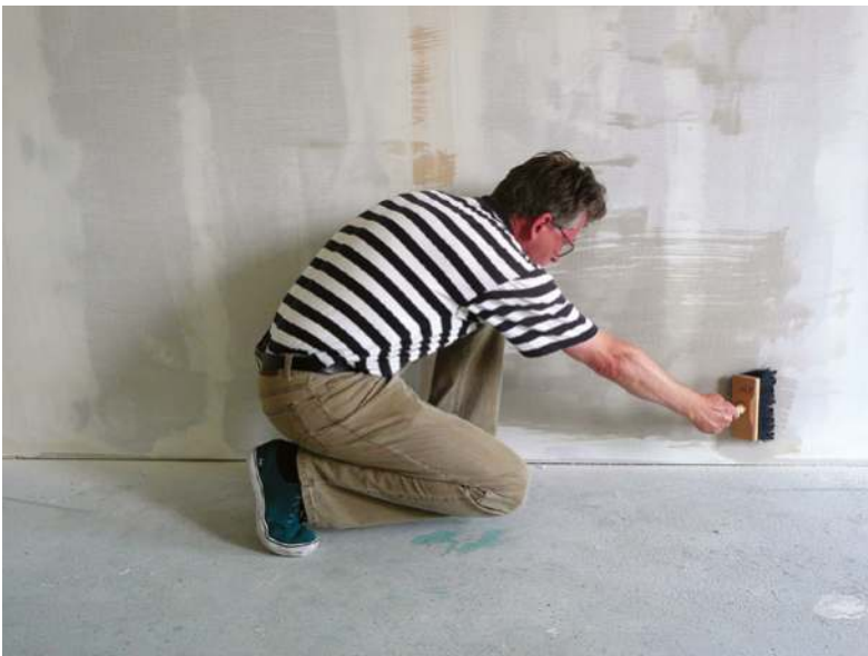
FIGURE 5.4 Intervention A. Work in progress.
