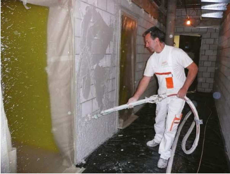
FIGURE 5.5 Intervention A. Work in progress.
