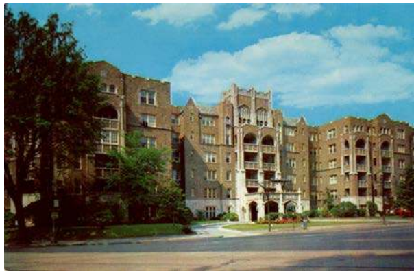
Fig. 3.13 Postcard depicting Alban Towers, Washington, DC (Yonkers, NY: Herbert C. Kahn Studios).
