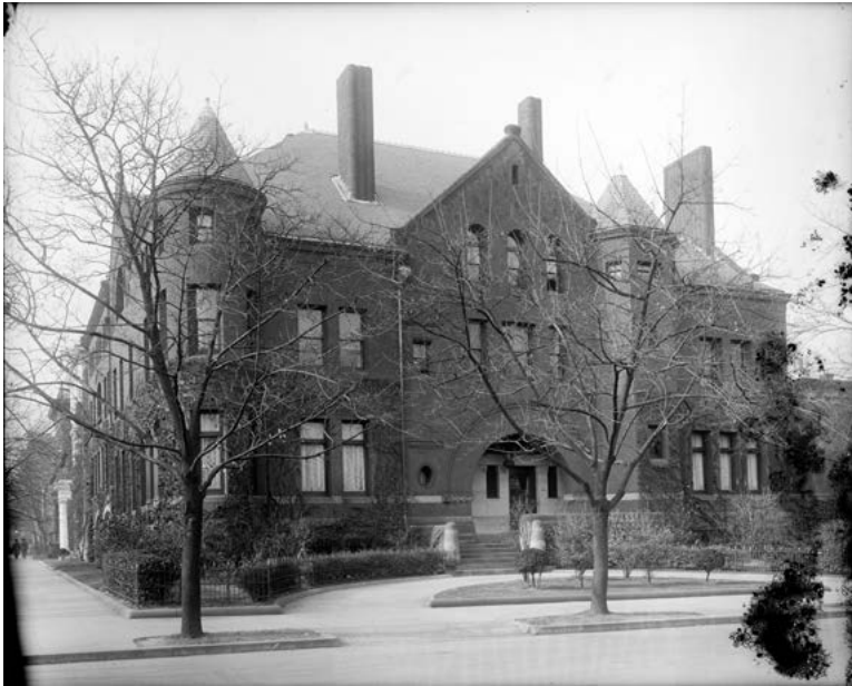
Fig. 3.25 John Hay House, Washington, DC. Photograph by Harris & Ewing, ca. 1910–1920. Washington, DC, Library of Congress, Prints and Photographs Division.
