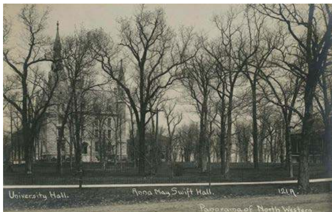
Fig. 5.25 Postcard depicting University Hall, Northwestern University, Evanston, IL (Chicago: The J. O. Stoll Co., early twentieth century).
