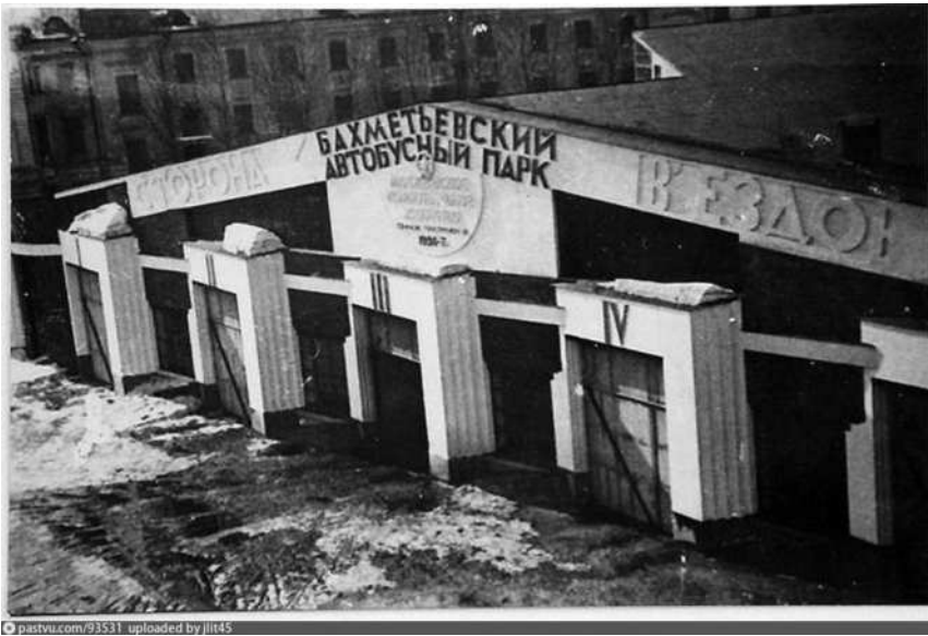
Figure 4 The Bakhmetevskii bus depot, before reconstruction.
