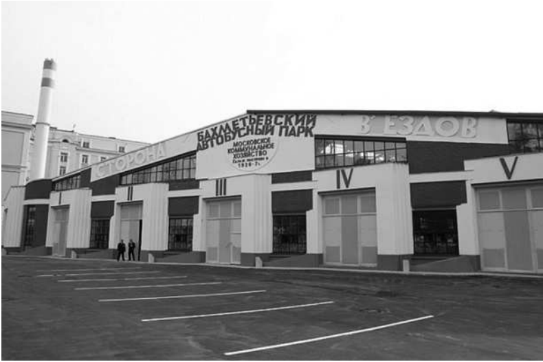
Figure 6 The Bakhmetevskii bus depot, after reconstruction.
