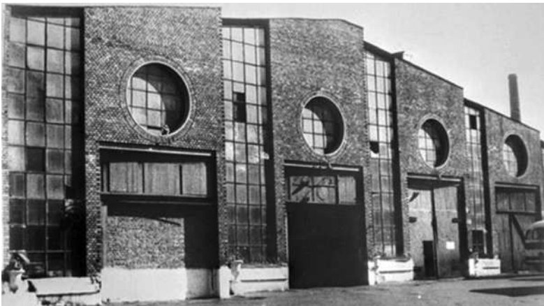
Figure 5 The Bakhmetevskii bus depot, before reconstruction.
