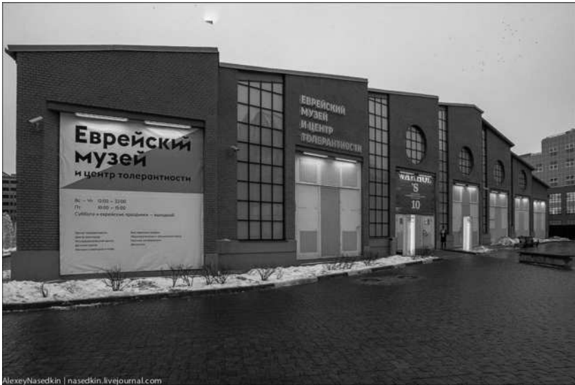
Figure 7 The Bakhmetevskii bus depot, after reconstruction.
