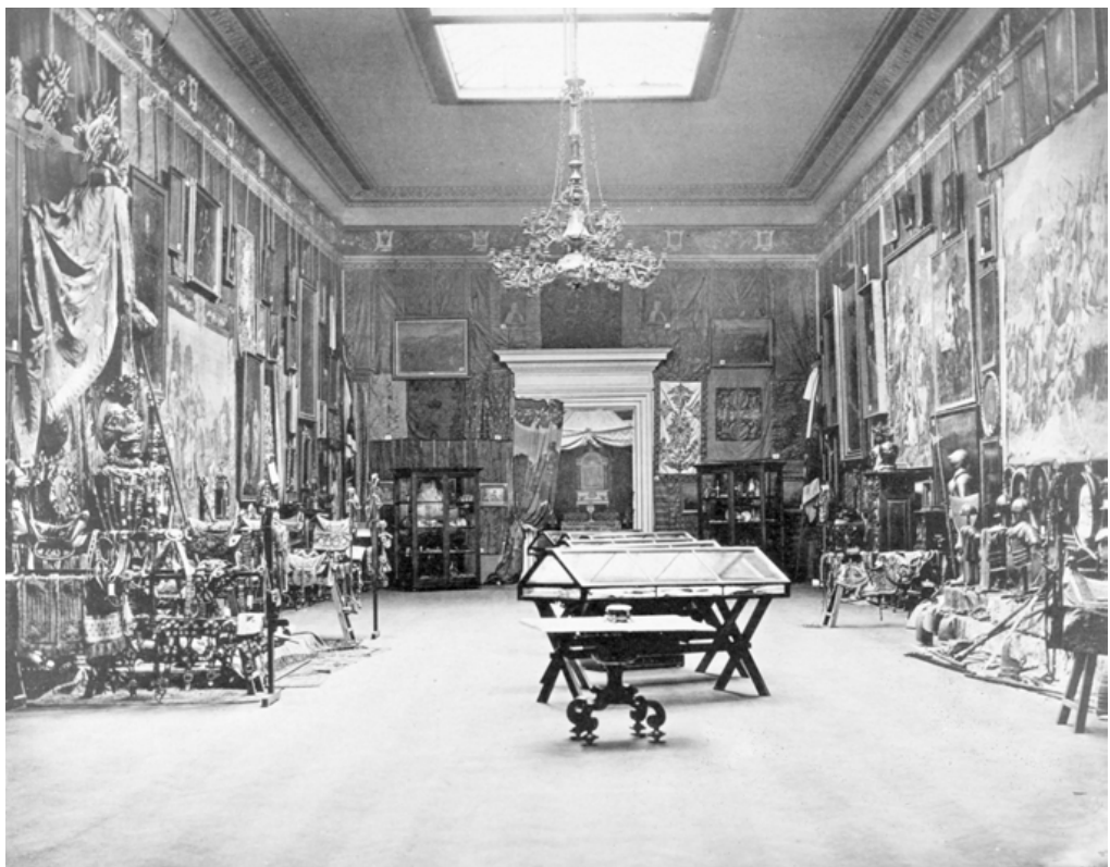
Fig. 4: View of the main hall of the Jubilee Exhibition of King Jan III in Krakow.
