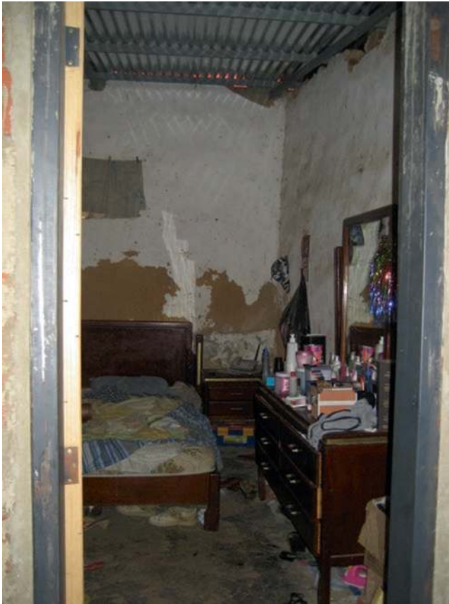
Photo 9.3 New roof acquired through a communal council project. Photo by the author
