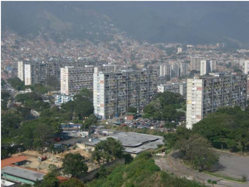
Photo 1.2 Some of the famous superbloques (apartment buildings) of 23 de Enero with the barrio la Pastora and the mountain ridge Ávila in the background. Photo by the author
