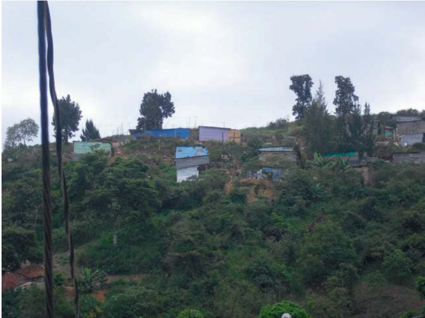
Photo 9.1 Ranchos in Casaalta 4, according to local residents built in unstable soil. Photo by the author
