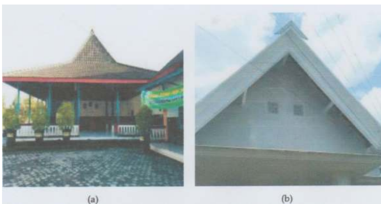
Figure 8. The changes of residential model around mount Kelud. (a) Joglo-shaped roof commonly called the “Tuo” building form and (b) the roof of a cone-shaped house is commonly called the “Enom.”.
