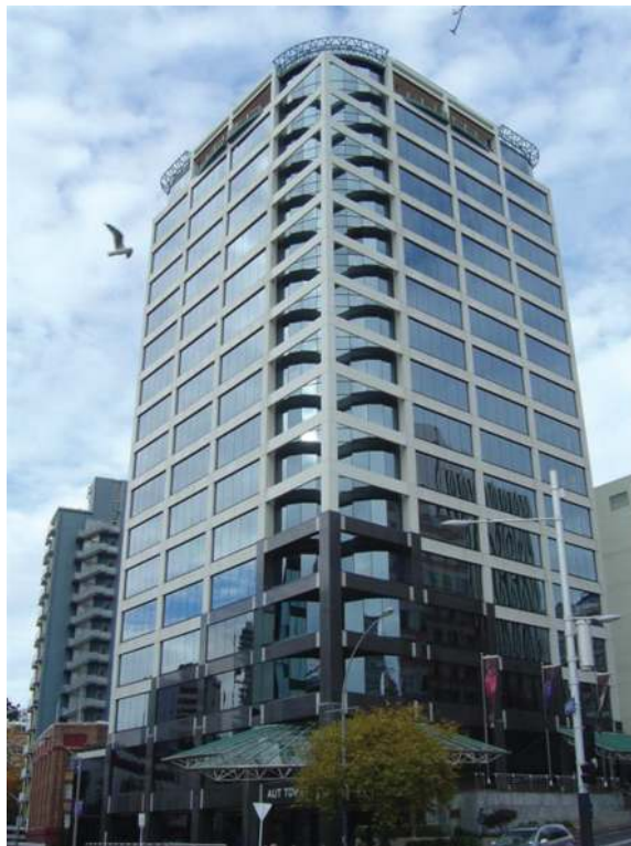
FIGURE 7.6 External view of Environment B (AUT tower).
