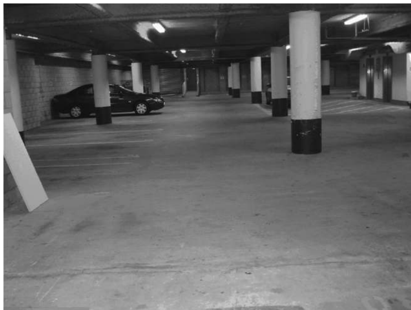
FIGURE 7.5 (SEE COLOR INSERT.) Internal view of Environment A basement parking lot.
