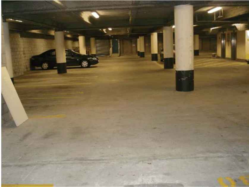
FIGURE 7.5 Internal view of Environment A basement parking lot.
