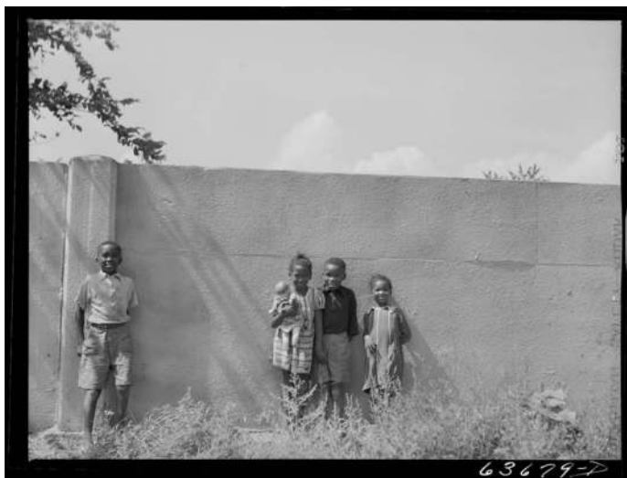
Figure 2.2 “The Wall,” Detroit, 1941. A half-mile long concrete wall was constructed along Detroit’s outer boundary. The wall was built in an effort to keep African Americans from Detroit out of a suburban area where new housing for whites was being developed just outside the city border. Interestingly, government housing finance agencies, and not just private investors, insisted on the construction of the wall to promote the marketability and stability of the new housing.
