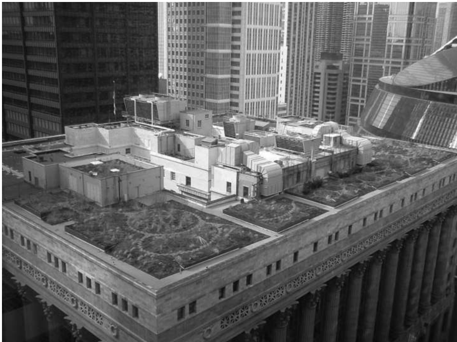
Figure 12.4 Green Roof Atop Chicago City Hall.
