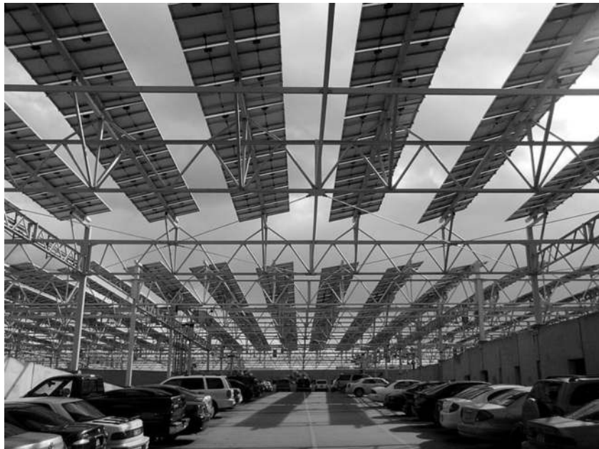
Figure 12.3 Solar Panels on Car Parking Lot, Arizona State University. Green building construction codes can encourage the utilization of renewable energy, such as the construction of photovoltaic cells over a parking lot.
