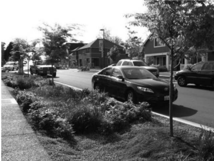
Figure 12.7 Green Streetside Swale, Seattle. By allowing for the capture of water runoff from abutting sidewalks and roadways, this low-lying green swale allows for natural on-site filtration of rainwater, minimizing the pollution of streams and rivers that result from underground piping and drainage of storm water that contains roadway contaminants.
