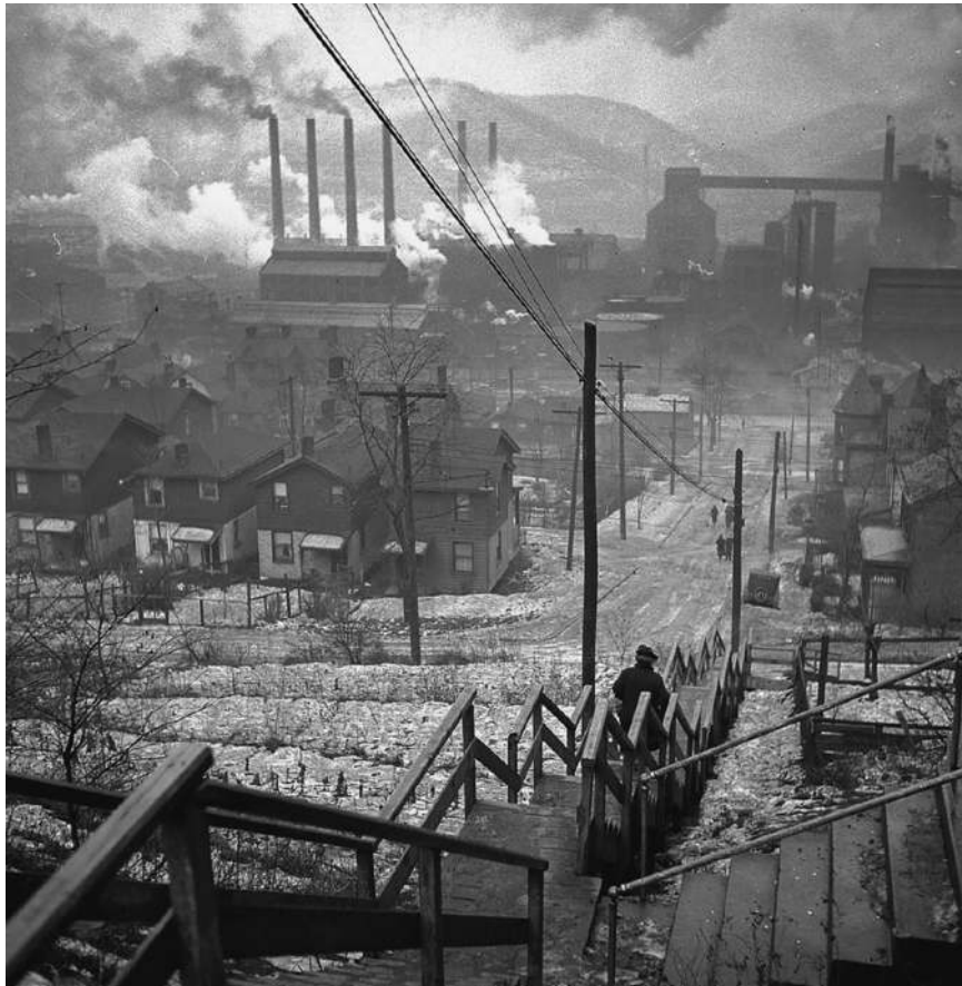
Figure 1.2(a) The Industrial City: Steel Mills and the South Slopes Neighborhood of Pittsburgh, 1940.
