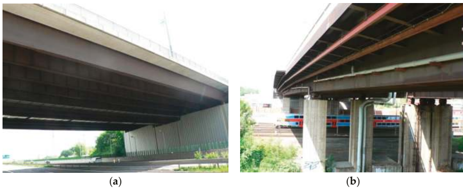
Figure 3. View at selected bridges for experimental testing: (a) Bridge No. 1 and (b) bridge No. 2.
