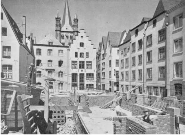
Figure 9: Cologne, rehabilitation works at the Eisenmarkt square, 1938
