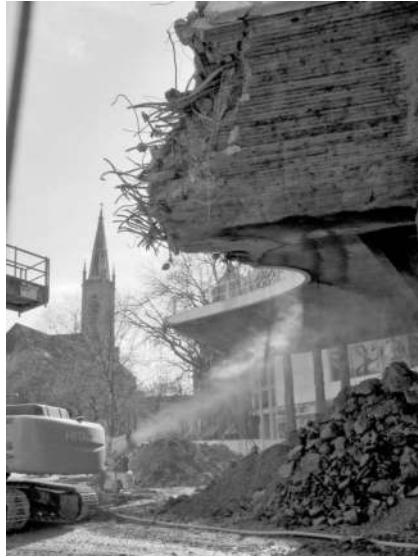
Figure 9: Düsseldorf, Demolition of the 'Millipede' next to St. John's Church (Photo: Perlgrau 2013)
