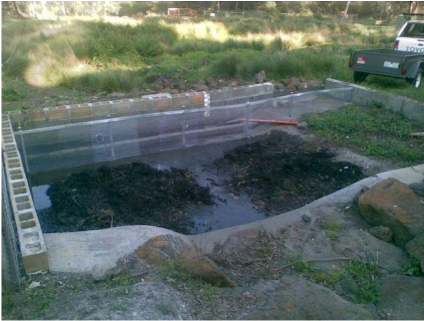
Figure 4.5 Example of primary treatment constructed to reduce blockage of downstream monitored pipes and diversion weir. In this case, the litter fence required monthly-cleaning to maintain satisfactory operation. Source: Peter Poelsma (University of Melbourne).
