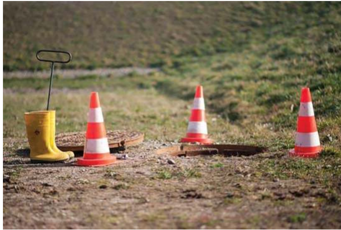
Figure 7.1 Some of the safety equipment required to enter UDSM systems. Source: courtesy of Robert Lohse Photography (2014).
