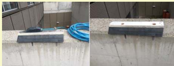
Figure 7.19 Elevated base for in situ wedge sensors. Source: Jakob Benisch (TU Dresden).
