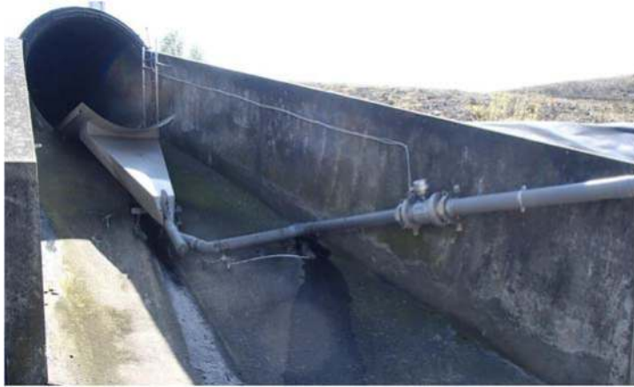
Figure 6.14 Photo of the leaping weir in Chassieu, France. Source: Nicolas Walcker (INSA Lyon).
