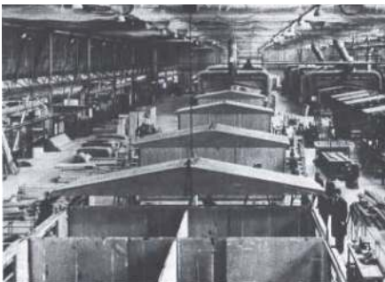
FIG. 25 Aluminium Bungalow, assembly line production, 1947 [source: Herbert, 1984]
