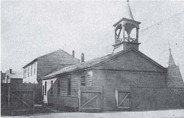
FIG. 09 St. Mary's Catholic Church, built in 1833 with the balloon frame system. (source: Chicago Historical Society, ICHI-37096)
