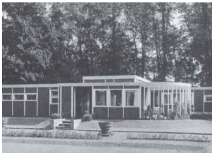
FIG. 16 Hans Scharoun, Berlin, 1927: Single family house in panel construction (made from Christoph & Unmack panels. [source: Junghanns 1994, p. 159]
