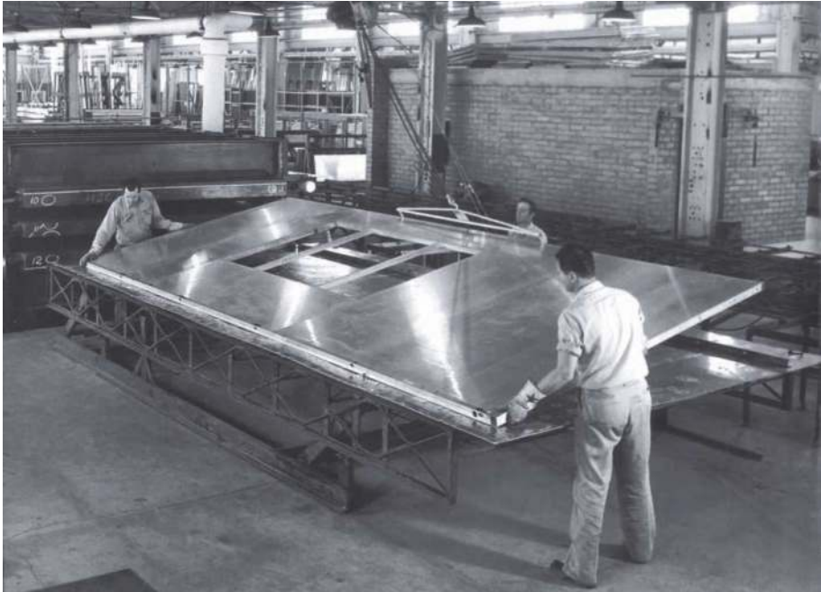
FIG. 24 Aluminium Panels with paper core being constructed at the re-purposed Vultex Aircraft factory in southern California in 1946. [source: Arieff, 2002, photographer Julius Shulman]
