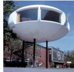
FIG. 30 The Rondo house on exhibition in Basel. [source: Casoni & Casoni architects]
