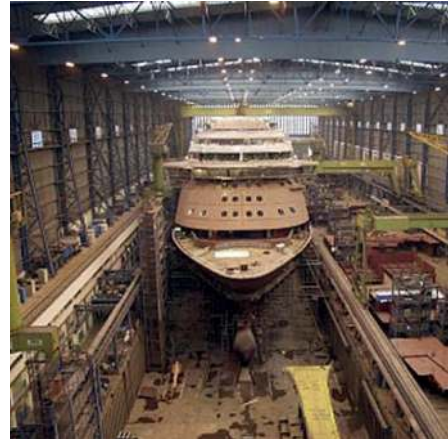
FIG. 70 The whole final assembly of the ship takes place in the main building berth. [source: www.meyerwerft.de]
