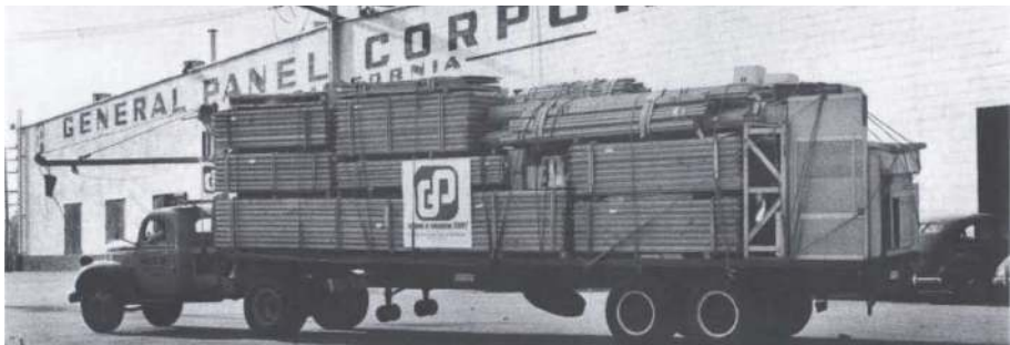
FIG. 19 General Panel, California, components being shipped by truck from factory, c. 1947 [source: Ludwig, 1998]
