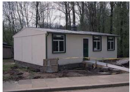
FIG. 26 A Type B2 aluminium bungalow, built in 1947, now re-erected and displayed at the Museum of Welsh Life, St Fagans. [source: National Museum of Wales]
