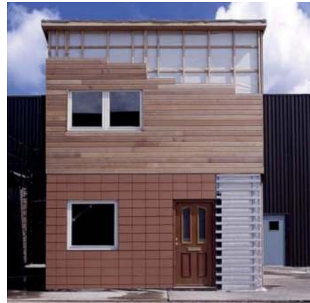
FIG. 114 A prototype built at the factory demonstrate different elevation options. [source: www.optimahomes.co.uk ]
