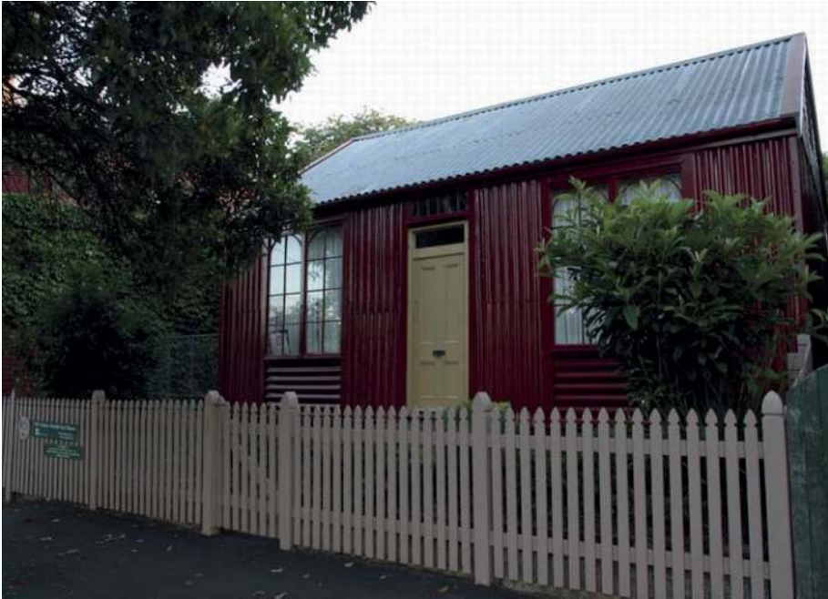
FIG. 06 The Portable Iron House was imported and erected in 1853-54 for local speculator Robert Patterson is still located on the original site, fronting 399 Coventry Street South Melbourne. The portable iron structure, of utilitarian design and unknown manufacture, is constructed of a tee and angle section wrought iron frame clad with five inch pitch corrugated sheet, which is partitioned and lined internally with horizontal boards to form an attic cottage of six rooms. [Source: www.onlymelbourne.com.au ]
