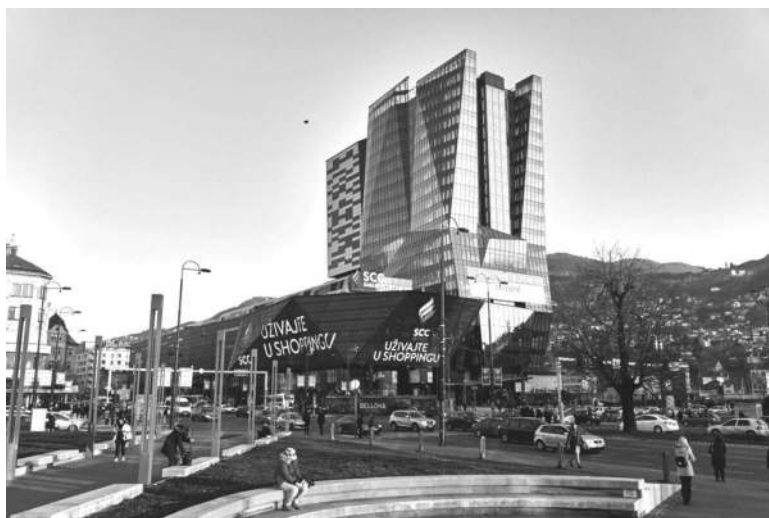
FIGURE 5.2 Sarajevo City Centre (outside).
