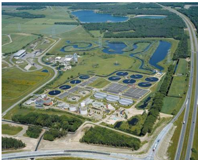
Figure 13.2 Overview of the STP Tilburg.
