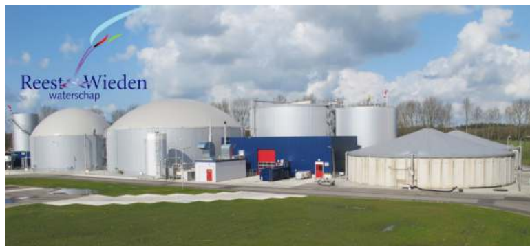
Figure 13.1 Overview STP Echten of the waterboard Reest & Wieden.
