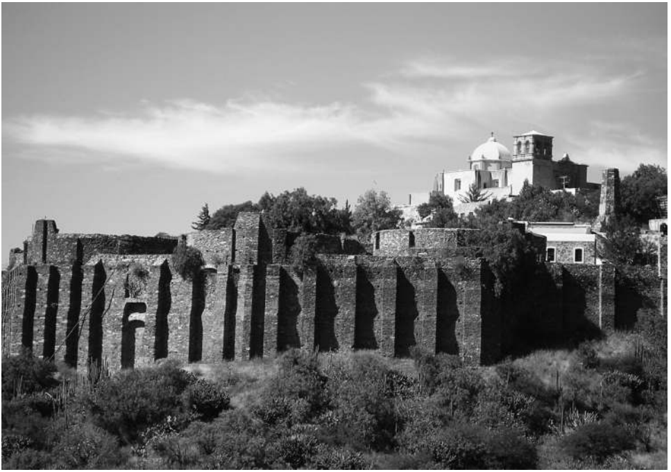
FIGURE 1.1. In the heights of silver capitalism: The Rayas Mine and Mellado Church, Guanajuato, Mexico. Author photo
