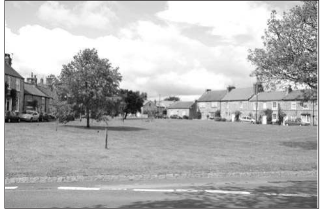
Fig. 4.22. Planned village at Catterick: a Washland village set around a green, distinct from the linear arrangement of 18th century inns and other service buildings that were established alongside the Great North Road, nearby to the east (photo: Blaise Vyner)
