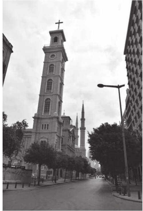
Fig. 19.5: The new campanile built to the south-west corner of the St. George Maronite Cathedral (Assaad Seif).
