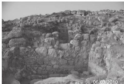
Fig. 6.5: Mamluk-era vaulted structure with doorway in Field M, view upslope. Note Early Islamic, Byzantine and Roman walls below (project files).
