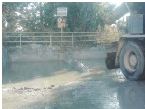
Figure 2. Sedimentation tank for the water-washing of the trucks.
