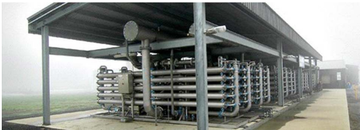
Figure 17.1 View of the ultrafiltration water recycling plant, eastern irrigation scheme (Photograph courtesy of Water Infrastructure Group, Melbourne).
