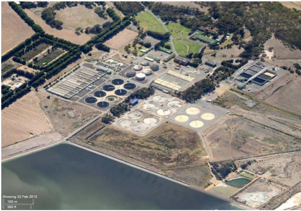
Views of the Bolivar water recycling plant.
