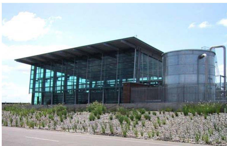
Figure 11.2 Homebush Bay Water Recycling Plant (Photograph courtesy of Sydney Olympic Park Authority).
