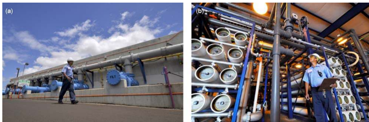
Figure 9.3 Views of the the Honouliuli Water Reclamation Facility and the membrane microfiltration unit ( Photograph courtesy of Veolia Water and Bryan Spear ).
