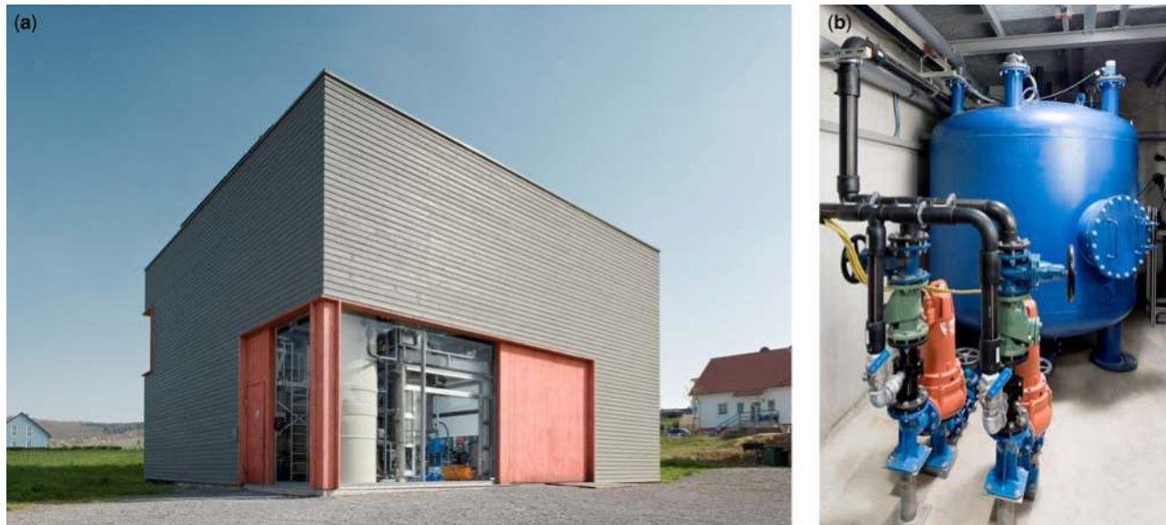
Figure 7.1 Photographs of the “Wasserhaus” in Knittlingen and the vacuum station in the basement.
