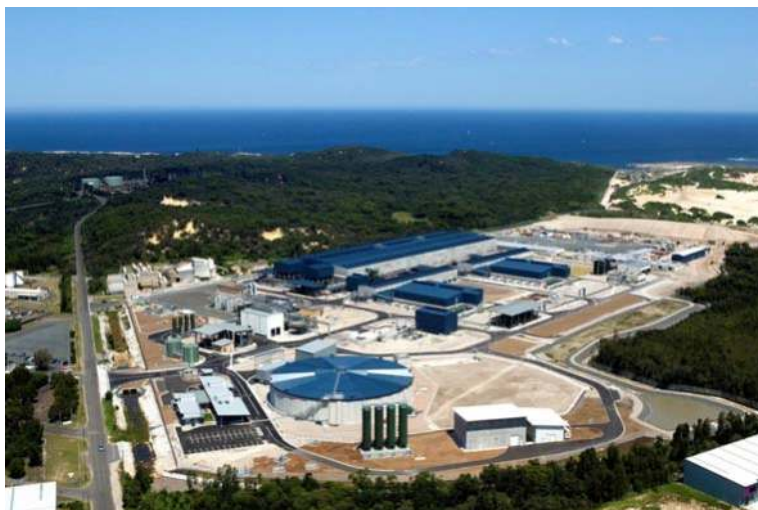
Figure 1.5 The Sydney desalination plant at Kurnell (Photograph courtesy of Sydney Water).
