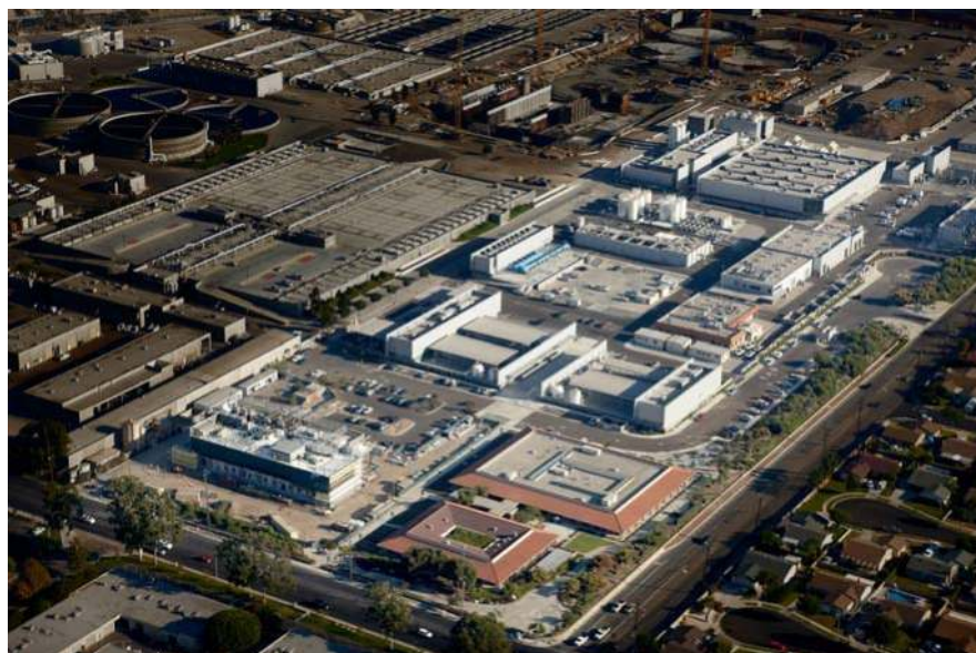
Figure 25.11 Aerial view of the Advanced Water Purification Facility (Photo credit: Larry Mack).
