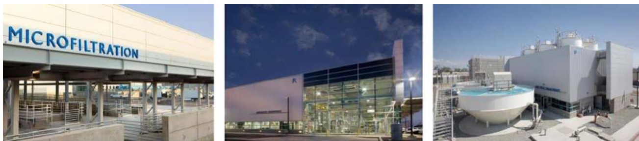
Figure 25.6 View of GWR process buildings: microfiltration, reverse osmosis and lime treatment (Photo credit: Larry Mack).
