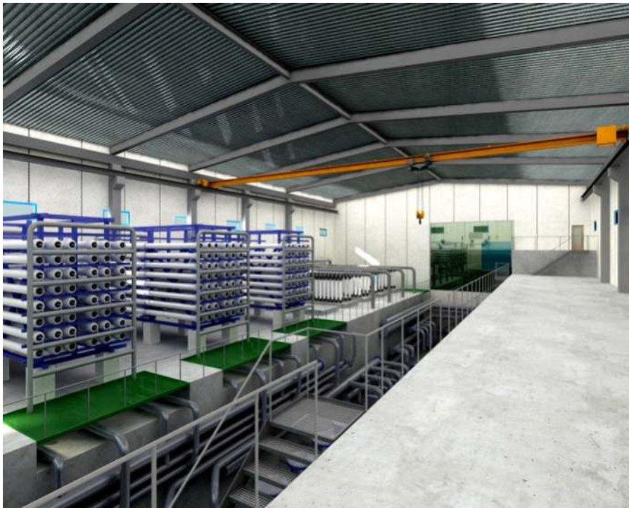
View of the advanced reclamation facility using ultrafiltration hollow fiber membranes and two-stage reverse osmosis to produce high quality recycled water for the Holmen Paper industry.
