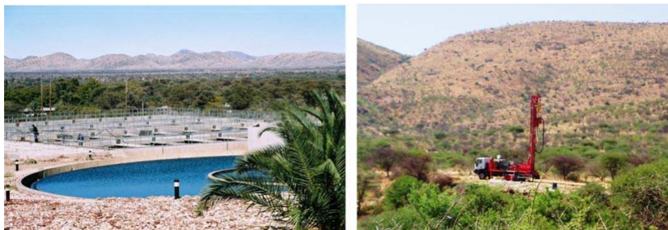
Figure 29.2 View of the Von Bach Dam WTP and Borehole Drilling in the Auas Mountains.
