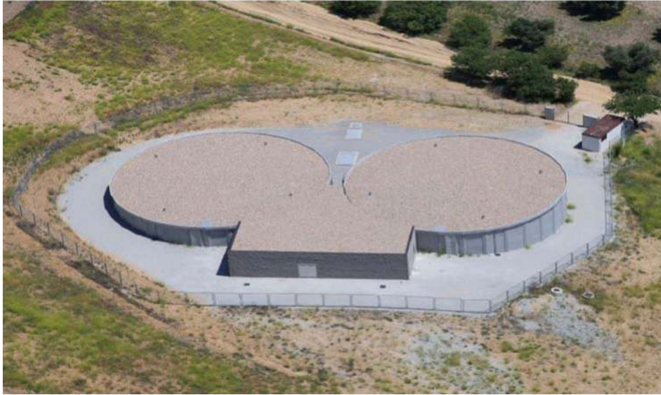
View of the water reuse holding tank and pumping station in Parla, Madrid.
