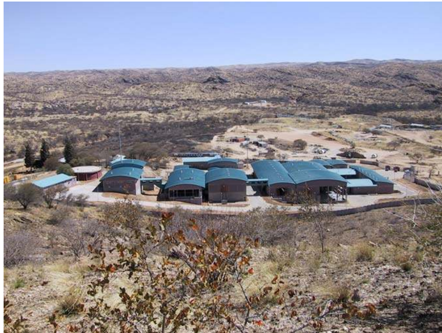
View of the New Goreangab Plant in Windhoek, Namibia.
