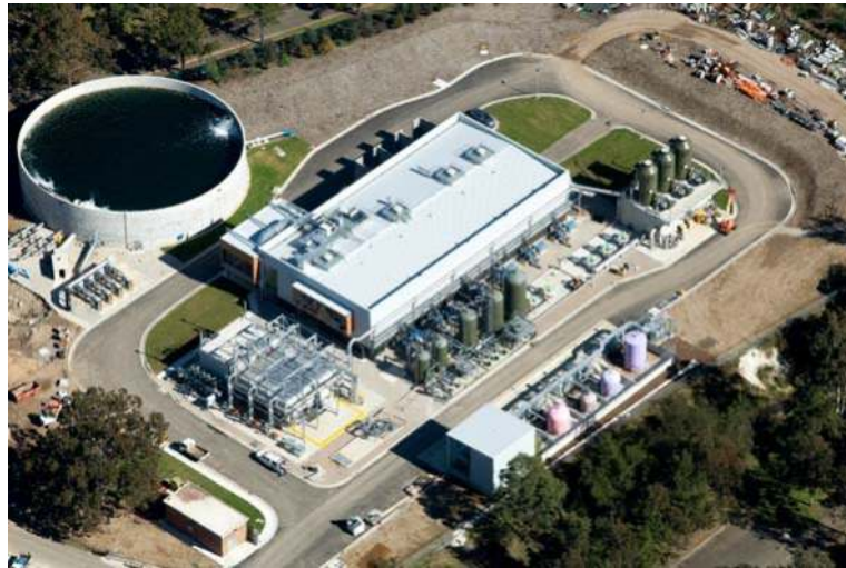
Figure 1.4 St Marys water recycling plant supplies 18 Mm 3 /yr for environmental flows (Photograph courtesy of Sydney Water).
