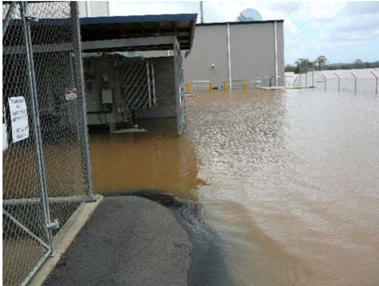
Figure 28.6 Bundamba AWTP during the 2011 Brisbane flood.
