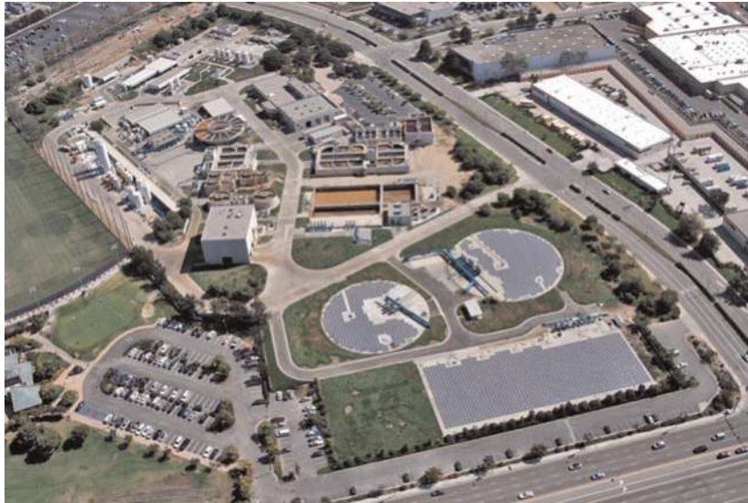
Figure 2.6 Aerial view of the Edward C. Little Water Recycling Facility in West Basin with solar panels.
