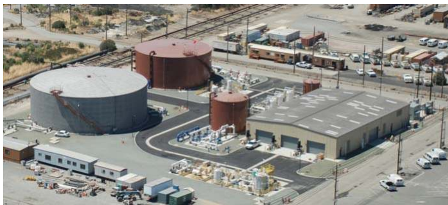
Figure 20.4 Aerial view of completed RARE treatment plant with the storage reservoir.
