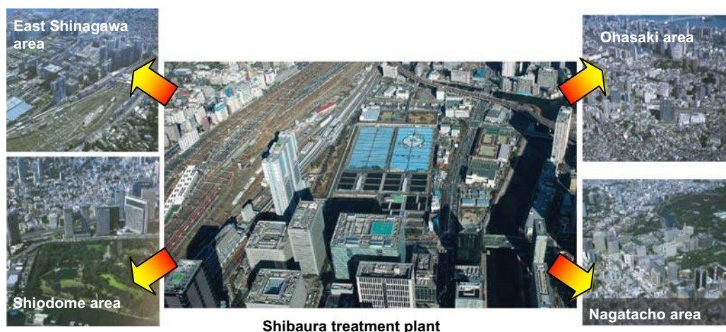
Figure 12.3 Views of the Shibaura Wastewater Reclamation Plant and four urban areas supplied with recycled water (Photography credit: Tokyo Metropolitan Government).
