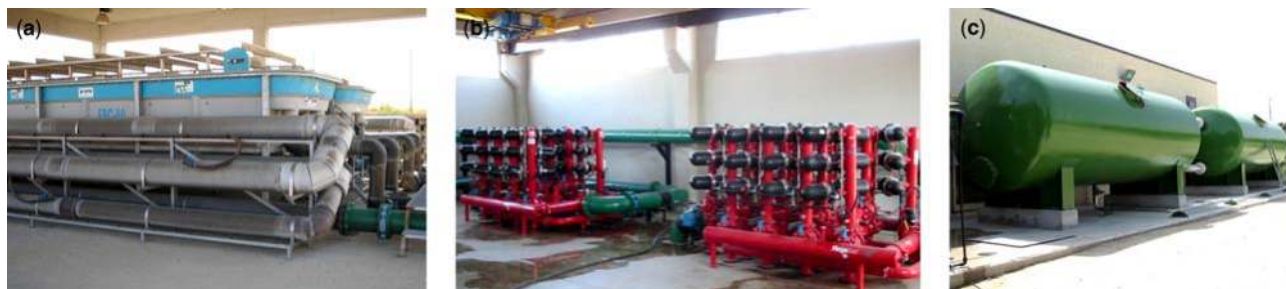
Figure 8.2 Views of tertiary pre-treatment processes: from left to right lamella settling (a), ring filters (b) and sand filters (c).
