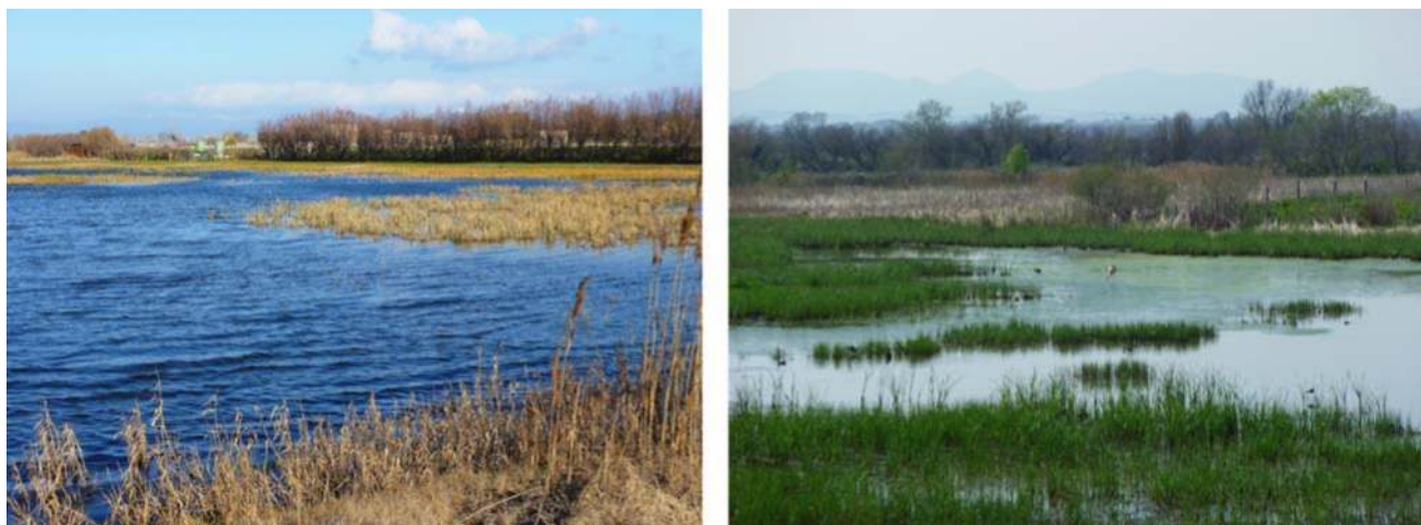
Figure 4.3 View of Empuriabrava constructed wetland system.
