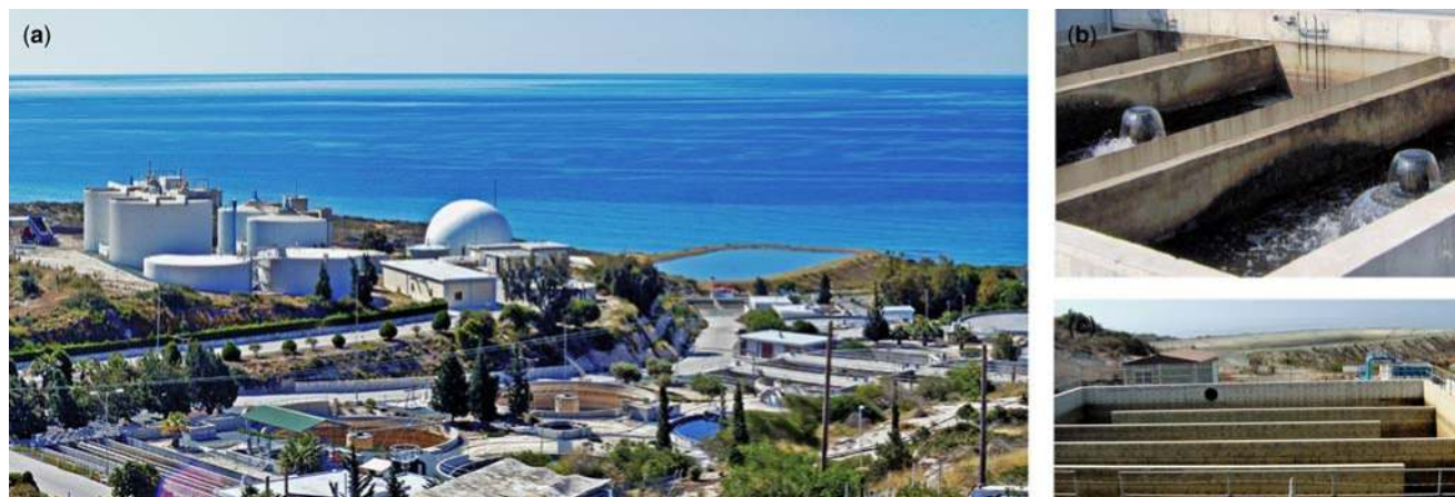
Figure 5.2 (a) A general view of the biological WWTP of Limassol (b) the tertiary treatment stage of sand filtration and (c) chlorination (the storage tank can be also seen at the back).
