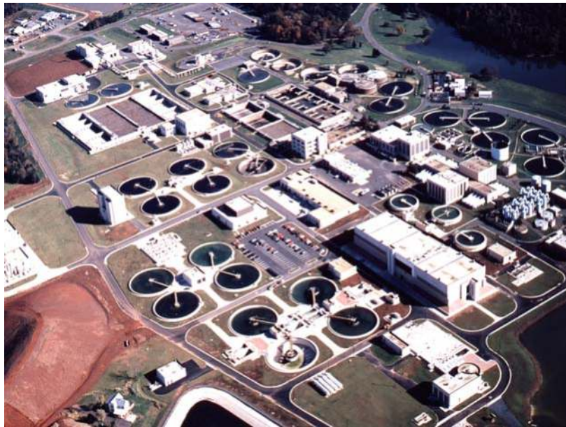
Figure 27.3 Aerial photo of a portion of the 204,400 m 3 /d (54 MGD) UOSA water reclamation plant known as the Millard H. Robbins, Jr. Water Reclamation Facility.
