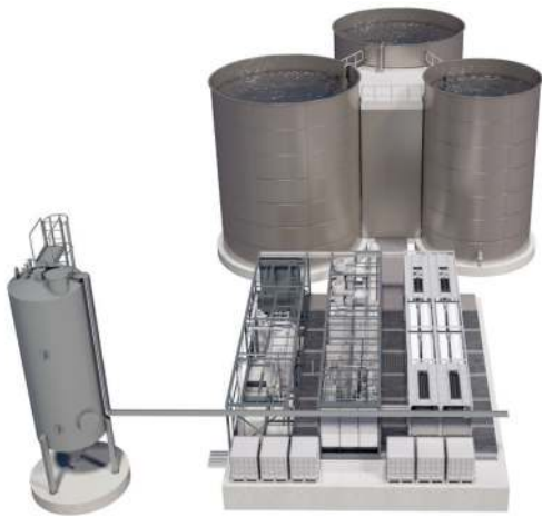
Figure 6.16: Arla -Vimmerby MBR WWTP in Sweden based on the Grundfos BioBooster modular concept. The concept of a Biobooster system and similar concepts, which have emerged in recent years, is a modular decentralised wastewater plant that is pre-assembled and can be delivered on trucks on site. The modularity allows for easy extending of the plant in case of increased load and vice versa.
