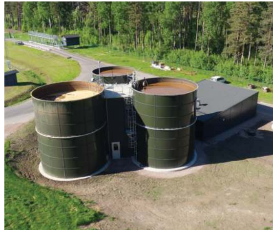
Figure 6.16: Arla -Vimmerby MBR WWTP in Sweden based on the Grundfos BioBooster modular concept. The concept of a Biobooster system and similar concepts, which have emerged in recent years, is a modular decentralised wastewater plant that is pre-assembled and can be delivered on trucks on site. The modularity allows for easy extending of the plant in case of increased load and vice versa.
