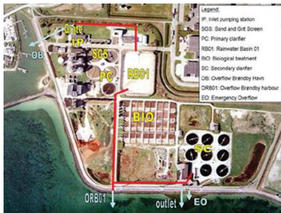
Figure 6.24: Aerial view of Avedøre WWTP.
