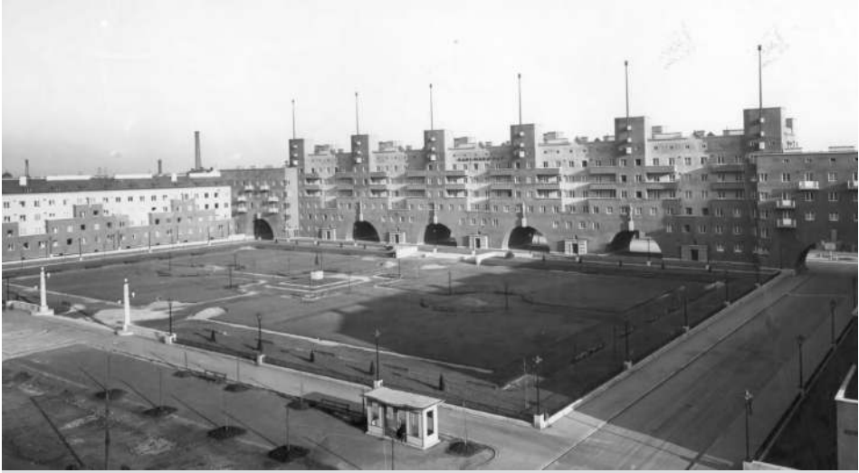
Fig. 127: The forecourt and central tract of the Karl Marx Hof in Vienna around 1930. Source: Municipal and Provincial Archives of Vienna, 3.3.2.FC1.2961M.
