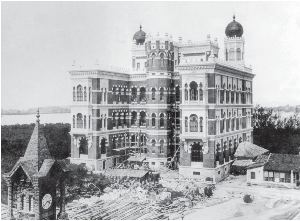
Construction of new buildings in 1908, when Adolpho Lutz was transferred to Instituto Soroterápico Federal, whose name was changed to Instituto Oswaldo Cruz in March that same year (DAD/Fiocruz).
