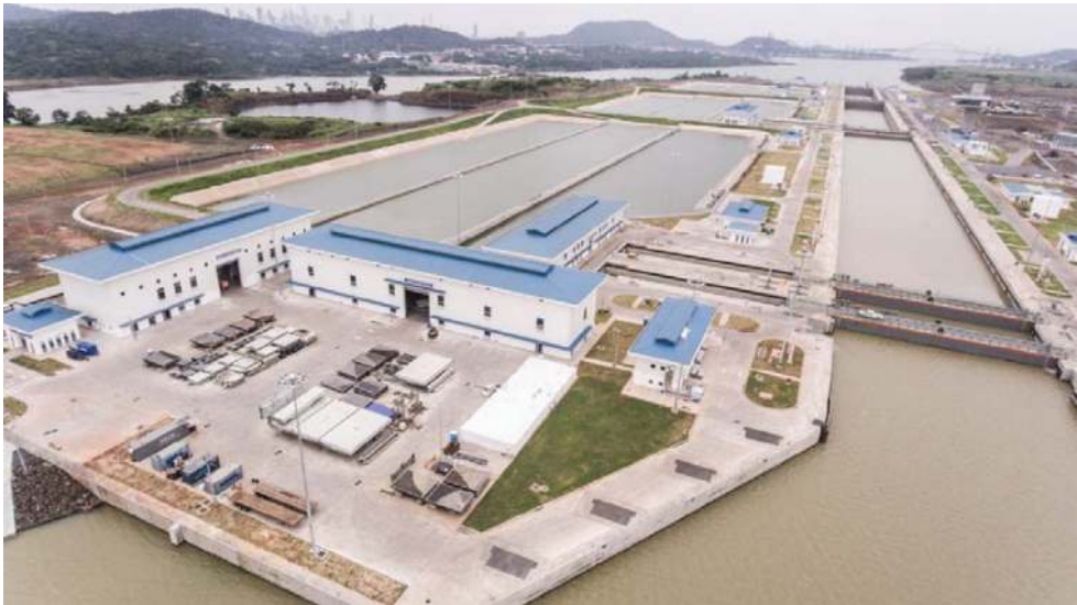
Figure 10. Overview of the structure where the two gates are located at each end of the chamber.
