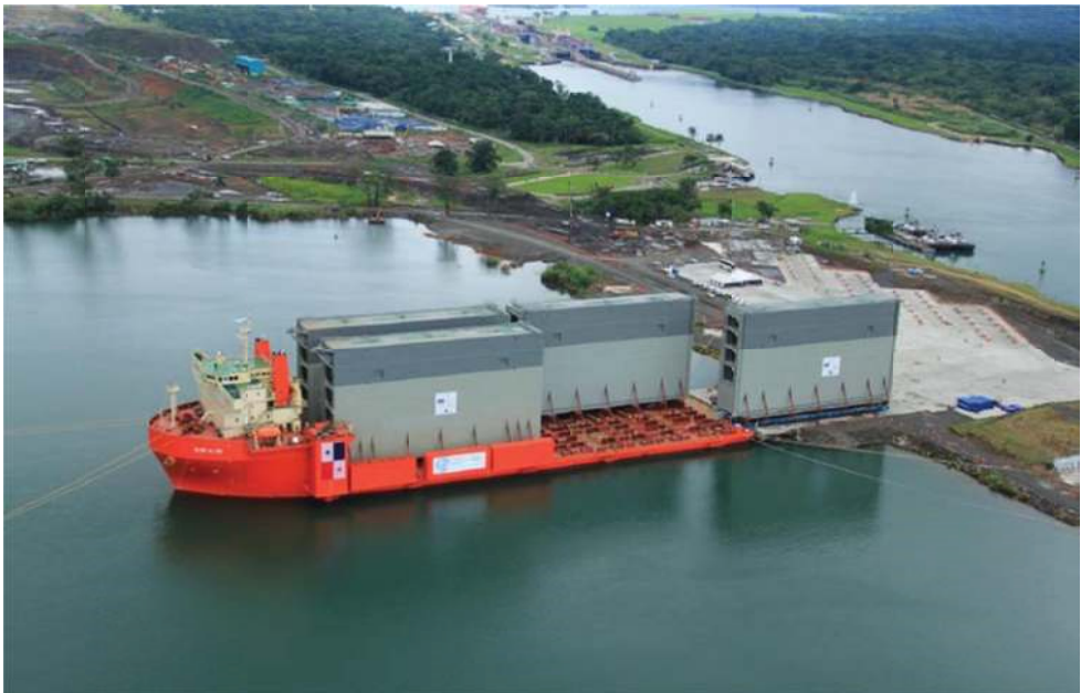
Figure 11. Unloading of the gates on the quay side Atlantic.
