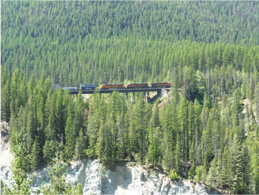
Fig. 18.4 A Burlington-Northern Santa Fe freight train crosses the Sheep Cr. Trestle
