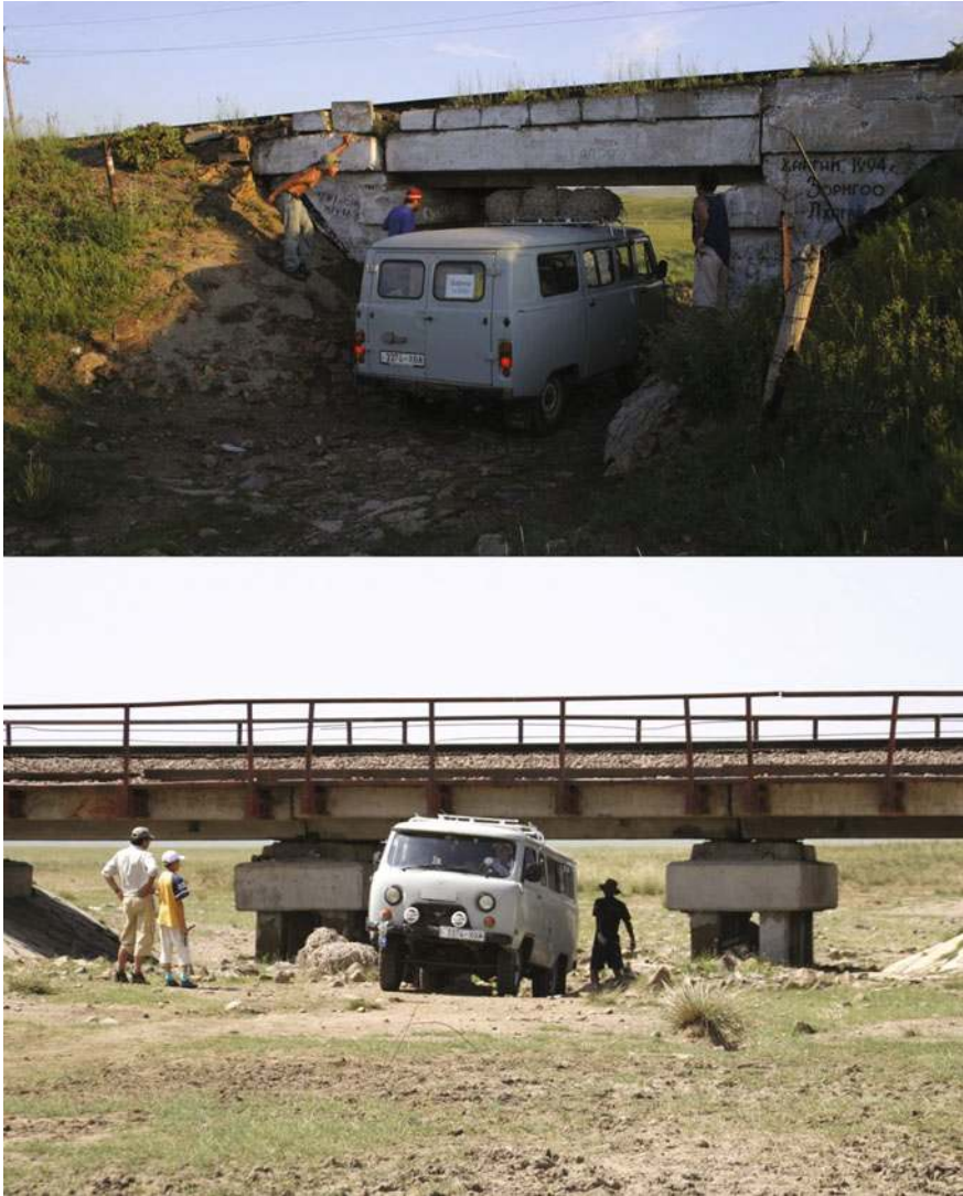
Fig. 14.4 Underpasses on the Ulaanbaatar–Beijing Railway
