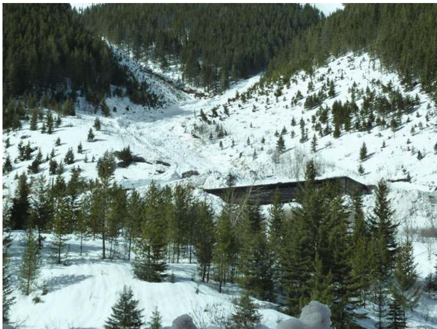
Fig. 18.5 An avalanche partially buries a snow shed on the Burlington-Northern Santa Fe railroad in the John F. Stevens canyon
