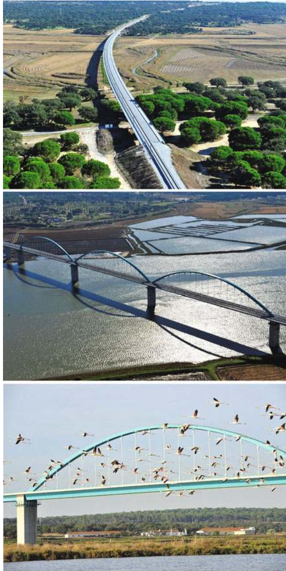
Fig. 7.2 Photographs illustrating aspects of the study area. Upper panel railway crossing rice fields (São Martinho stream); middle panel bowstring railway bridge crossing the Sado River; lower panel flock of flamingos flying close to the Sado railway bridge
