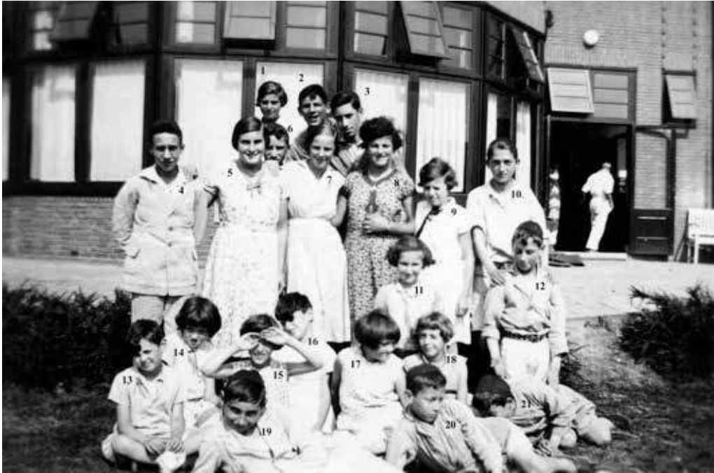
Figure 5.5: Summer 1934. Photo taken by Mimi Weiman at the back of the building, in front of the half-round annex.
