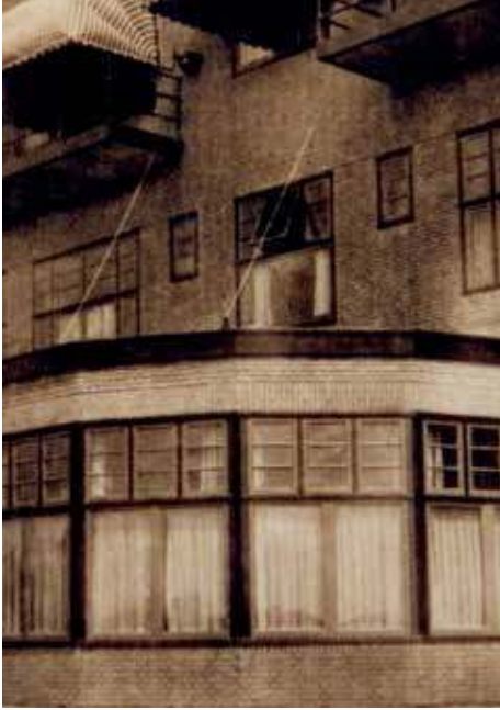
Figure 3.7: The back side, just after completion in 1929, showing the annex and the two cables by which the roof could be elevated during Sukkot.
