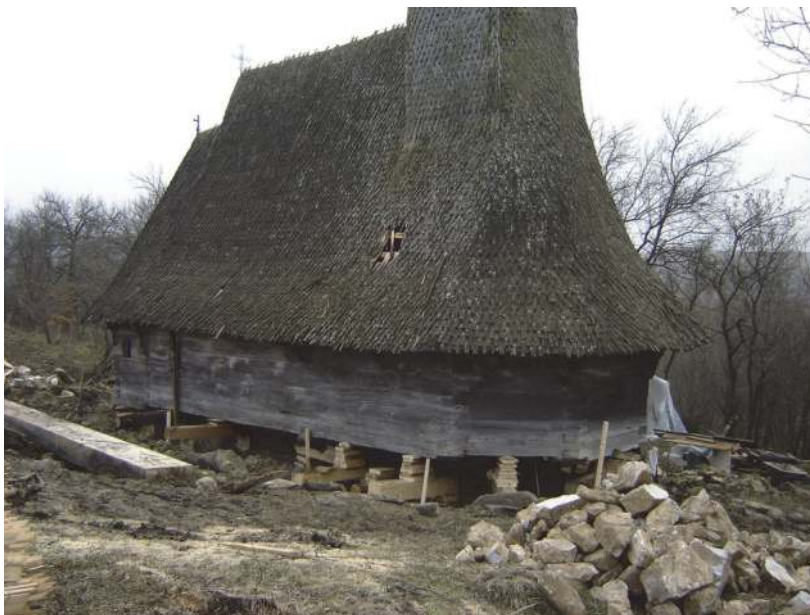
Figure 5. The lifting of the church.
