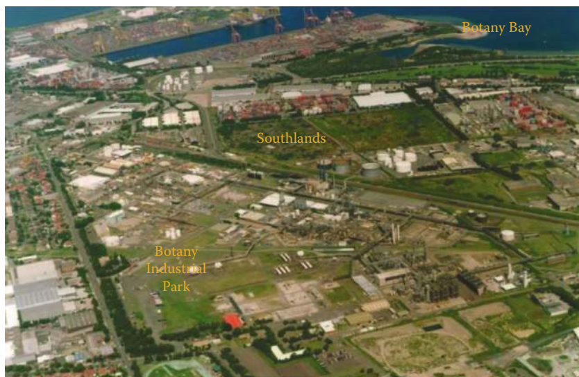
FIGURE 12.2 BIP and surrounds. (From Orica Ltd.)
