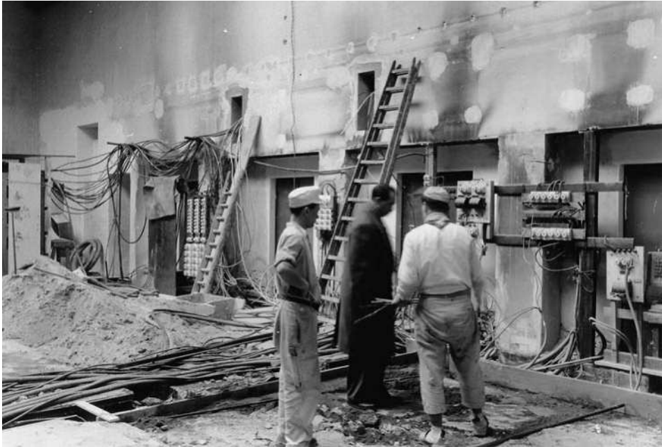
Fig. 4.10. Refitting the "Machine Hall," circa 1955.
