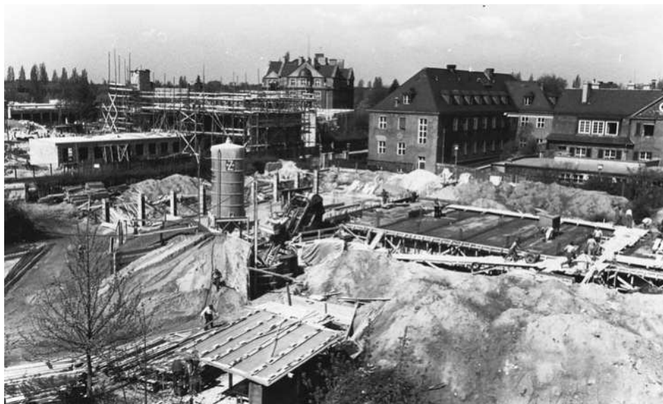
Fig. 4.20. Construction site of the Institute for Electron Microscopy, the library and the administration building, 9 May 1958. In the background on the left, the construction site of the campus of the Freie Universität.
