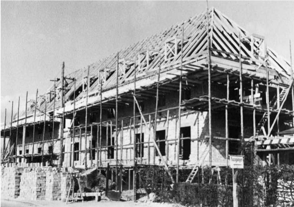
Fig. 3.12. Framing of the new X-ray building, 1938.
