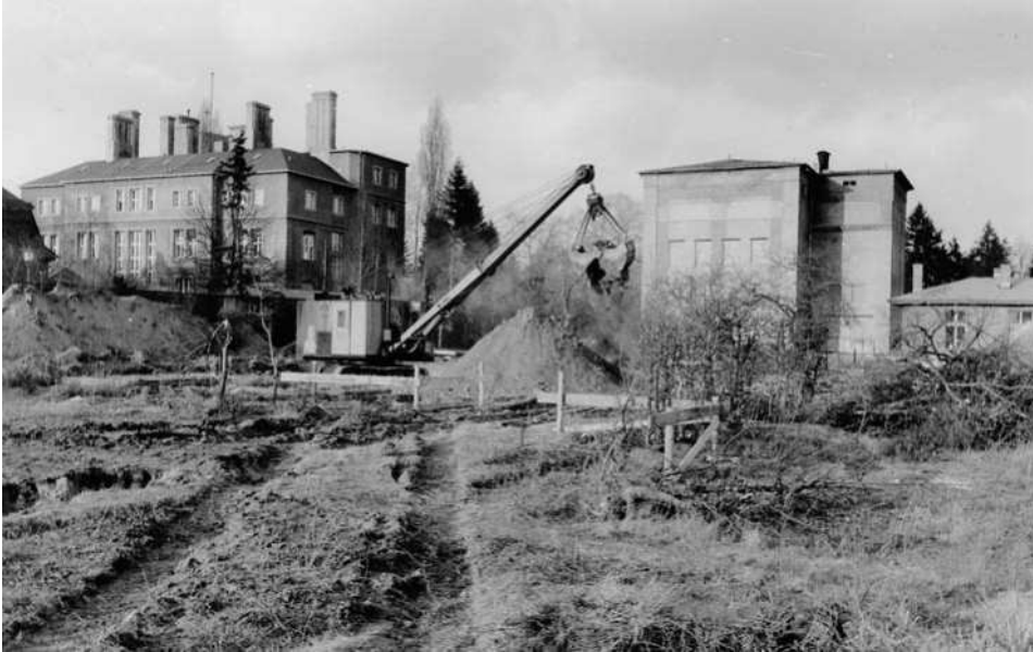
Fig. 4.18. The site being prepared for the construction of the library and administration building, 10 March 1958. On the left, the main building of the FHI. On the right, the Minerva Tower and, far right, the "Radium Hut" of the former KWI for Chemistry.
