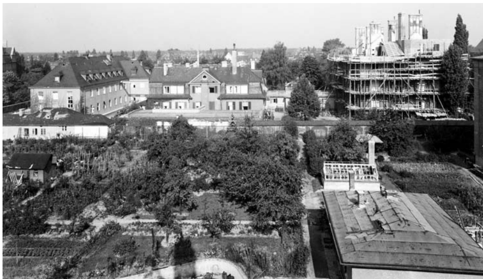
Fig. 3.20. KWI for Physical Chemistry and Electrochemistry, Summer 1944. The destroyed sections of the roof of the main building are being replaced.
