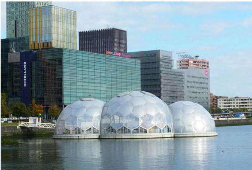
Figura 6-10: Floating Pavilion, Rotterdam 2014.
