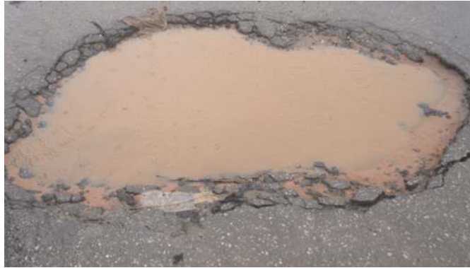
Figure 3. Showing how water aids road failure.
