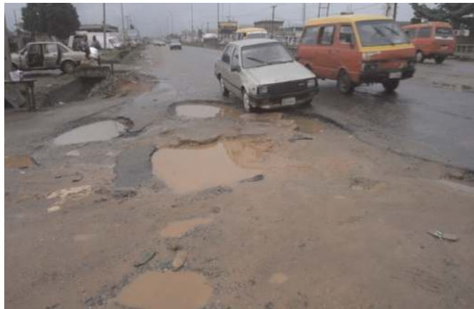
Figure 4. Showing how water aids road failure.
