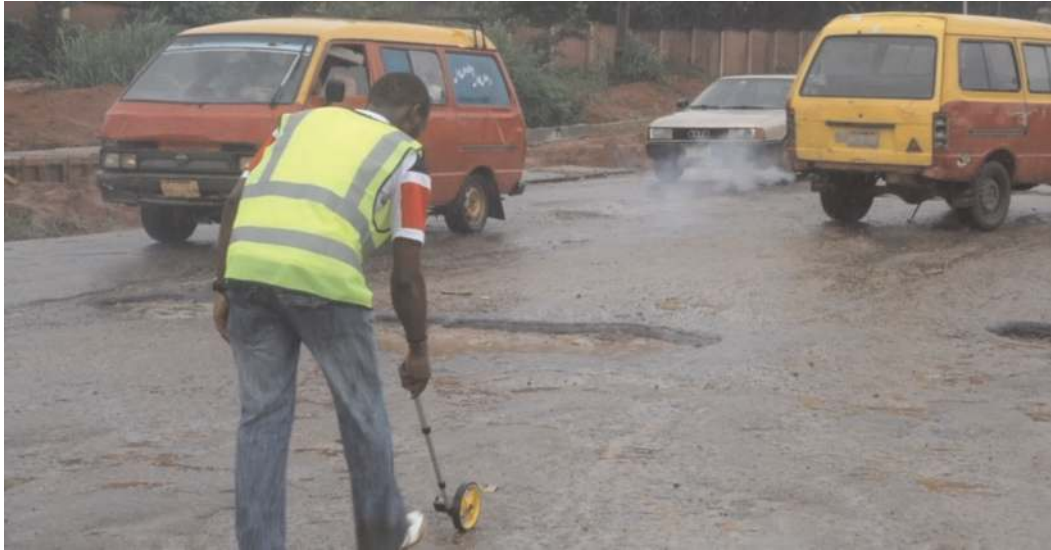
Figure 12. Failed portion in Upper Sapele Road.
