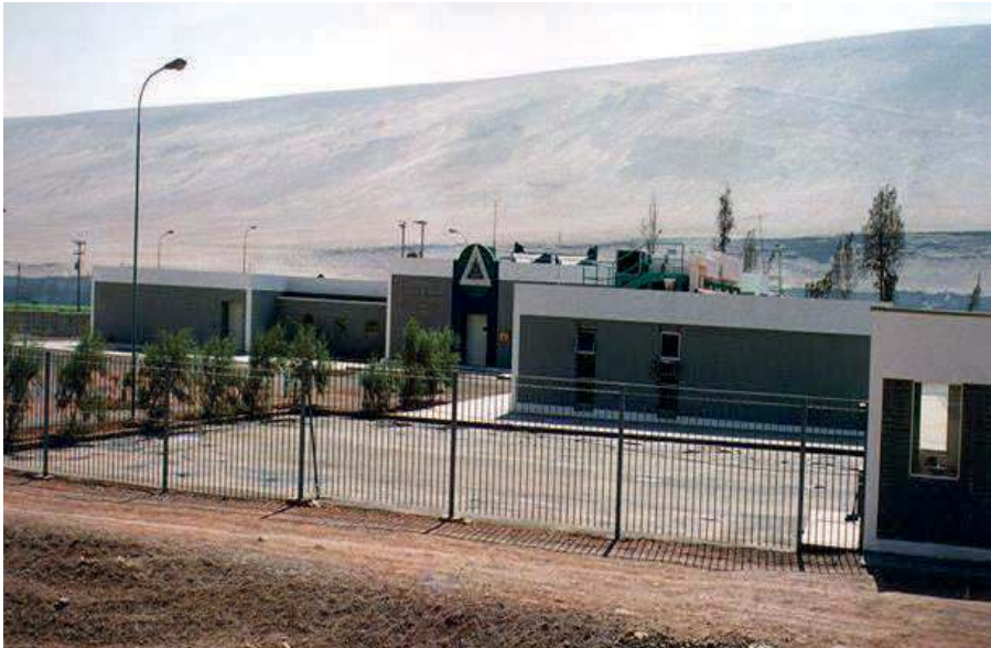
Figure 8. Mediterranean fruit fly mass-rearing and sterilisation facility in Arica, Chile (photo from R. Rodríguez SAG Chile; reproduced with permission).
