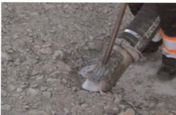
Figure 4. Removing soil with the vacuum / sucking lorry.
