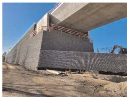
Figure 6. Direct bridge abutment G03 after the launch of the bridge.
