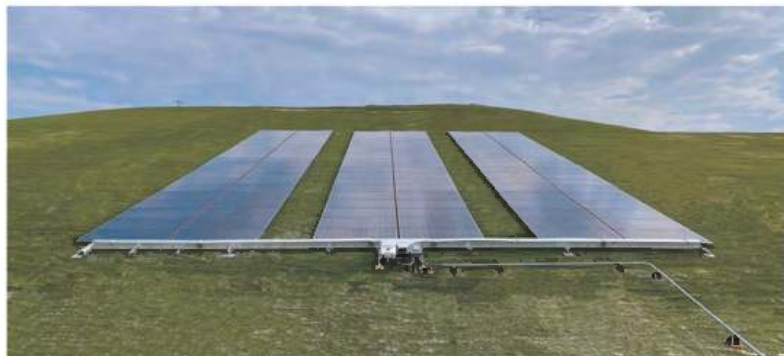
Figure 7. PowerCap installed on engineered turf cover at a confidential CCR impoundment, Southeastern US.
