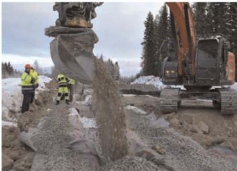
Figure 6. Filling of the trench with granular material.
