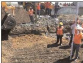
Figure 8. Checking the excavation level.
