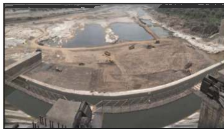
Figure 8. Execution of multistage secondary apron (Kapadia 2020).
