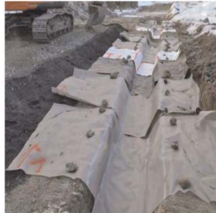
Figure 5. Installed geotextile samples.
