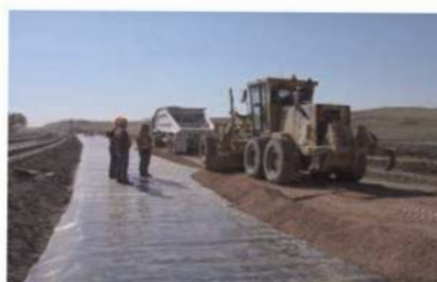
Figure 6b. Sub ballast placement directly on BGM.
