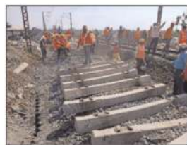
Figure 16. Placing sleepers over ballast.
