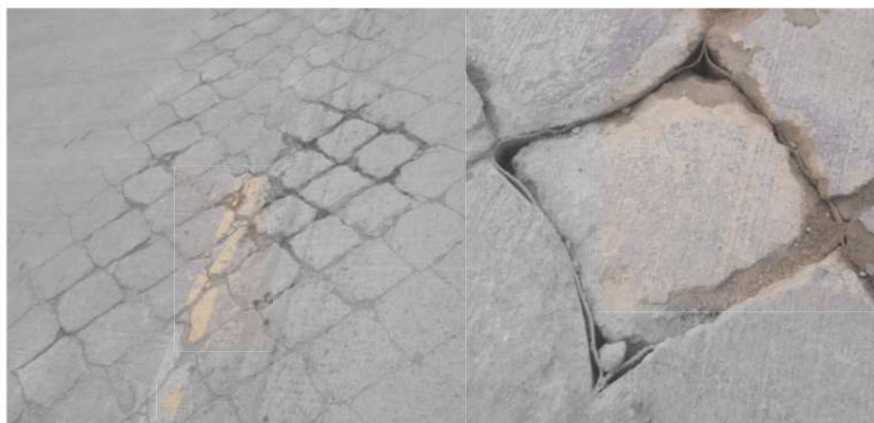
Figure 6. Fail presented in a soft soil with high fines and water presence.
