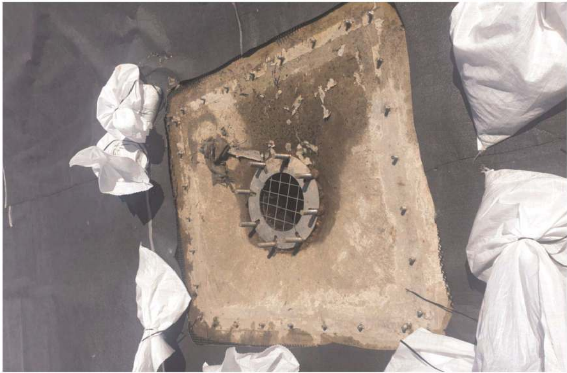
Figure 8. An old concrete structure for a scour outlet.
