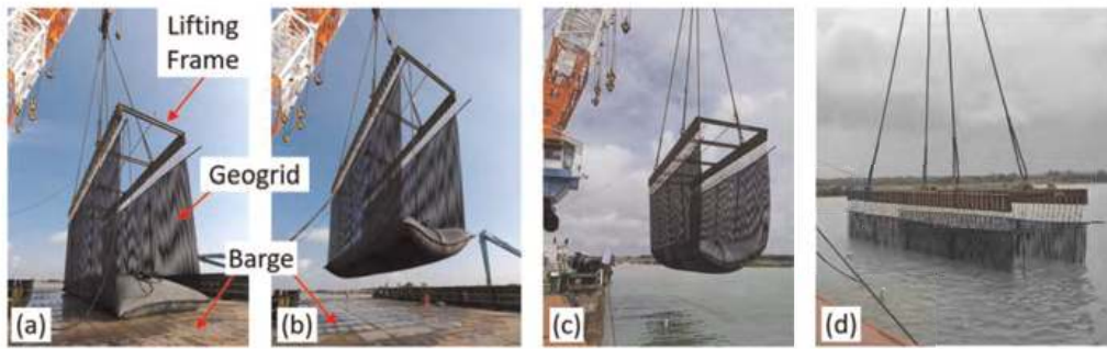
Figure 7. Lifting and lowering process: (a) Setup of lifting frame and geogrid; (b) Lifting of geotextile tube from the barge; (c) Shifting of barge that was used to install the geotextile tube; (d) Lowering of Geotextile tube into the water.
