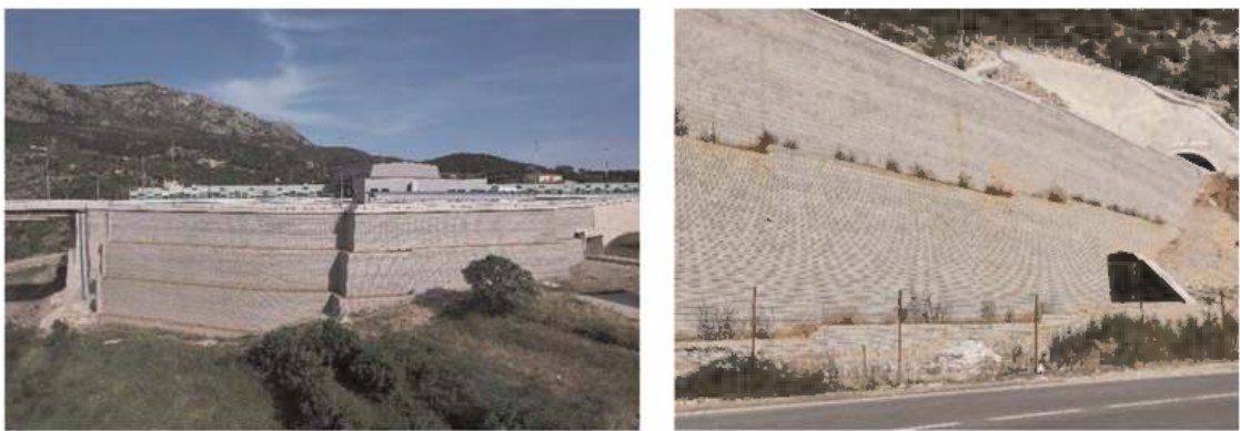
Figure 7. a) Angular wall for highway widening at toll station; b) Wall at tunnel entrance.
