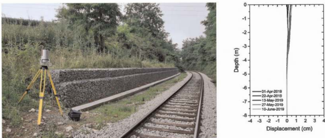
Figure 4. Retaining structure after completion (left) and horizontal displacements in borehole above the retaining wall (right).
