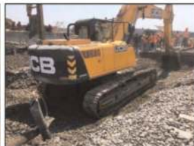
Figure 5. Removal of sleepers.
