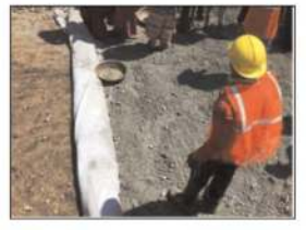
Figure 10. Infilling 100mm thick blanket layer.
