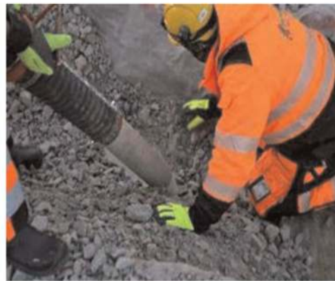
Figure 10. Removal of last part of granular material using a vacuum and by hand.
