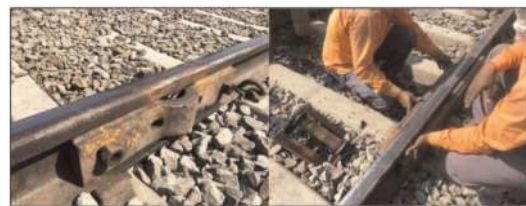
Figure 17. Placing rail fish plates; left picture shows stiffening fishplate.
