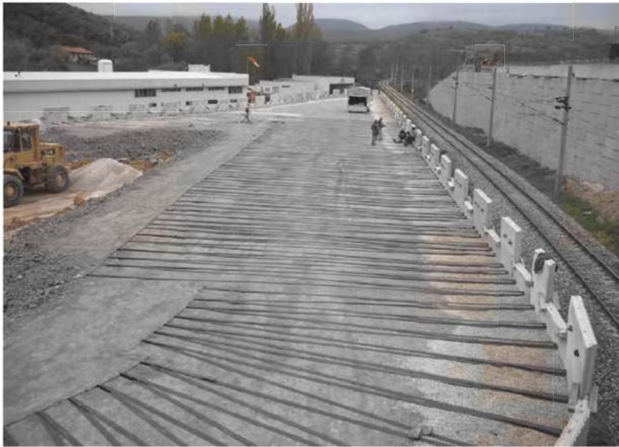
Figure 1. Polymeric strips extending from the rear side of the concrete panel.
