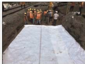
Figure 9. Laying the nonwoven geotextile.
