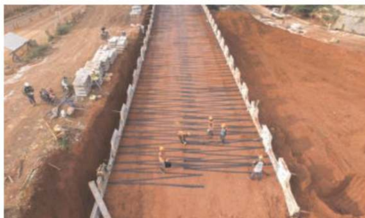
Figure 2. Construction of geoforce segmental retaining wall system.
