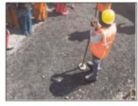
Figure 11. Compaction with manual hand tamper.
