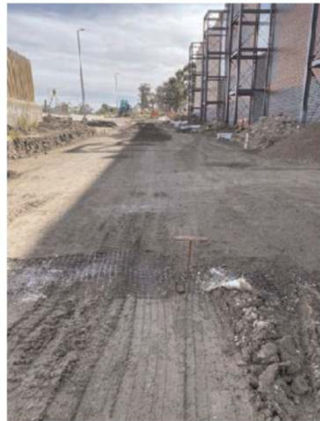
Figure 4. Final pavement ready for asphalt wearing course.
