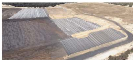
Figure 3. Aerial image of site during construction.
