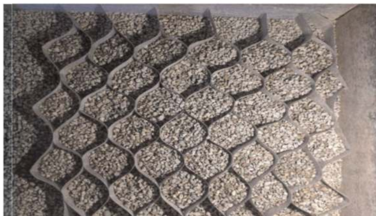
Figure 1. A view of installed geocell in the backfill.
