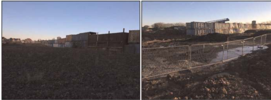
Figure 1. Cargo containers separating recycling facility & Housing development (prior to bund construction).
