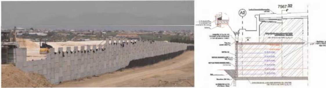
Figure 3. True bridge abutments in Nicosia orbital road: (a) elevation view; (b) cross section.
