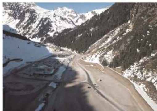
Figure 6. Rockfall protection dam Eisgratbahn-Stubaital.
