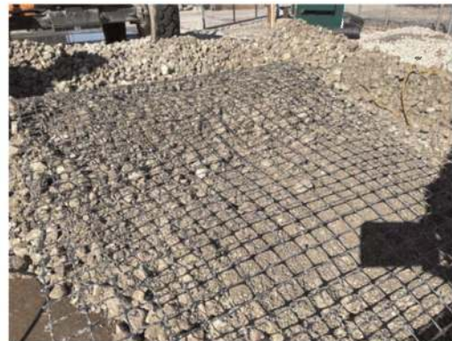
Figure 2. Close-up of UL-FGA and geogrid.
