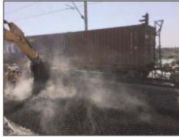
Figure 13. Infilling the geocells.
