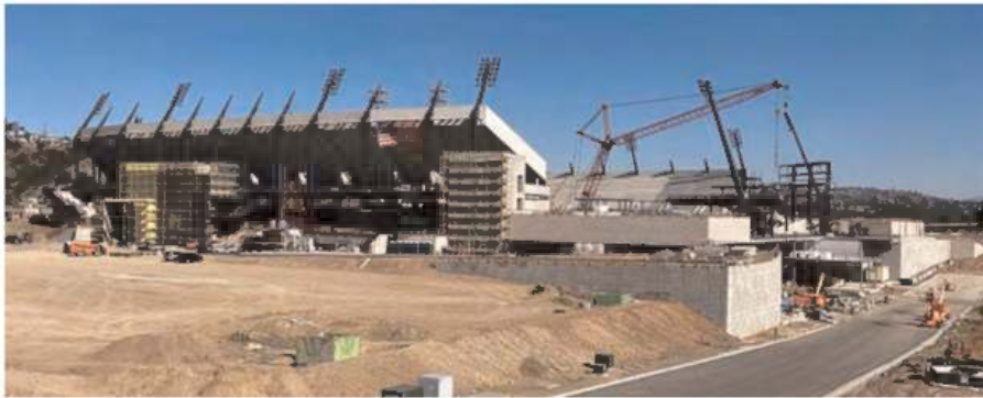
Figure 5. SDSU Stadium under construction.
