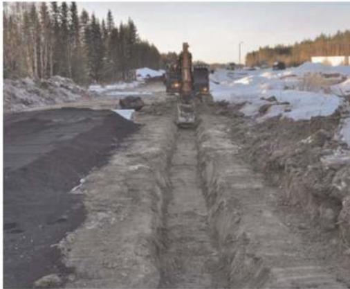
Figure 4. Excavation of trench.
