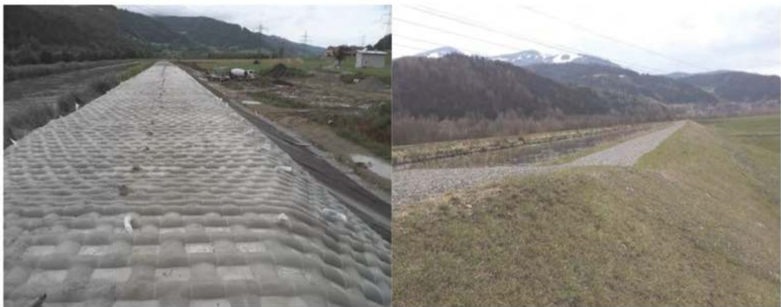
Figure 4. Concrete mattress: after installation (left); after being vegetated 2 years later (right).
