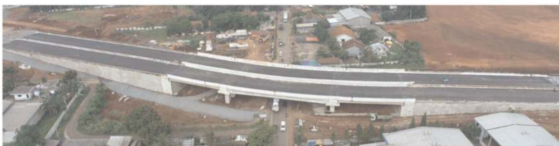
Figure 1. Kadusirung Flyover, Banten, Indonesia.
