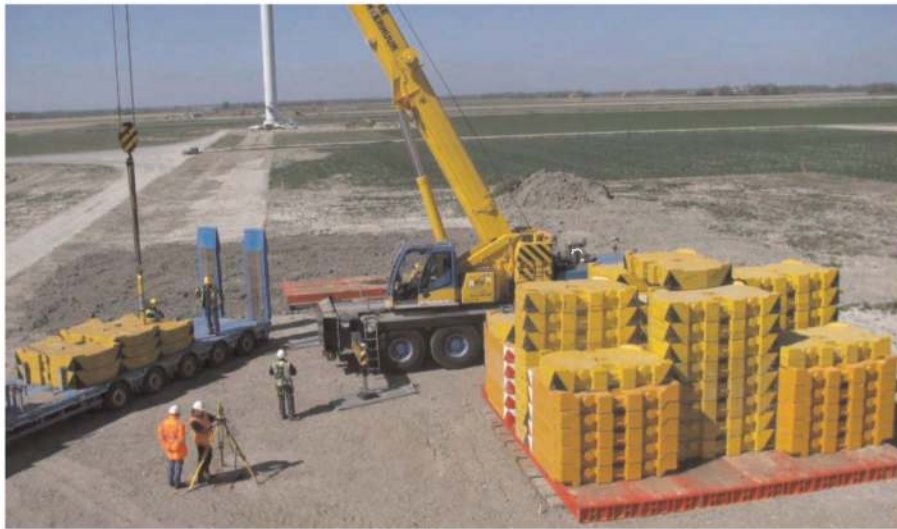
Figure 3. Wieringemier project – general view of the full-scale test.
