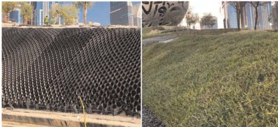
Figure 7. Geocell: before and after vegetation growth.
