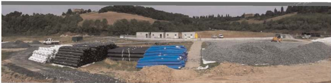
Figure 2. GCL and drainage geocomposite rolls stored on flat surfaces to avoid detrimental deformations.
