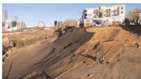
Figure 6. Installation of geocell.
