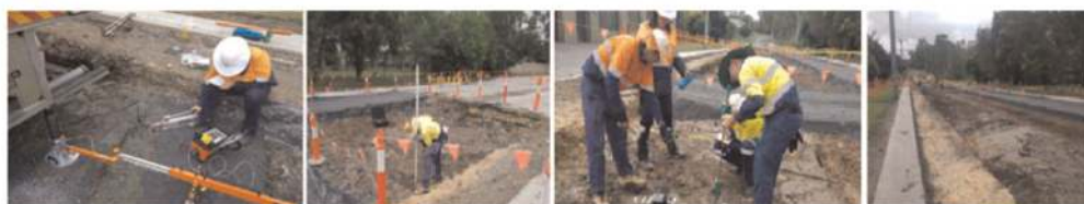
Figure 2. Subgrade preparation and testing.
