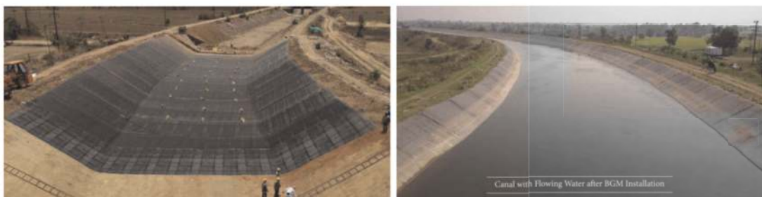
Figure 3. Canal during BGM installation and after 4 years of flowing condition.
