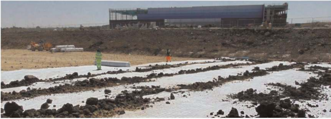
Figure 6. Placement of starter layer geocomposite prior to raising of formation level (ABG Geosynthetics Ltd).
