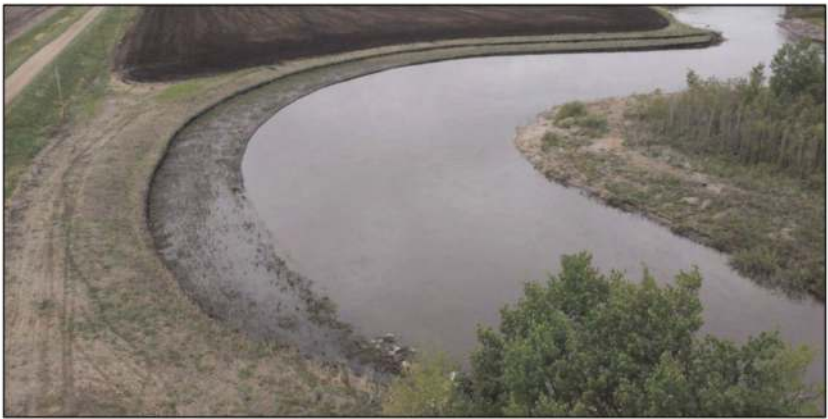
Figure 10. SCOURLOK and ARMORMAX performance during flood conditions, May 2022.
