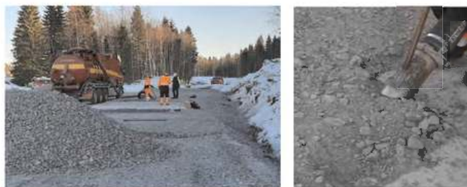
Figure 3. Vacuum lorry and system for sucking of material from the geosynthetics.
