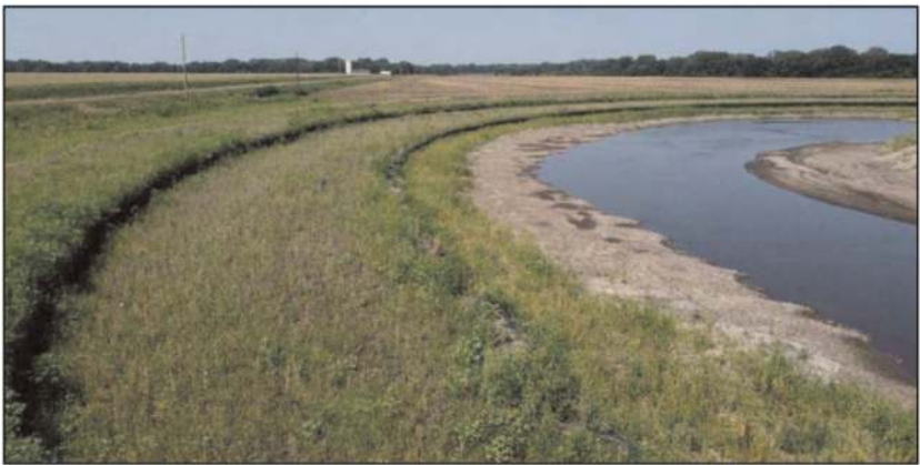
Figure 8. Vegetated SCOURLOK and ARMORMAX performance, July 2021.
