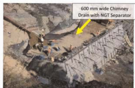
Figure 11. Internal drainage system shown during construction.
