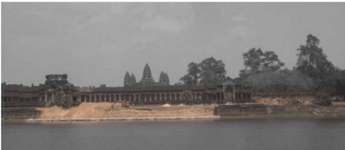
Figure 1. Intervention area during the rehabilitation intervention.
