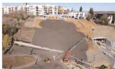
Figure 7. Filling of geocell.
