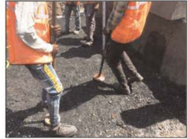
Figure 14. Watering and compaction of infill.
