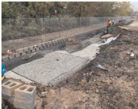
Figure 3. Photo of AASHTO #57 installation.
