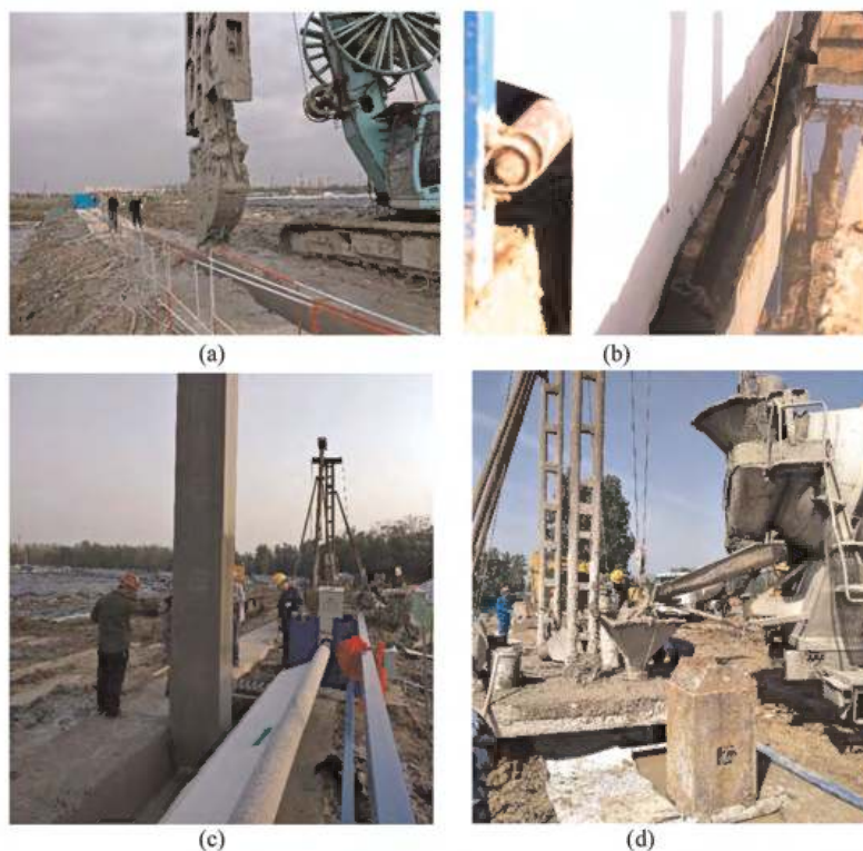
Figure 5. Construction of GCL composite vertical anti-seepage barrier: (a) Trench excavation, (b) Laying of GCL composite component, (c) Dropping down the joint box, (d) Pouring wall materials.
