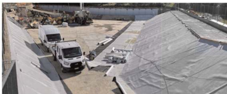
Figure 8. Photo of the geocomposite placing activities.
