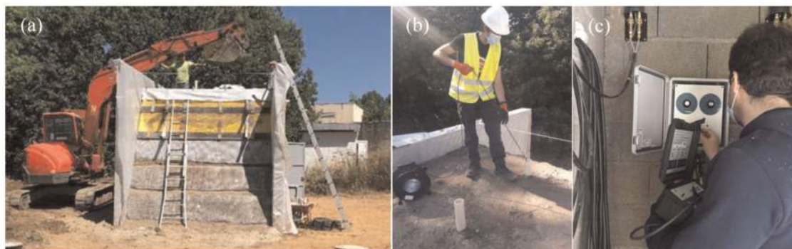
Figure 3. Full-scale instrumented geosynthetic-reinforced structure: (a) during construction; (b) readings on the inclinometers; (c) pressure cells readings.
