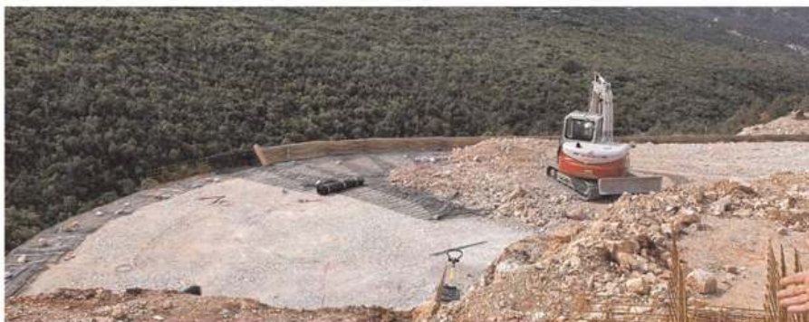
Figure 3. Construction phase of reinforced earth structure with mono-oriented extruded geogrids in HDPE.
