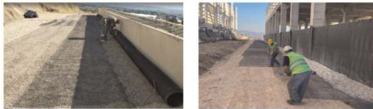
Figure 5. Installation of geogrids.
