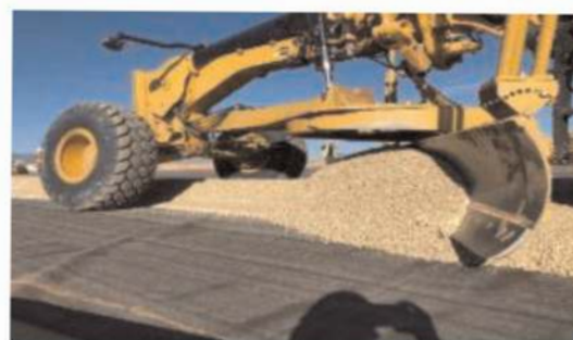
Figure 4b. Equipment and material over BGM.
