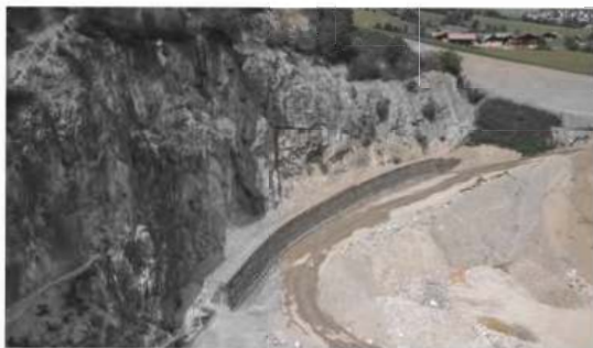
Figure 7. Rockfall protection dam Tenneck.
