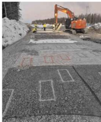
Figure 4. Installed geogrid materials with test samples pre-marked before base layer placement.
