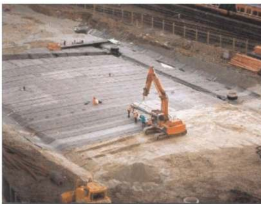
Figure 8a. Membrane installation.
