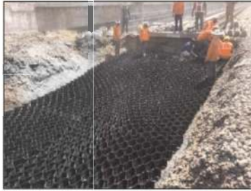
Figure 12. Bottom-most geocell layer.
