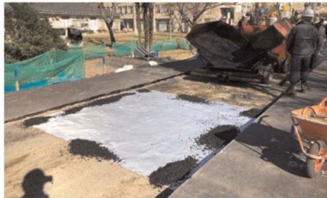
Figure 3. Placement of geotextile PET at 200 mm from the surface of prototype scale model test road.
