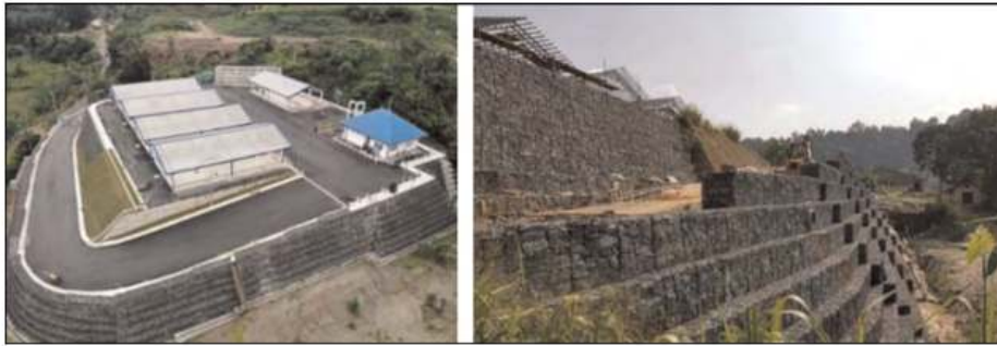
Figure 7. Completion of reinforced soil retaining slope.
