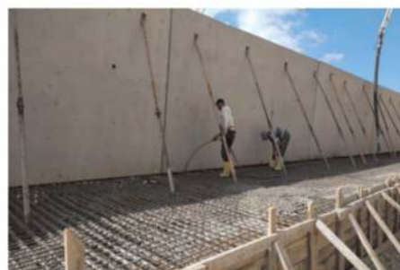
Figure 4d. Pouring of concrete.
