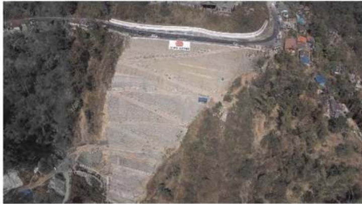
Figure 15. The completed structure.
