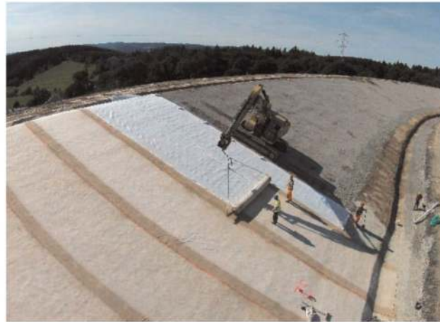
Figure 17. Geosynthetic drainage composite mat (white color) with a Geosynthetic Clay Liner (GCL, light brown) on top as sealing system.
