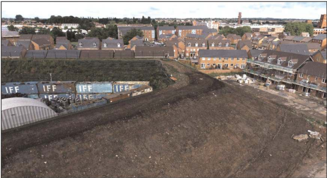
Figure 4. Aerial shot of the completed bund.
