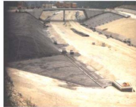
Figure 7b. Exit covered by BGM.
