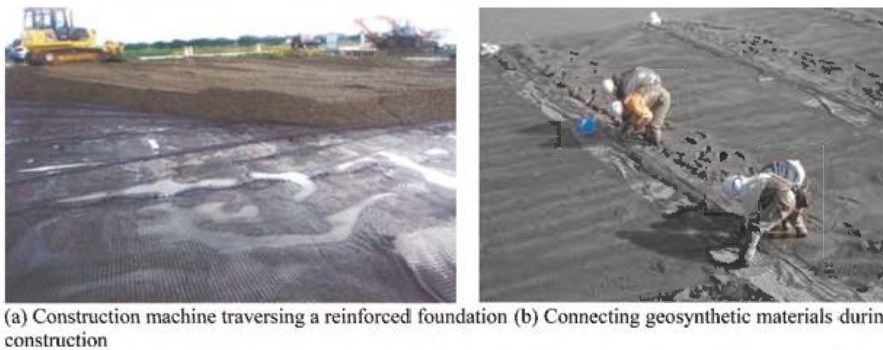
Figure 5. Case history of geosynthetic reinforcement applied to the surface layer in Japan.
