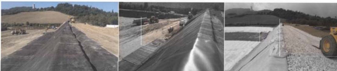
Figure 3. Slopes covered, from left to right, with the rough GCL, the HDPE liner, drainage geocomposite (slopes) and nonwoven geotextile (bottom).
