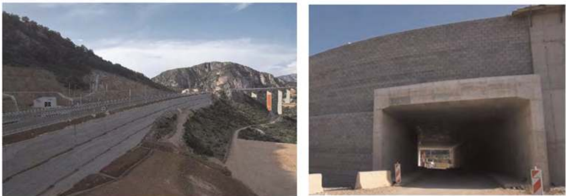
Figure 8. a) Wall with sudden height variation; b) Wall layout around a concrete culvert.
