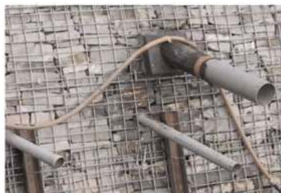
Figure 12. Sub-surface drainage outlets.
