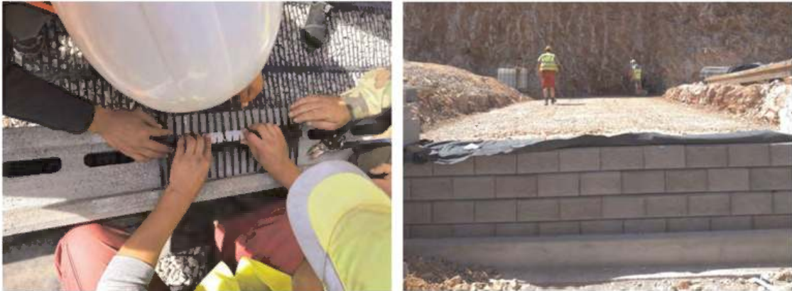
Figure 2. a) Top view of the concrete blocks with the connectors and the uniaxial extruded geogrids; b) Front view of the first row of blocks placed against the tooth of the concrete foundation pad.
