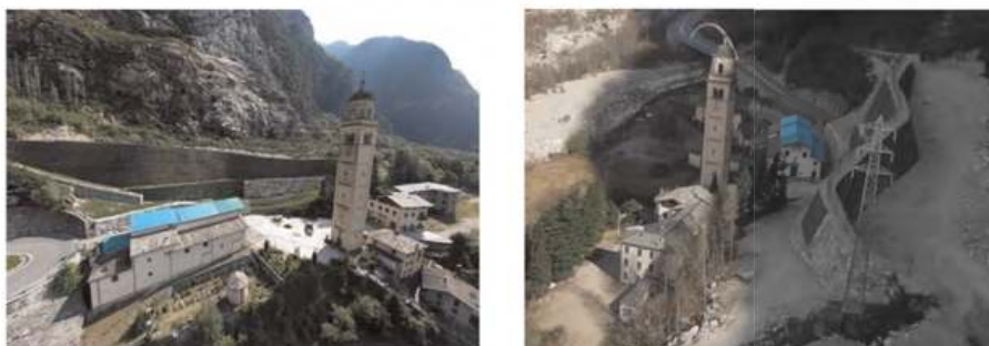
Figure 6. Aerial views of the finished works.
