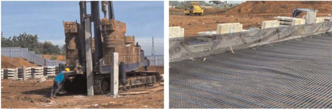
Figure 3. Geosynthetic reinforcement scheme in piled embankment system.
