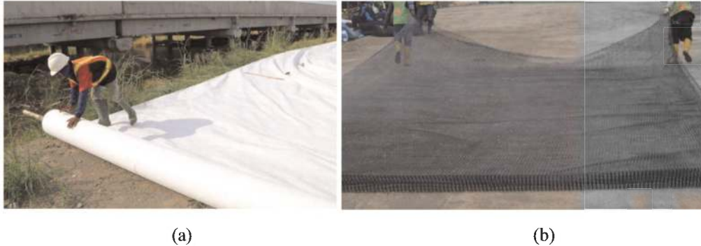
Figure 2. (a) Non-Woven and (b) Geogrid.
