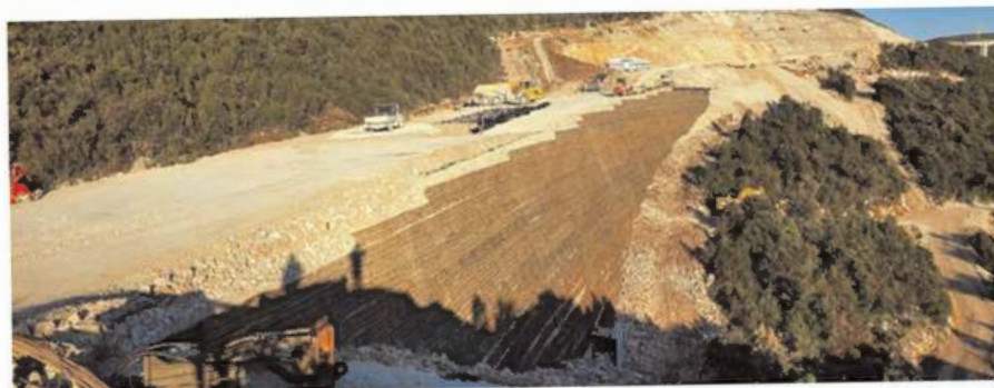
Figure 4. Replacement of the Doli viaduct with a wrap-around geogrid reinforced embankment (span 180 m, maximum height over 17 m).
