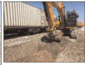
Figure 7. Removal of sub-ballast/blanket.
