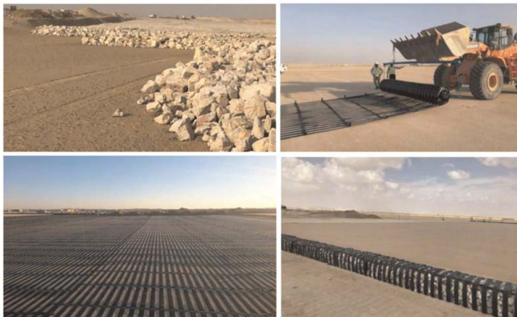
Figure 10. Stages of basal reinforcement installation.
