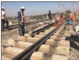
Figure 4. Removing rails.
