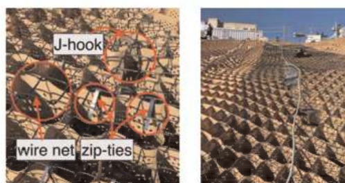
Figure 5. Installation of wire net with geocell.
