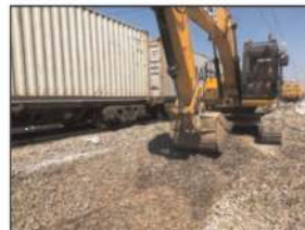
Figure 6. Removal of ballast.
