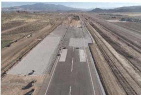
Figure 4a. General view of the site.
