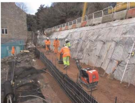
Figure 2. Wall under construction.
