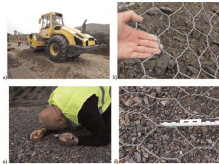
Figure 2. Procedure for installation damage of metallic geosynthetics: a) fill compaction on the sample; b) retrieving sample and identifying local damages; c) microscopic examination to assess exposure of the metallic core; d) indicating points where the metallic core is exposed.
