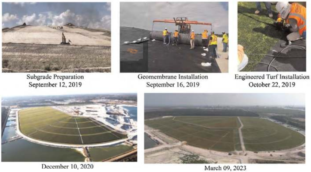
Figure 2. Engineered turf cover construction at the Mississippi phosphates corporation gypsum stack, a US EPA superfund site.
