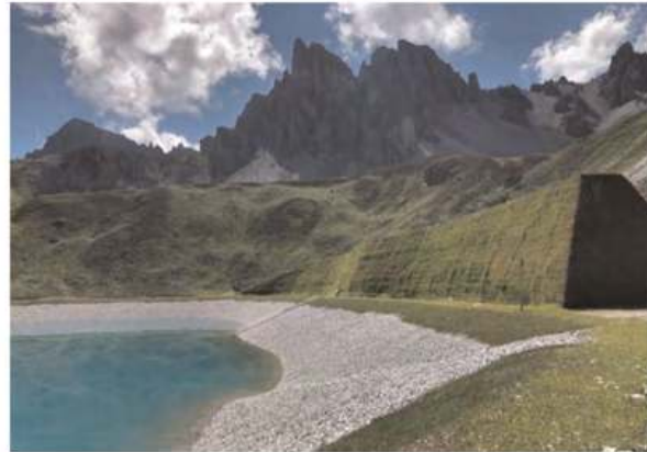
Figure 4. Avalanche protection dam Axamer Lizum after completion.
