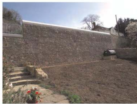
Figure 3. Finished wall with masonry reattached.
