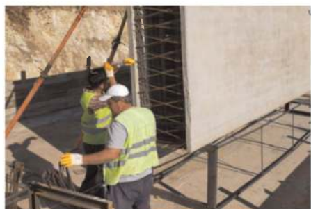
Figure 4c. Installation of horizontal continuity reinforcements.
