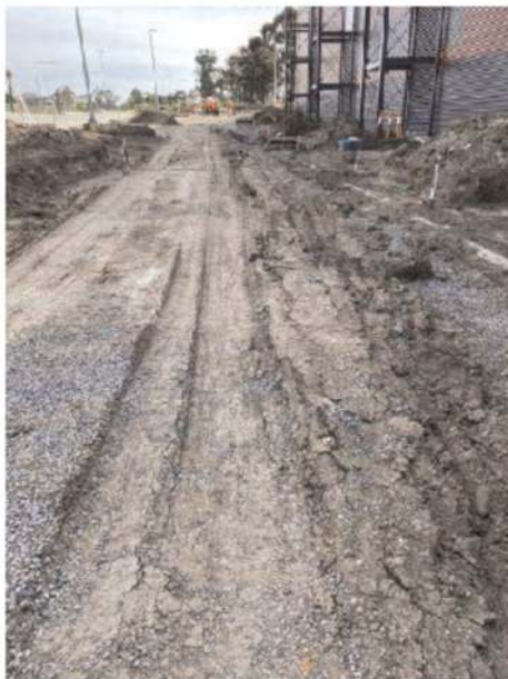
Figure 3. Installing crushed rock capping layer over geogrid.
