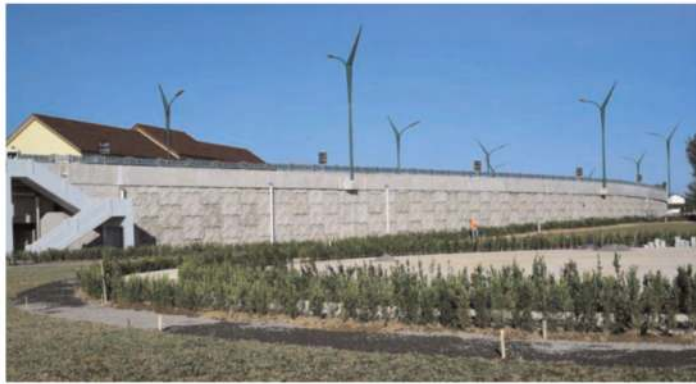
Figure 1. Kretek II Flyover's, Yogyakarta, Indonesia.
