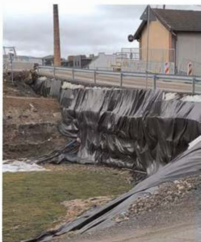
Figure 8. Bypass temporary construction – facing.
