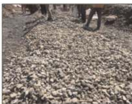
Figure 15. Laying ballast over the blanket layer.
