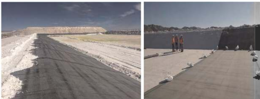
Figures 4 and 5. Lithium salt ponds in the extreme Atacama Desert of Chile. Note the thermal stability of the BGM with no wrinkles.
