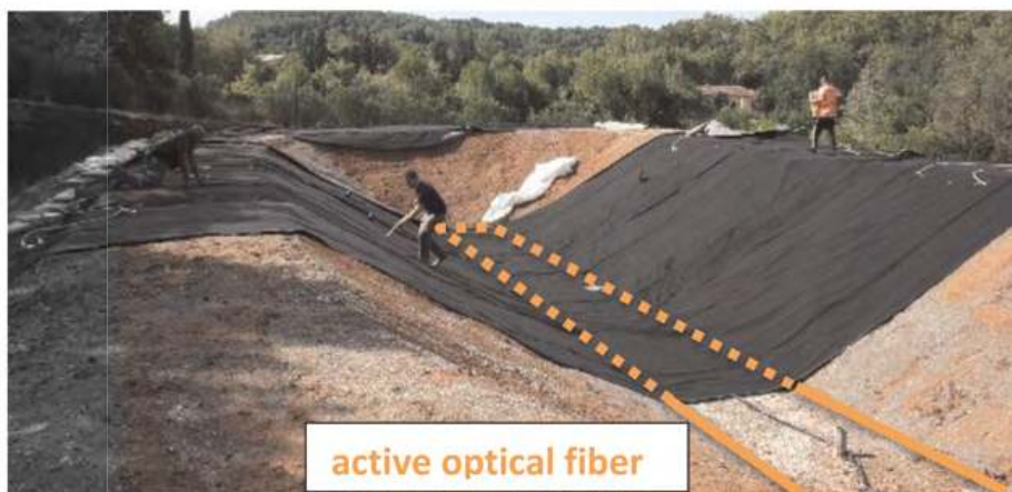
Figure 6. Localization of the active optical fiber.
