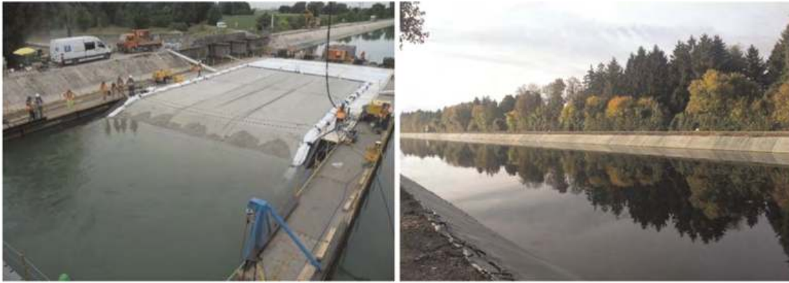
Figure 5. Canal sealing: during installation from pontoon (left); after installation (right).
