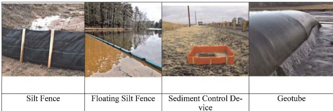
Figure 2. Examples of vertical surface erosion control products.
