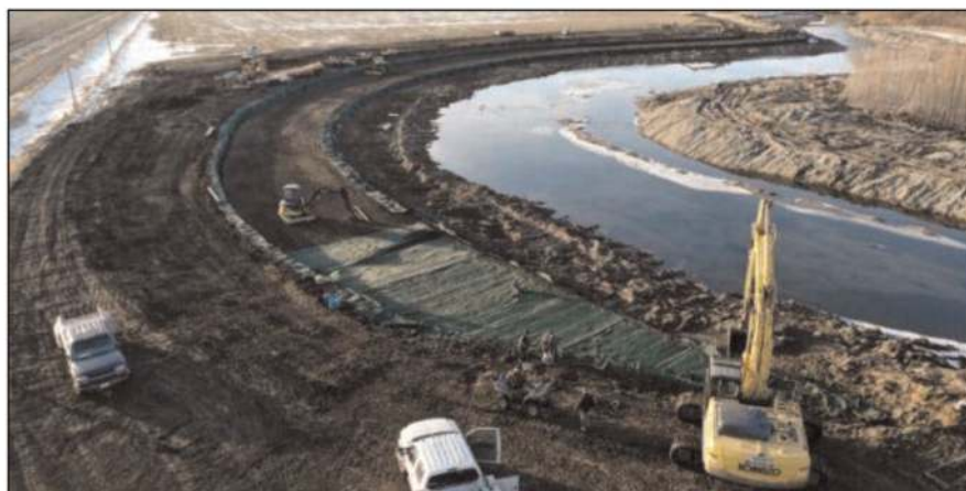
Figure 7. Installation of SCOURLOK and ARMORMAX, January 2021.
