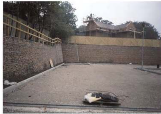
Figure 6. Gabion stone faced wall nailed on left boundary full RSS on adjacent face 1998 (Comtec UK Ltd).
