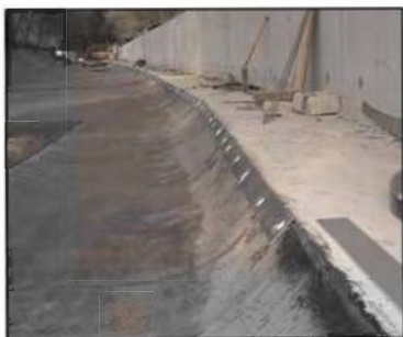
Figure 4. Canal in UK along deep slope.
