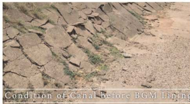
Figure 2. Original condition of canal stretch.
