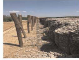
Figure 6. Geomattress filled with a stone material.
