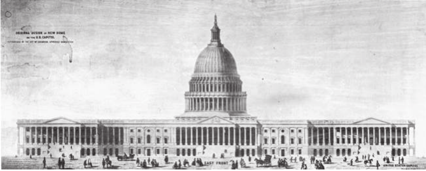
FIG. 7. “Original Design of New Dome on the U.S. Capitol,” by Thomas U. Walter, 1854. This period photograph of the lost seven-foot-long drawing of the architect’s proposed new cast-iron dome attracted much attention when it hung in Walter’s office. ( Architect of the Capitol )
